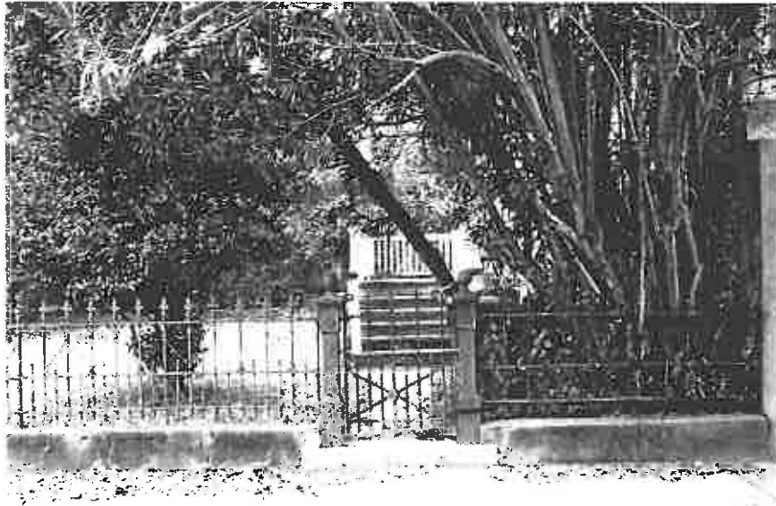
Entry on Smith Street, cast-iron posts and wrought iron gate and fence with masonry coping wall
