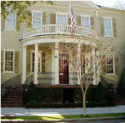
Josiah Smith House at 7 Meeting Street, circa 1785. The house has a hipped roof and cupola. The walls are insulated with brick between the framing timbers, with wood siding.
