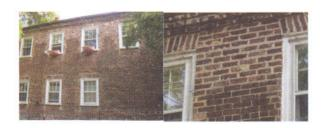
**25 Bull Street** shows evidence of repairs. Clearly visible is the difference between the pre-earthquake building and the repaired structure.
