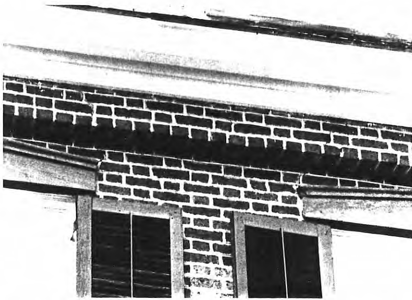
Illustration 6. The appearance of regularity in this example was produced by thin white lines painted onto the surface of flush tooled mortar joints. The mortar was originally the same color as the bricks.
