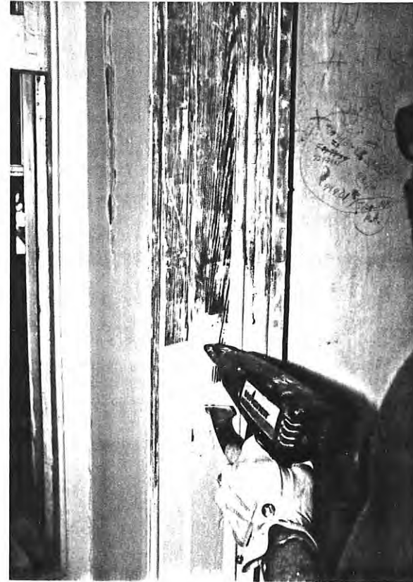
Illustration 33. Less destructive means of paint preparation are available. In areas which must be stripped heat guns can be used. This technique is most effective on molded elements that would be damaged by more aggressive methods.
