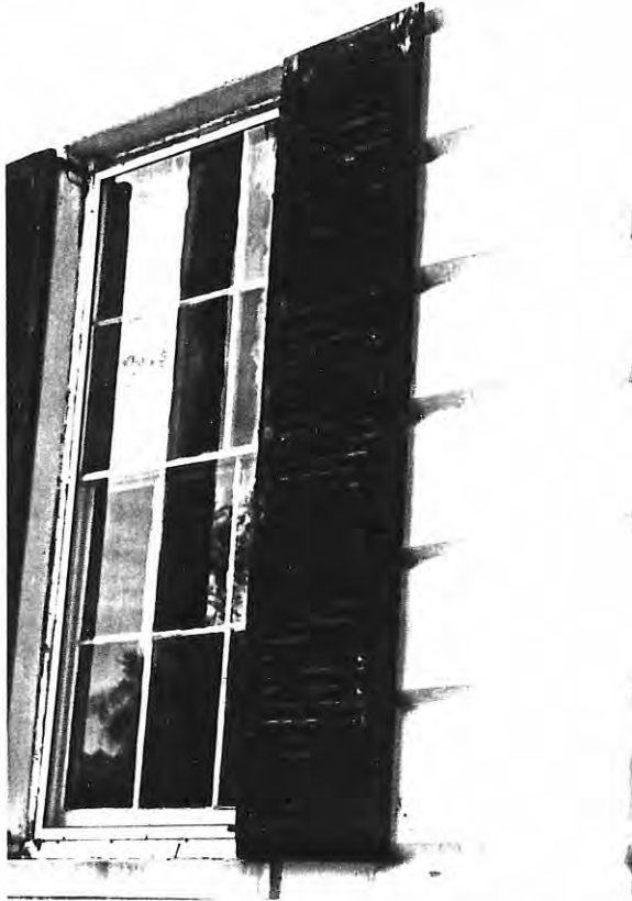
Illustration 32. Wood elements such as doors, sash, shutters and blinds should never be "dipped" in caustic baths. The most common bath solution is lye. This material is quite destructive to the wood fibers and is nearly impossible to remove or "neutralize". These blinds were dipped to remove the accumulated paint. The absorption of the caustic material into the wood is continuing to strip the paint from the surfaces.
