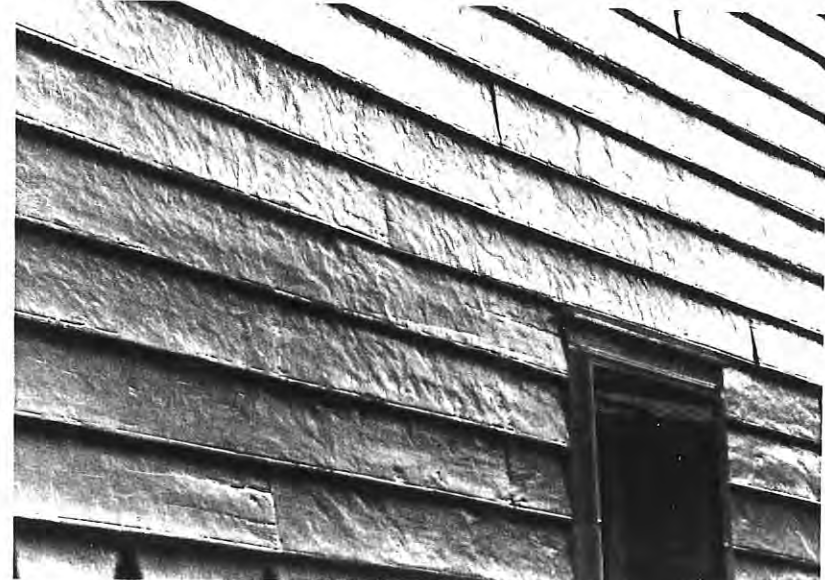
Illustrations 28 and 29. The fine moldings of this entry have been damaged by the disc sander. The cyma recta and cavetto profiles of the smaller moldings have been removed, leaving in their place a rounded, course line. The scalloped texture of the clapboards is typical of the damage produced by the rotary sanders on flat surfaces.
