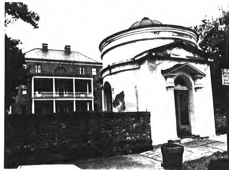
Illustration 19. The gate house at the Manigault House demonstrates the durability of original lime stuccoes and lime repair stuccoes.
