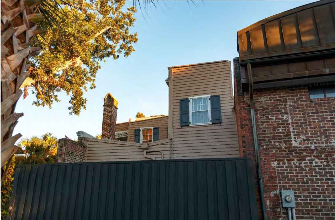
Figure 23 Rear of house showing original piazza, small rear room and the two-story addition to accommodate extended family that moved in the 1920s or 1930s.
