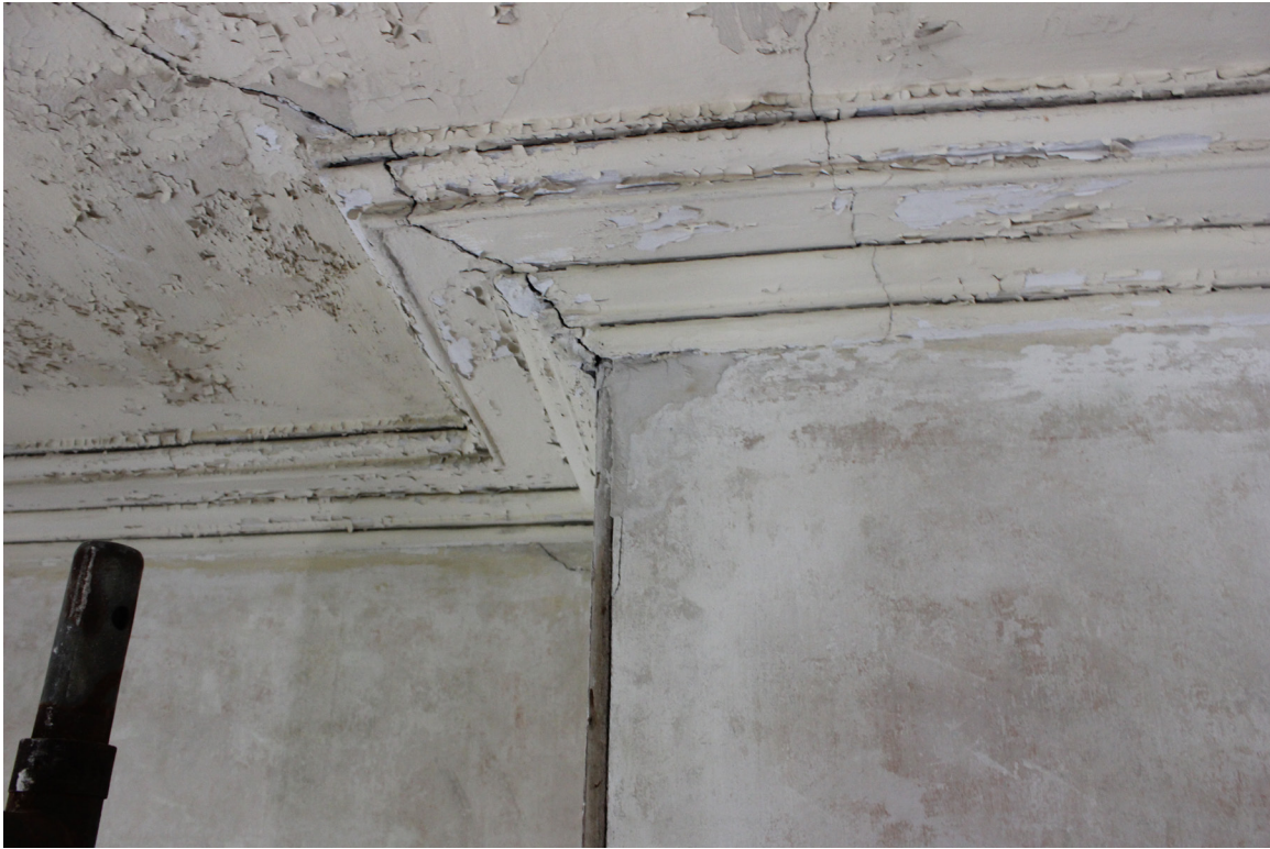
Figure 13: Southeast chamber, cornice: Rolling scaffolding provided access to plaster within the room, ensuring that all surfaces were physically inspected.
