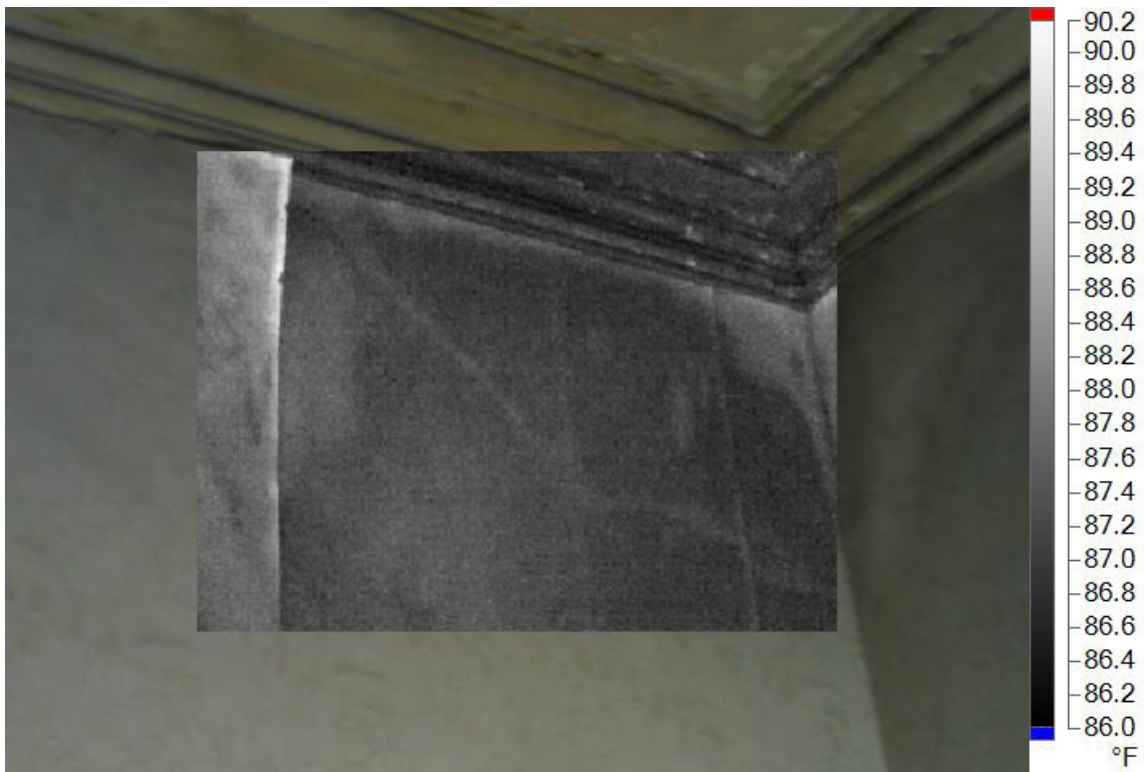
Figure 23: Southeast chamber, west wall: The cracking within the plaster obscured by wallpaper was visible through infrared analysis.
