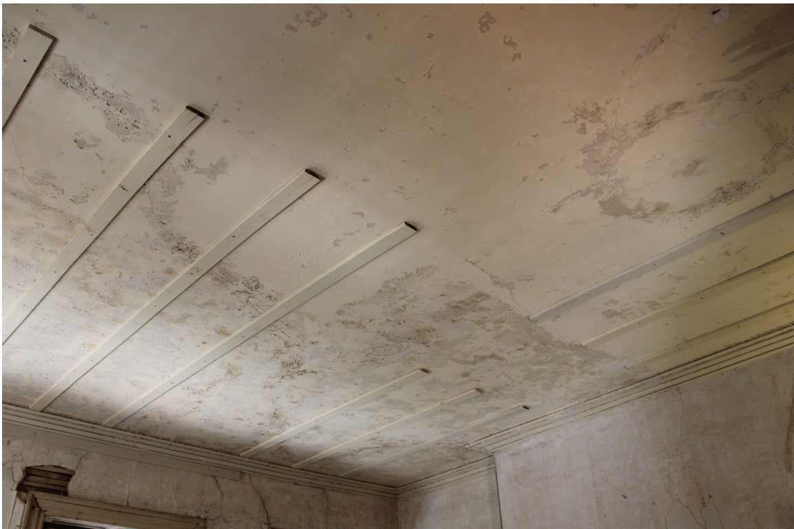
Figure 8: Southwest chamber, facing northwest: Stabilization installed in 2014. The battens in this room only partially span the ceiling.
