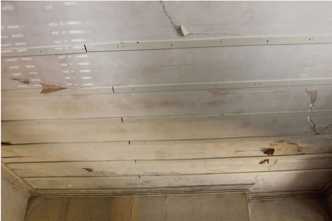
Figure 7: Southeast chamber, facing north: Stabilization installed in 2014 over existing cracks. The battens in this room span the full width of the ceiling.
