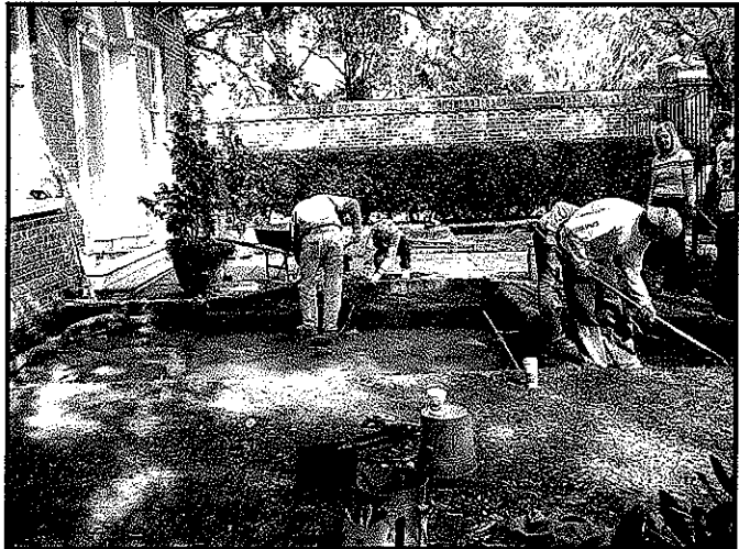
2003: Expanding the N200 block, facing north
