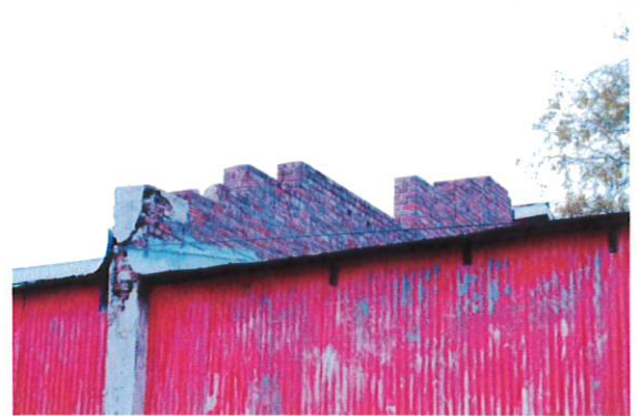
Brick firewall separating the building's east wing from its northern neighbor (5 Pinckney Street)
