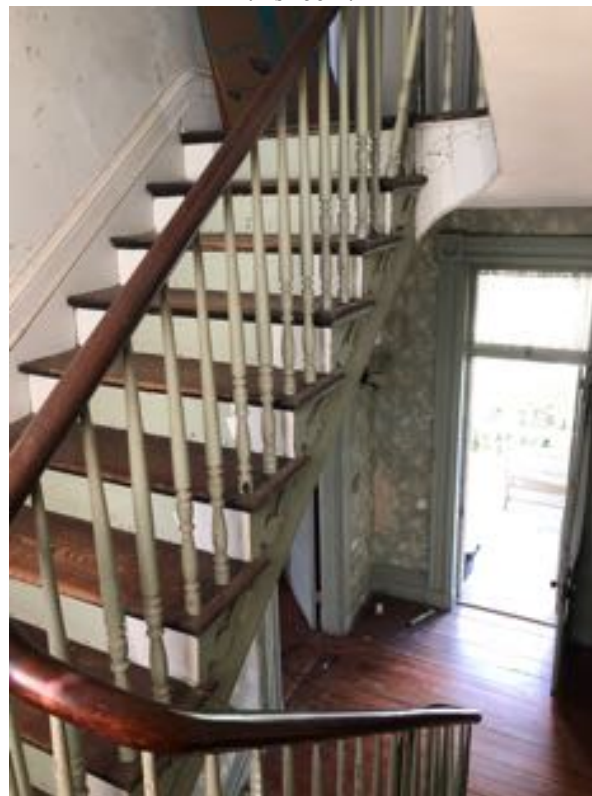
Simple but elegant Greek Revival style balustrades along the stairs. Note the thick Greek Revival door casing with corner blocks.
