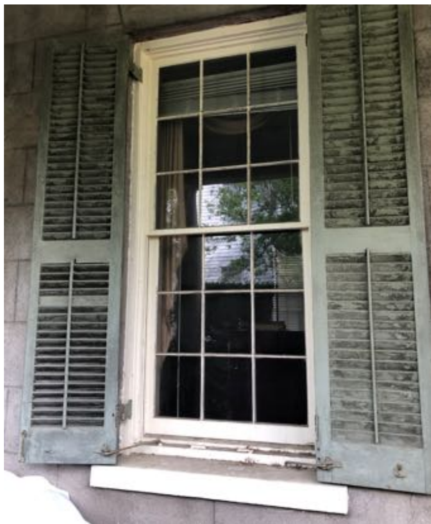
A traditional nine over nine wood sash window with historic louvered shutters.
