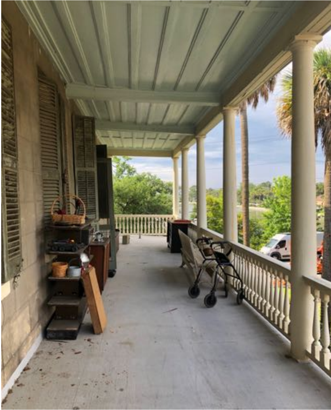
A view toward Colonial Lake from the second story piazza. The Tuscan columns and balustrades are likely original. Note the heavily scored stucco on the exterior wall, to mock a stone block finish. The piazza ceilings have early wood paneling.
