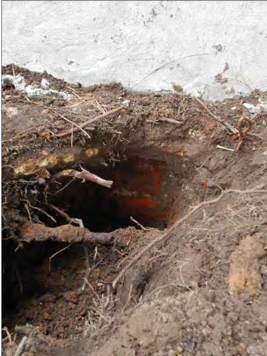
Figure 14. View of the exploratory excavation and the exposed brick wall at the two-story house.
