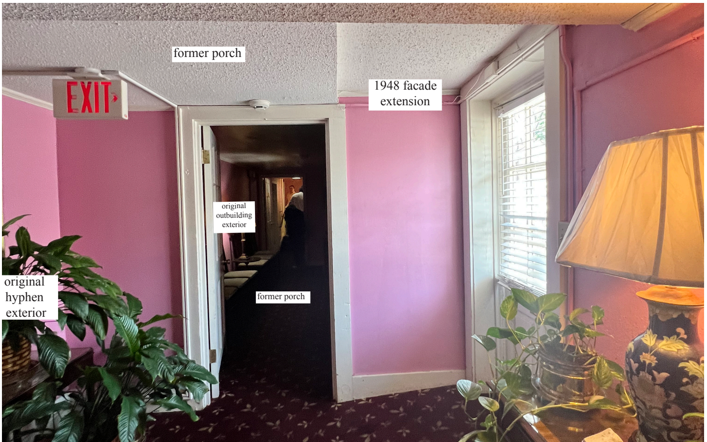
Figure 5: Looking east from within the hyphen's former porch towards the outbuilding; the soffit delineates the footprint of the former porch from the 1948 facade extension.
