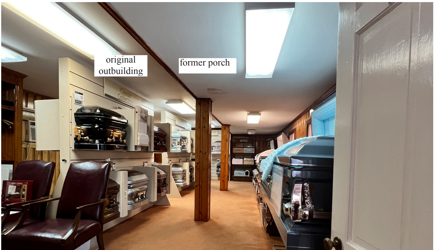
Figure 8: Directly upstairs from Figure 7, looking east; the original outbuilding's footprint is delineated by the columns and trim
