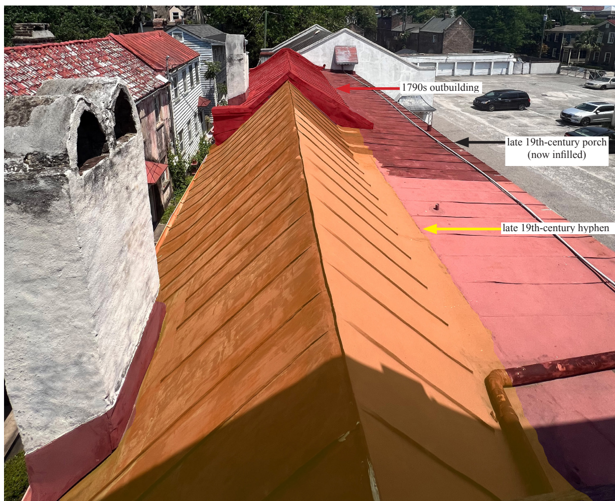
Figure 4: Roof of outbuilding and hyphen (looking east); original outbuilding delineated by surviving gable ends
