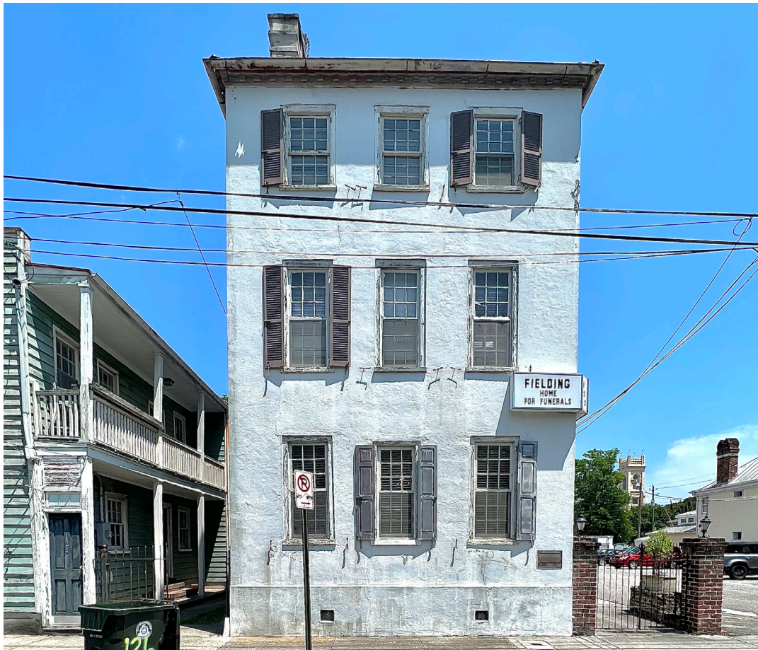
Figure 1: Main (west) elevation of No. 122 Logan Street, showing original water table, cornice and surviving eighteenth-century windows at the third story.
