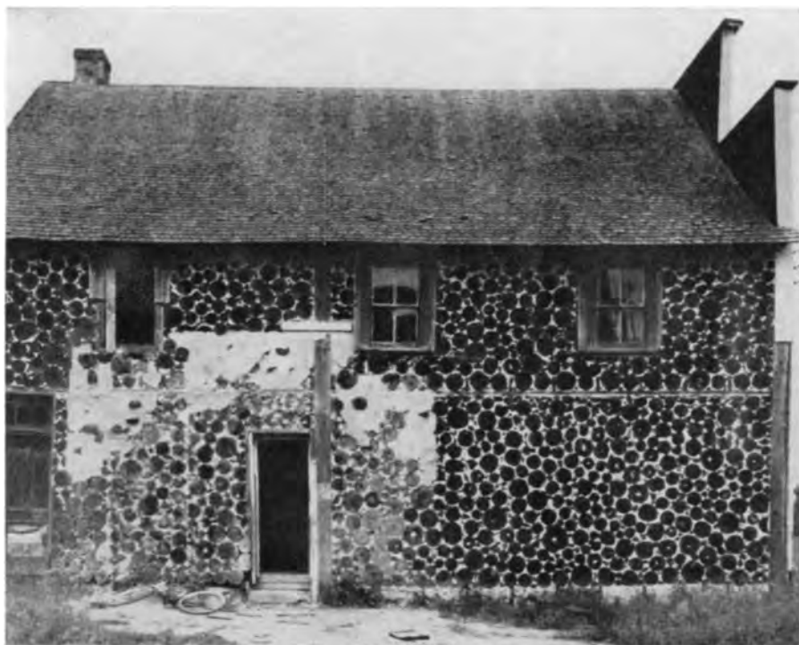
FIG. 30—Stovewood construction, Wisconsin. (Photograph courtesy R. W. E. Perrin.)
