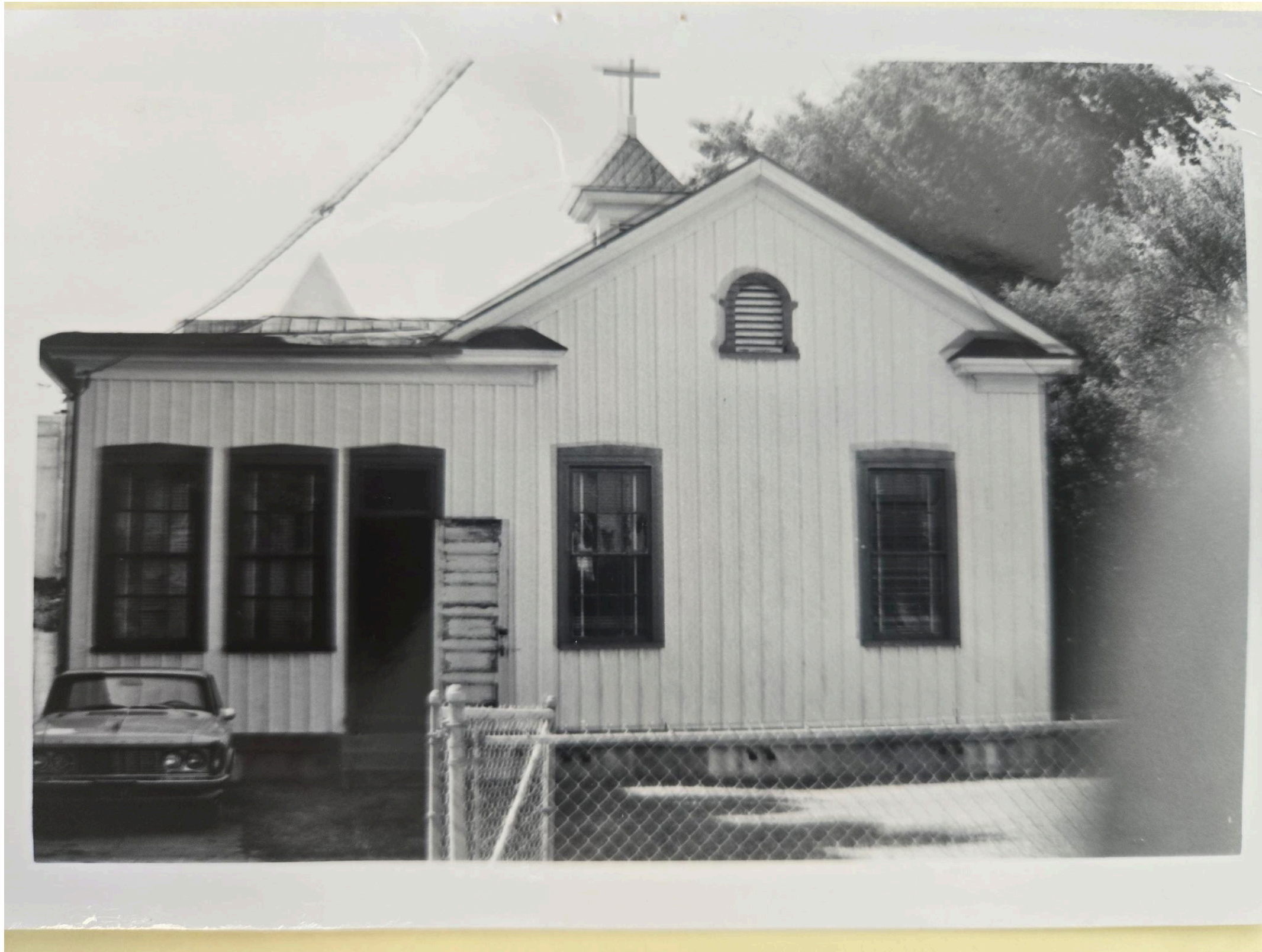
Figure 17. 1968, South Elevation, Appraisal Photographs, Roman Catholic Diocese of Charleston.
