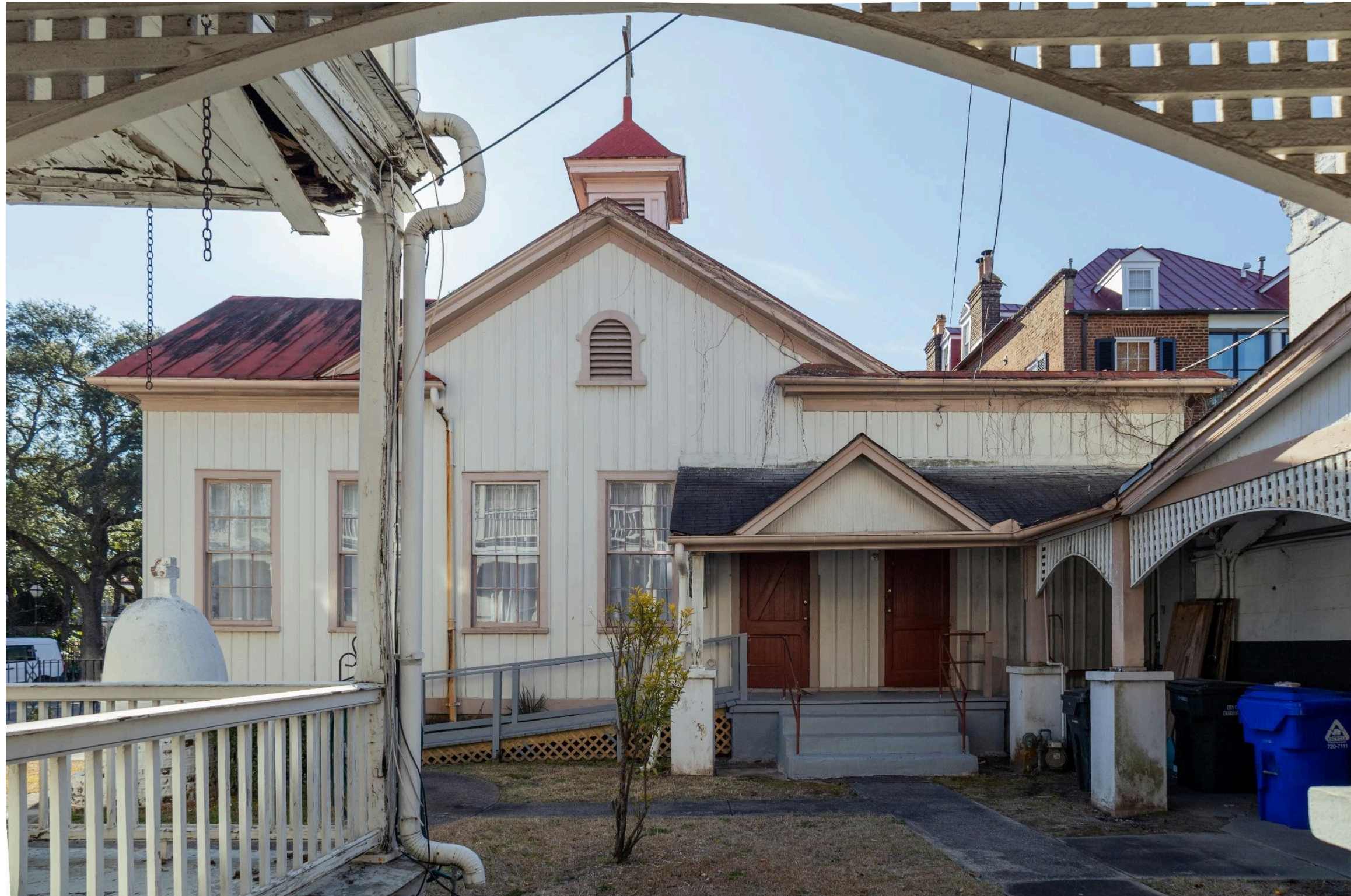
Figure 12. East Elevation from porch of Parishioners Hall.
