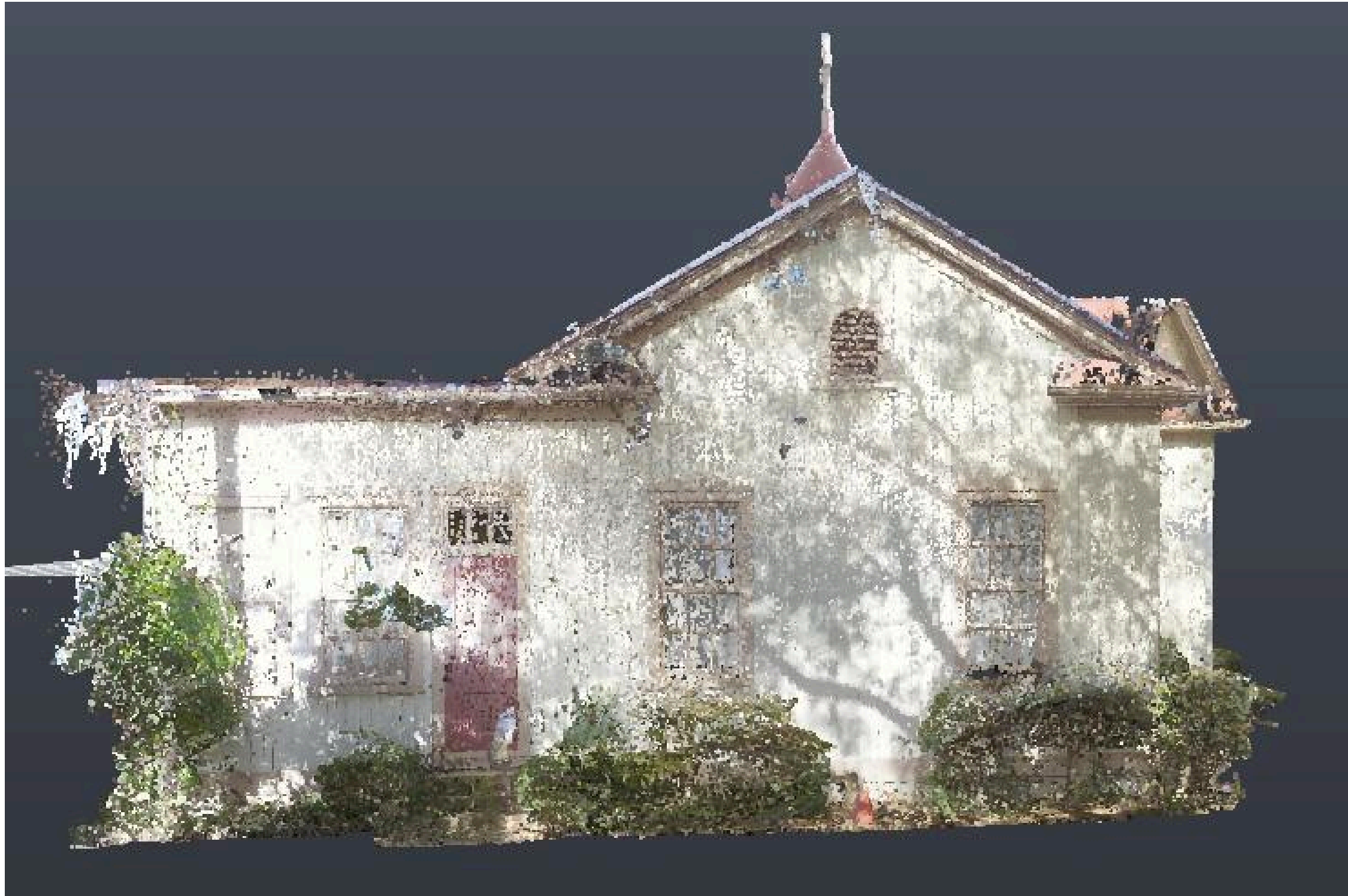
St John's Ed Building West Exterior Facade
