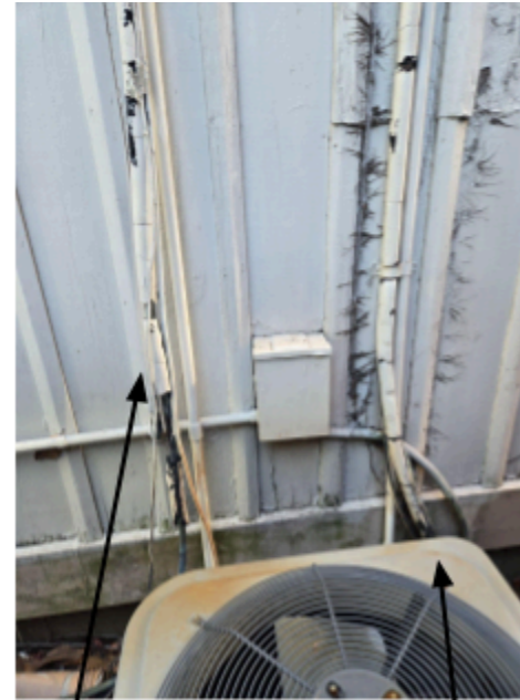
Chipping electrical covers.
