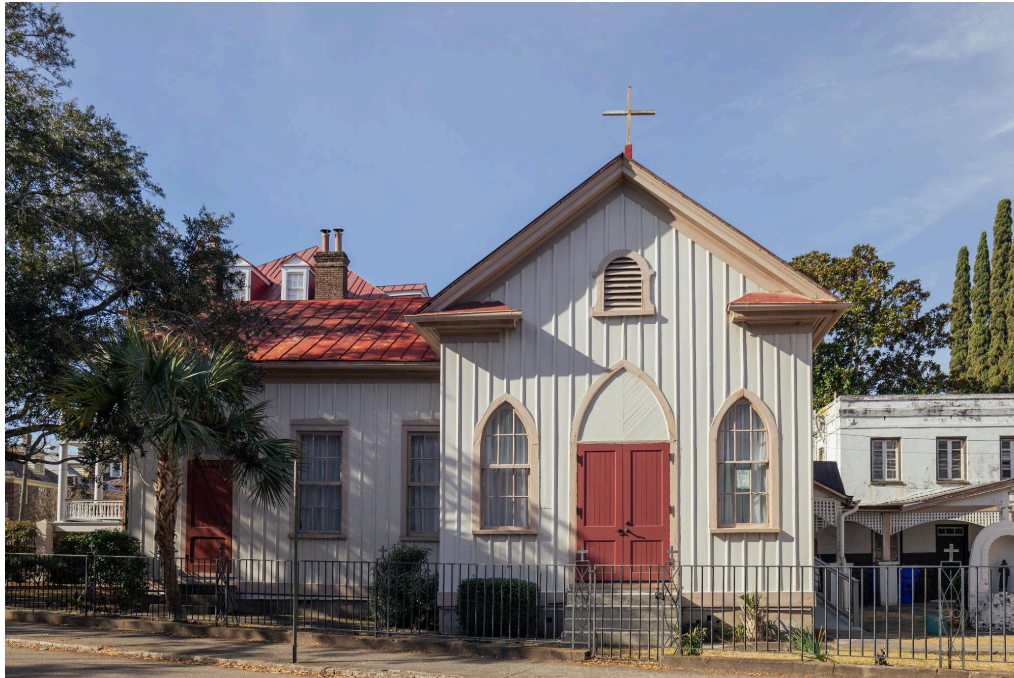
Figure 1. East Elevation, Anson St.
