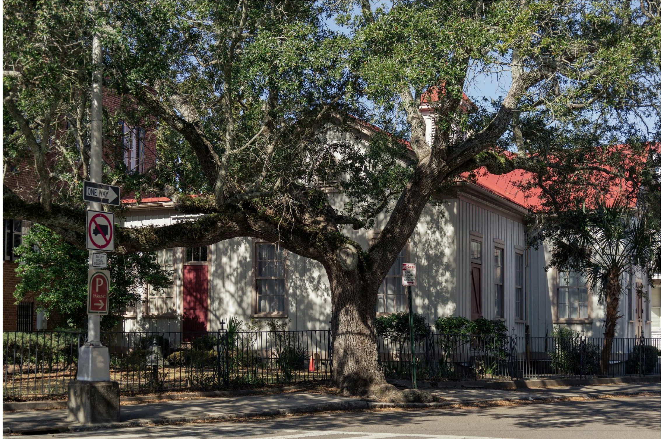
Figure 5. South East Elevation from the corner of Anson and George Streets.
