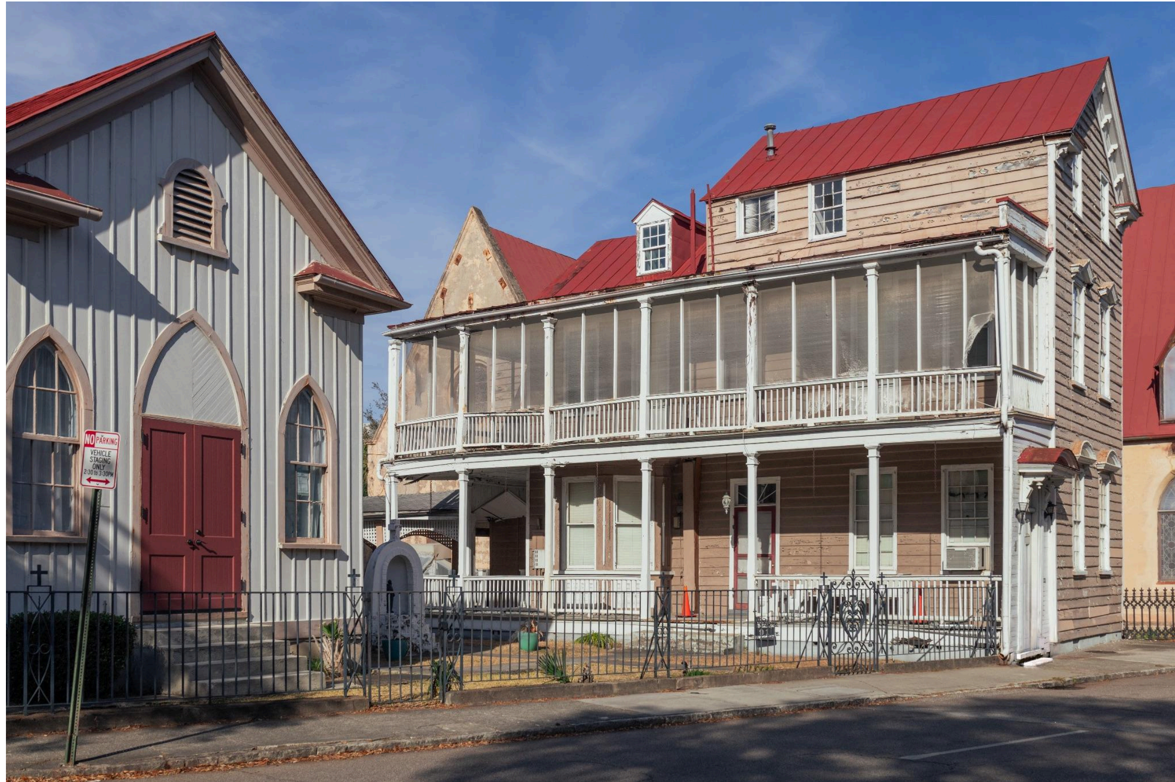
Figure 15. East elevation of Education Building and South Elevation of Parishioners Hall.
