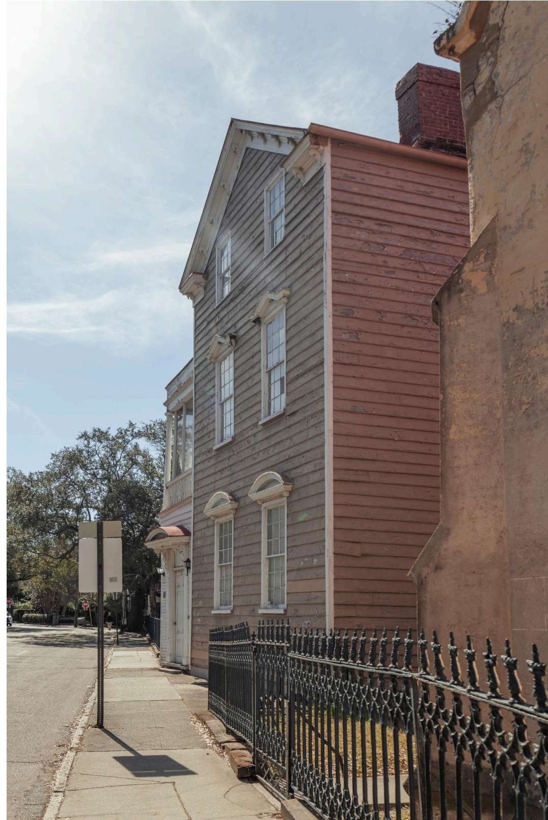
Figure 17. North East elevation of single house.
