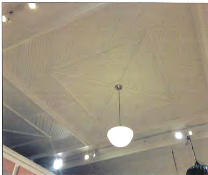
Detail of diagonal beadboard ceilings inside first floor. The ceilings were rediscovered and restored during the 2003 restoration of the building.
