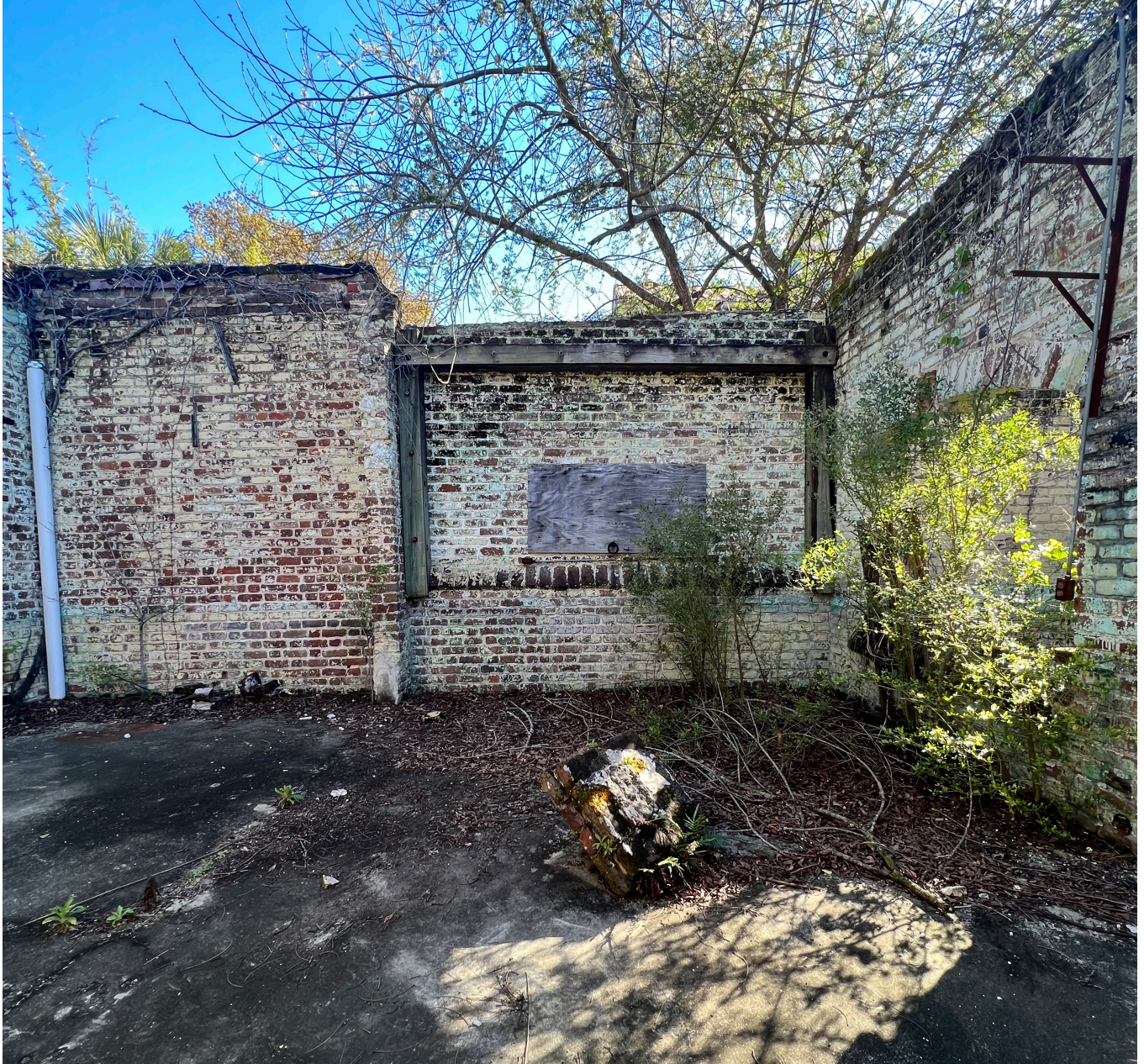
View looking east within middle 1938 service bay, showing 1930s infill of half-height boundary wall
