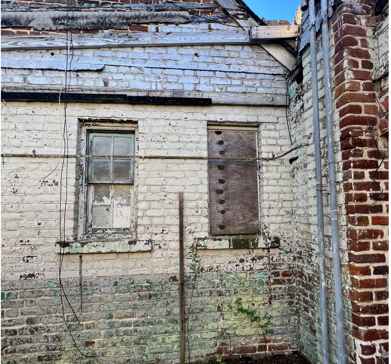
Detail of north elevation of main office, showing original 4/4 wooden sash
