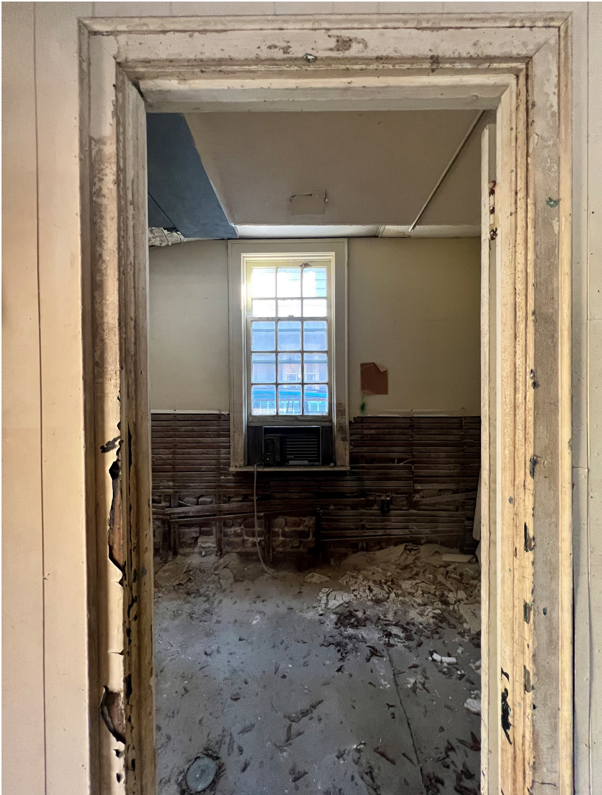
View looking east within original office at first floor, showing original 9/9 wooden sash and lath
