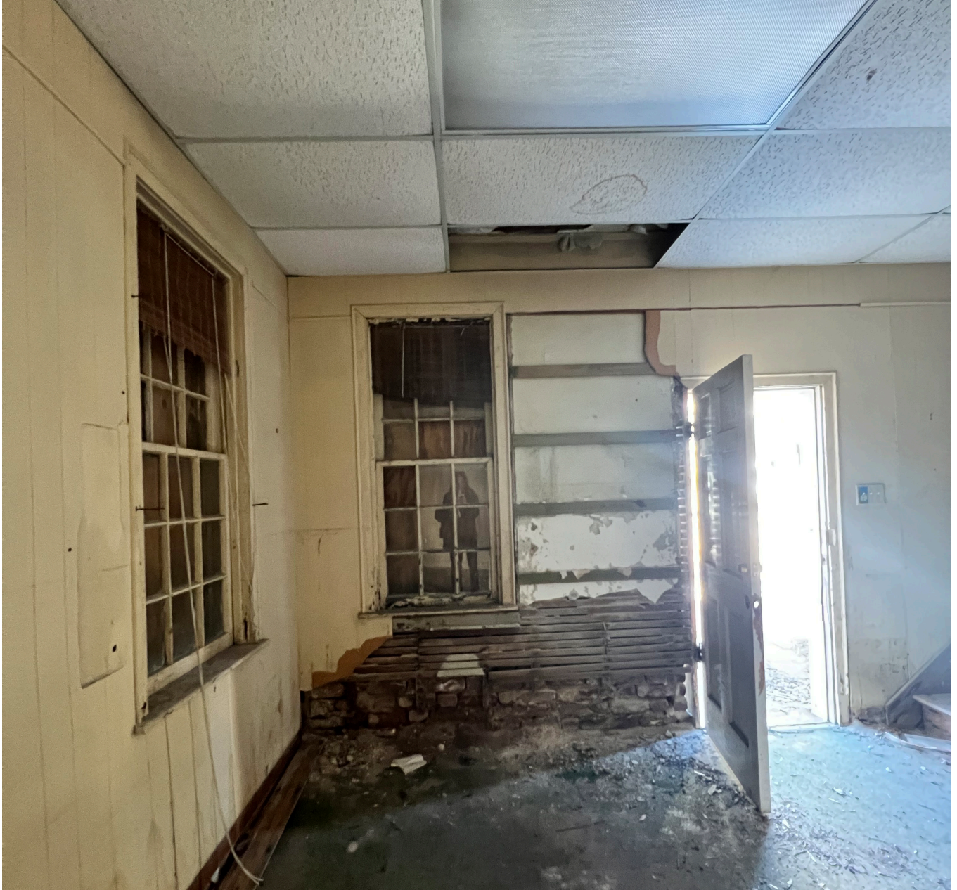
View looking west at first floor, showing original window sash, lath and evidence of plaster
