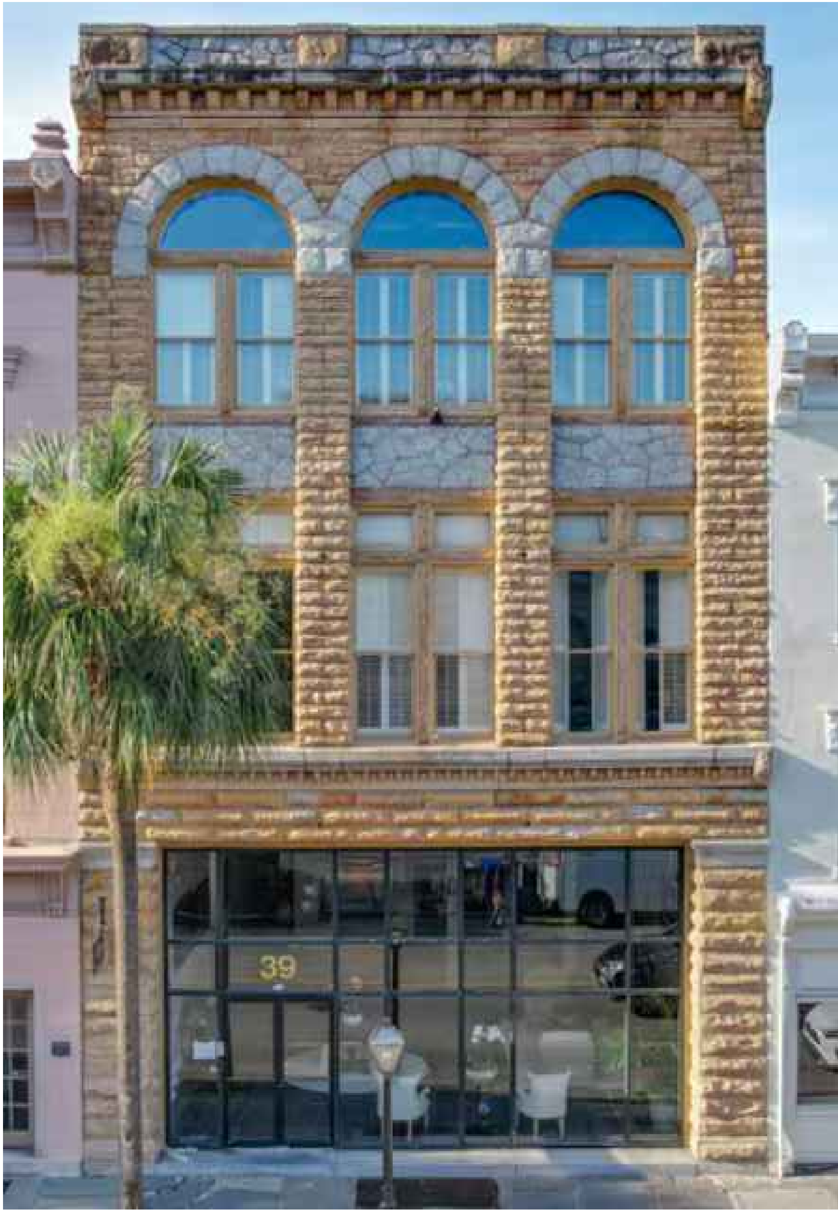
01 A-200 PHOTOGRAPH OF FACADE 2025 NTS
