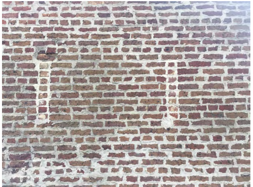
(Above) Northern wall showing English Garden Wall bond and filled in decorative vents
