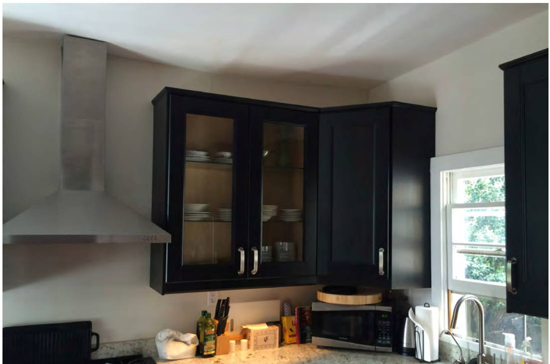
Figure 90. Ceiling Deformation in the Kitchen Addition.
