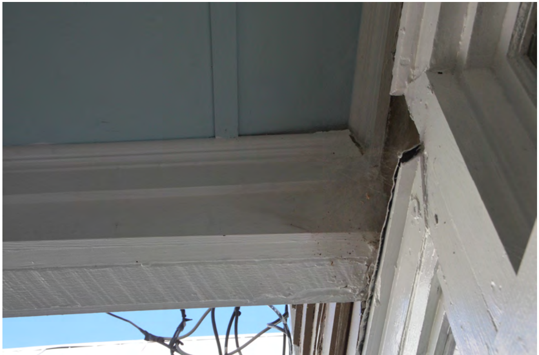
Figure 60. Twisting of the 2nd Floor Framing Edge Beam at the Kitchen Addition.
