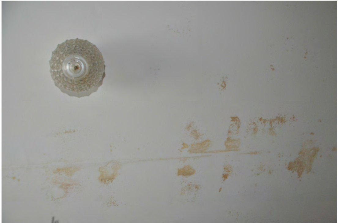
Figure 73. Water Stains on the Ceiling of the Laundry Room.
