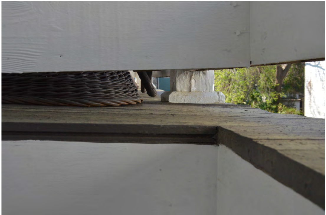
Figure 62. Buckling of the Floor on the 2nd Level of the Piazza.
