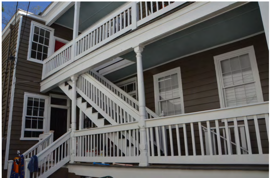
Figure 54. Deformation of the 2nd Floor Framing Edge Beam.
