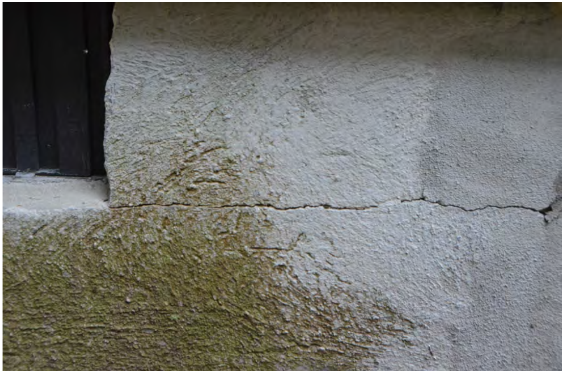
Figure 40. Foundation Cracks.
