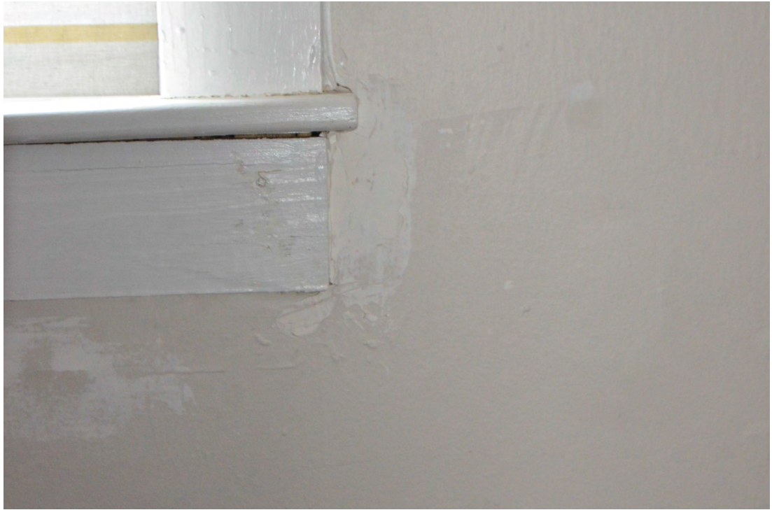
Figure 89. Plaster Failure in the Living Room.
