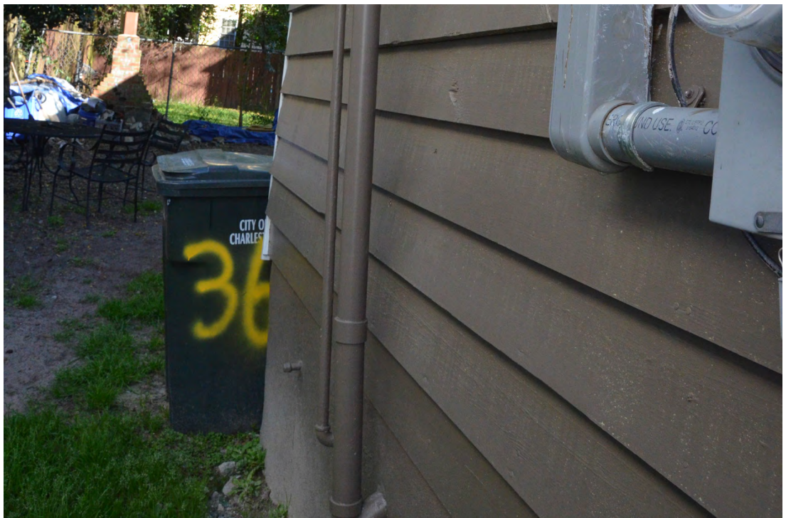
Figure 42. Bowling of the Northwest Corner of the Kitchen Addition.
