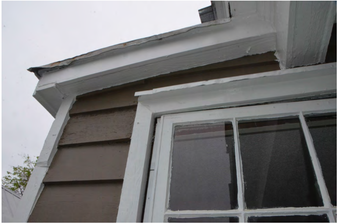
Figure 35. Shifting of Fenestrations on the 2nd Level.
