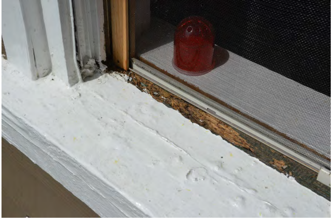
Figure 29. Wood Rot on a Window of the Kitchen Addition.
