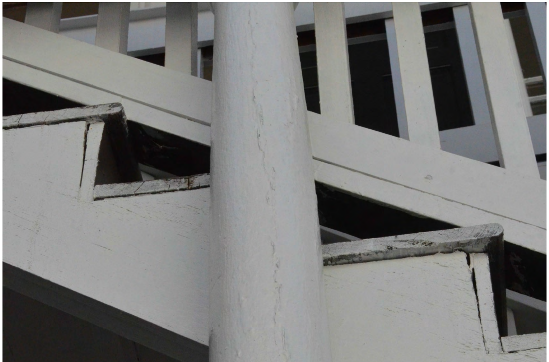
Figure 46. Splitting Columns.
