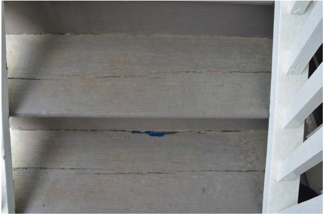
Figure 51. Splitting Wood on the Exterior Piazza Stairs.
