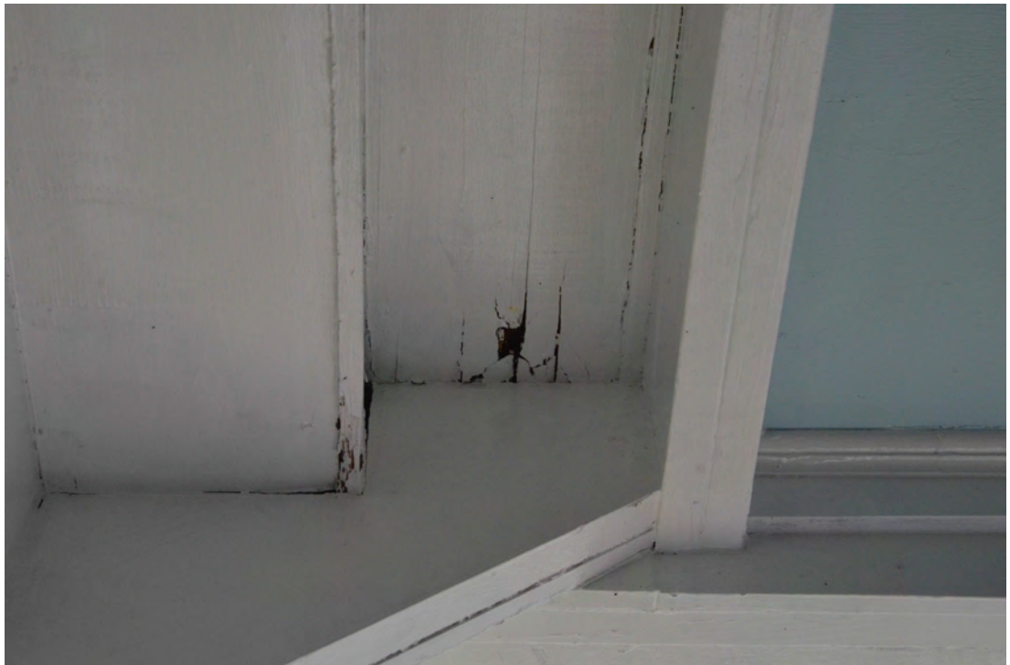
Figure 48. Deteriorated Wood on the Exterior Piazza Stairs.
