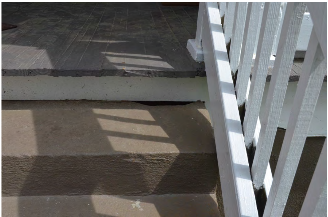
Figure 44. Loss of Material (Concrete) on the Side Stairs.
