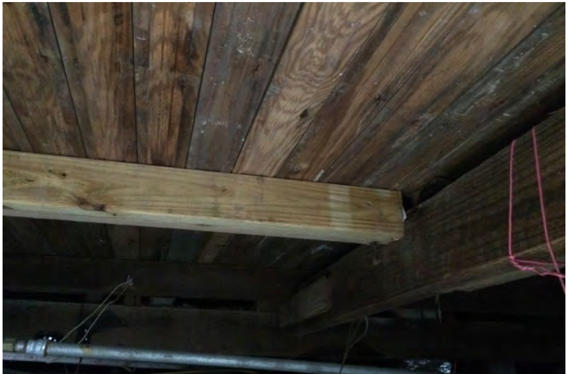
Figure 96. New framing beneath first level of the piazza.
