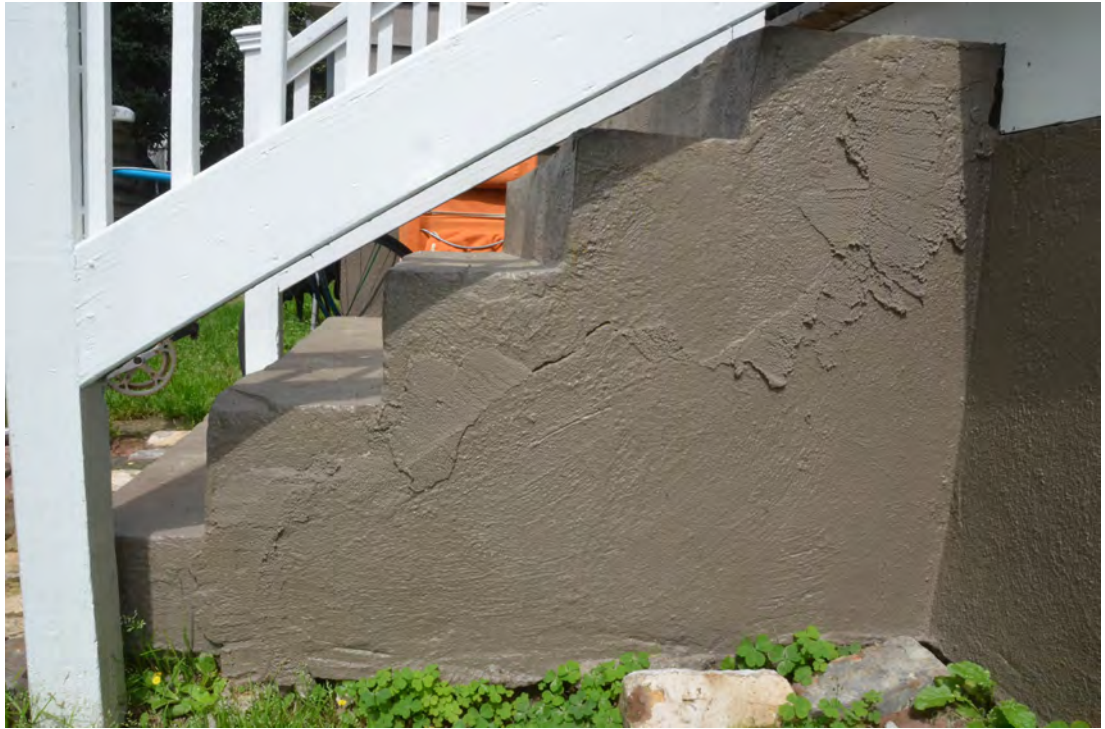
Figure 43. Diagonal Crack in the Side Concrete Stairs.
