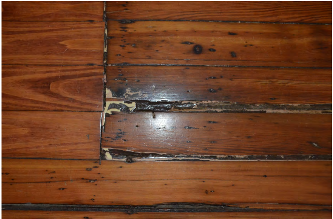
Figure 66. Failed Wood Consolidant Repairs.
