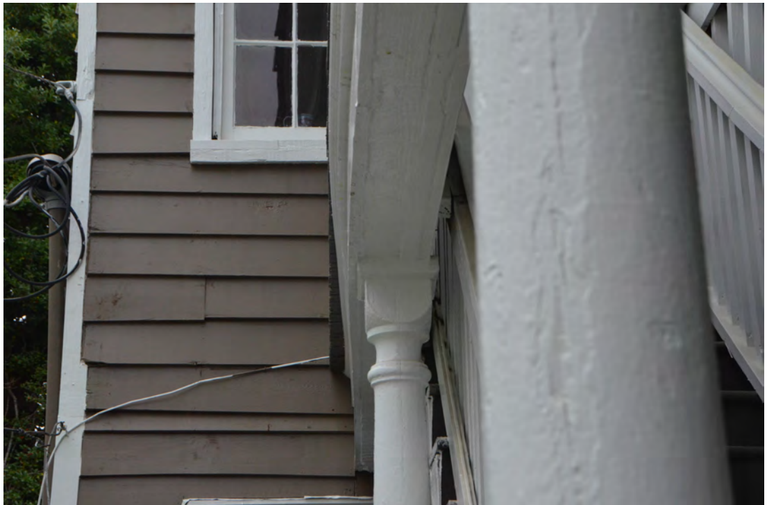
Figure 56. Outward Bowing of the 2nd Floor Framing Edge Beam.
