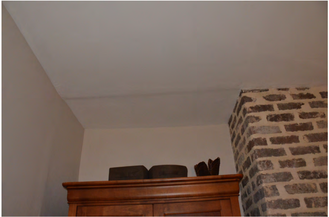
Figure 71. Ghost Marks from a Former Wall.
