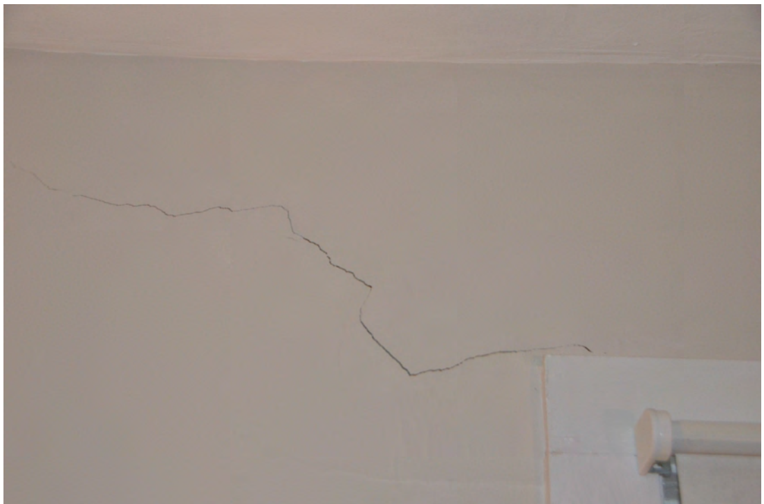
Figure 80. Diagonal Crack in the Plaster at Corner of the Window.
