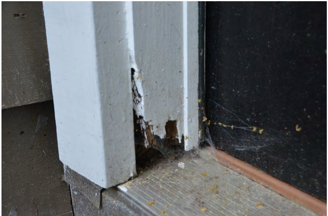
Figure 28. Wood Rot on an Exterior Door Surround.
