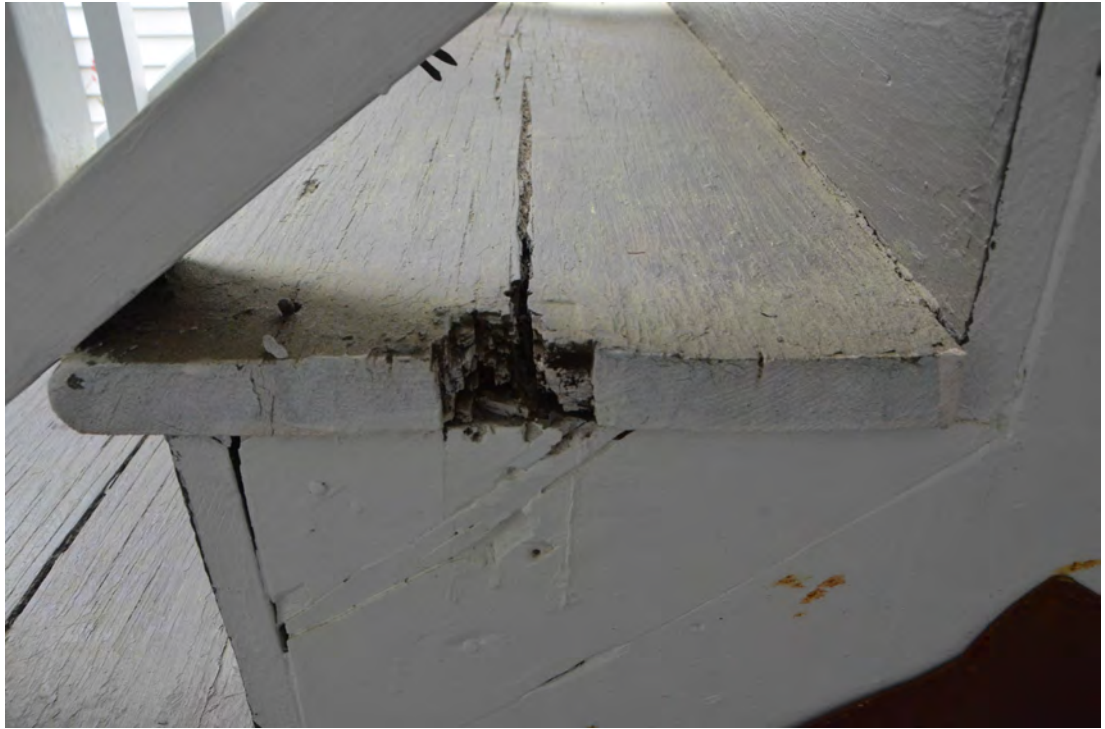
Figure 49. Deteriorated Wood on the Exterior Piazza Stairs.
