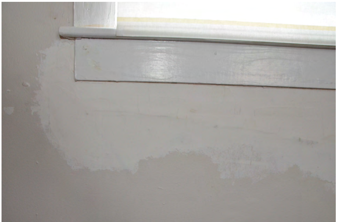
Figure 88. Plaster Failure in the Living Room.
