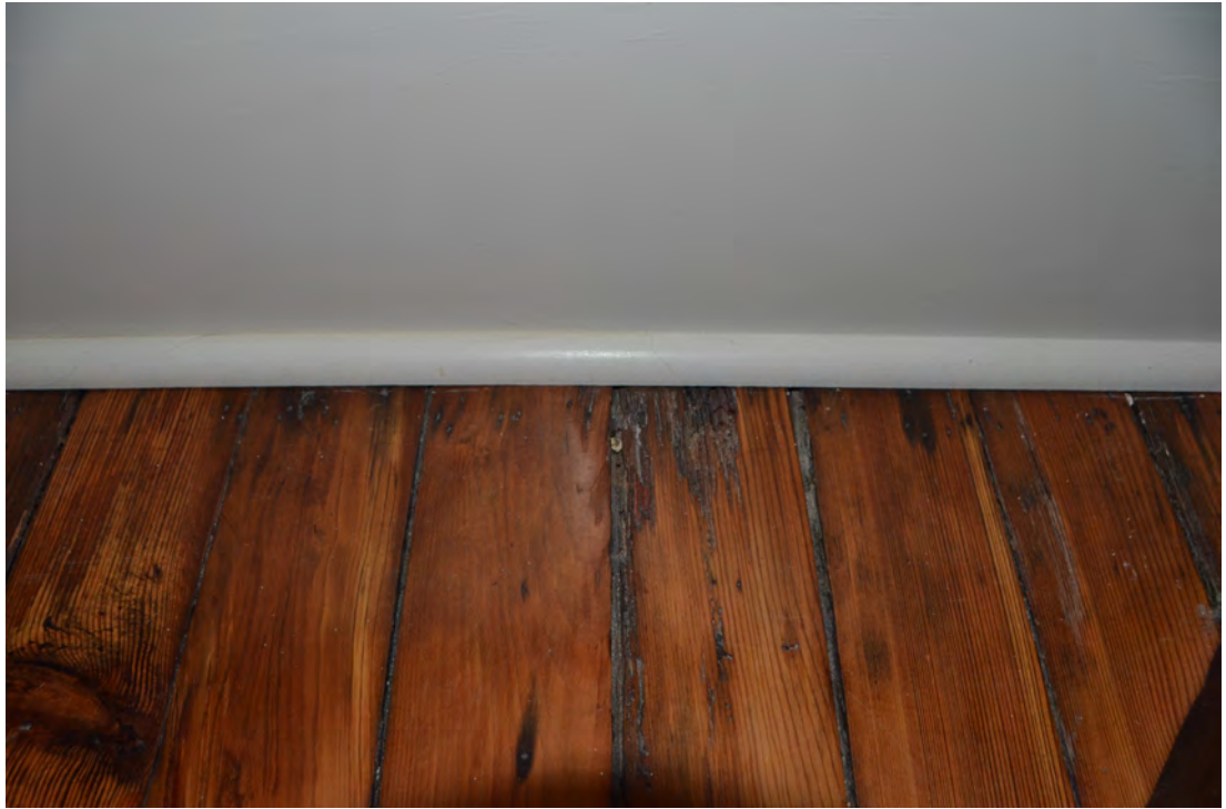
Figure 63. Deterioration of the Wood Flooring.
