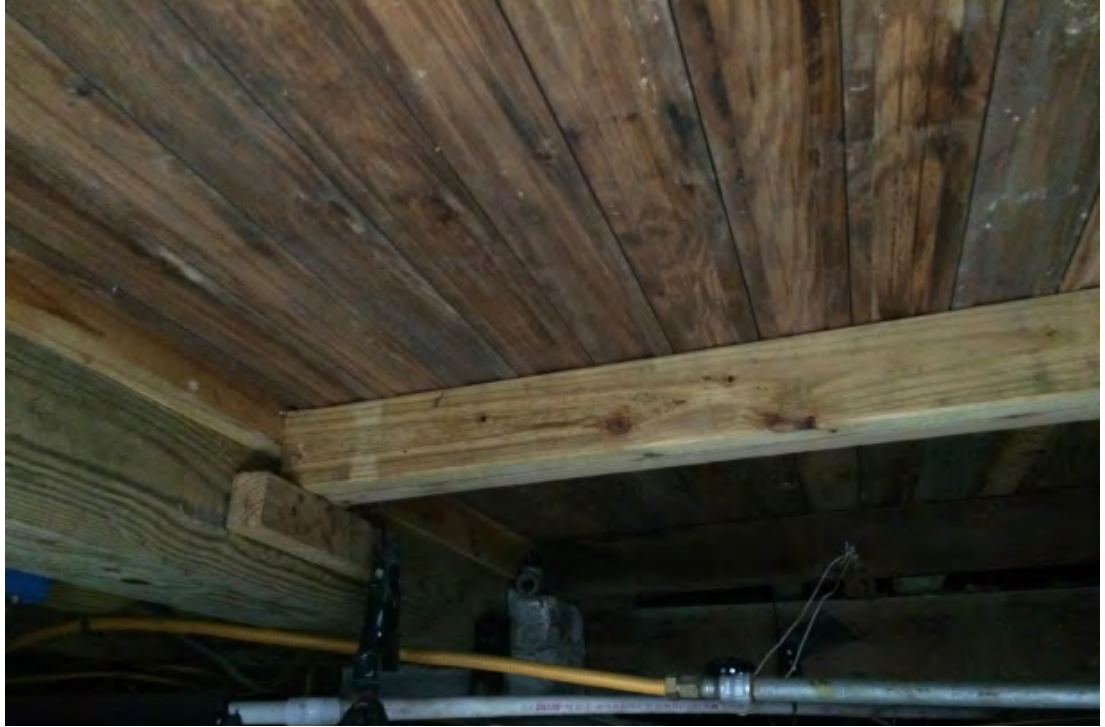
Figure 95. New framing beneath first level of the piazza.
