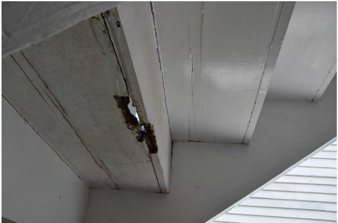
Figure 50. Deteriorated Wood on the Exterior Piazza Stairs.
