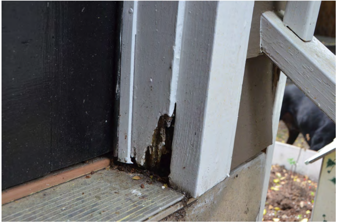
Figure 27. Wood Rot on an Exterior Door Surround.
