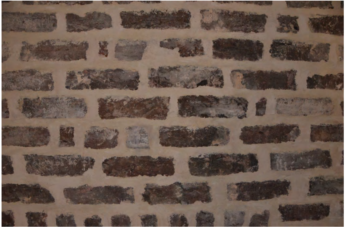
Figure 75. Inappropriate Mortar Repair on the Fireplace.
