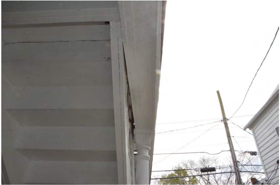
Figure 55. Outward Bowing of the 2nd Floor Framing Edge Beam.
