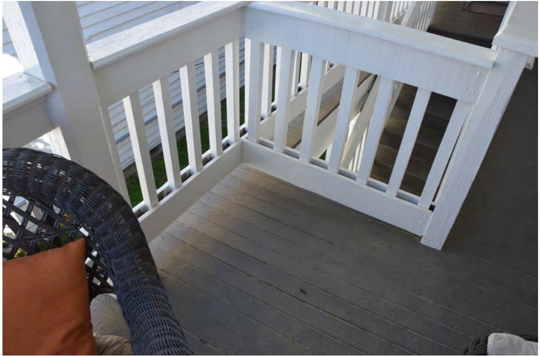
Figure 61. Settlement of the Floor on the 2nd Level of the Piazza.
