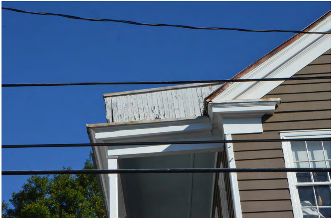
Figure 24. Deteriorated Parapet.
