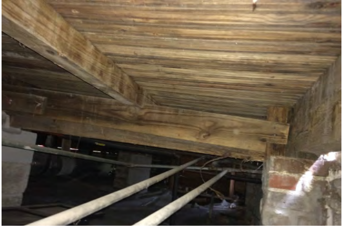
Figure 97. New framing beneath first level of piazza.
