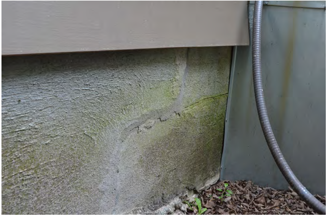
Figure 41. Foundation Cracks.
