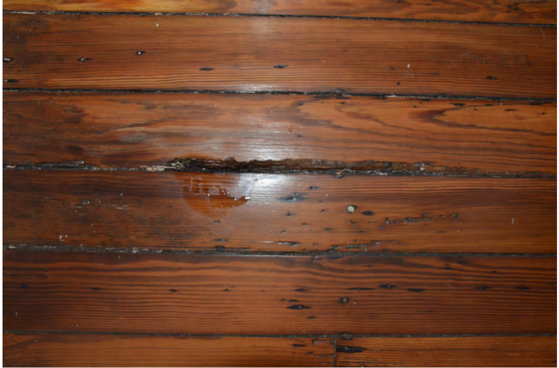
Figure 65. Deterioration of the Wood Flooring.
