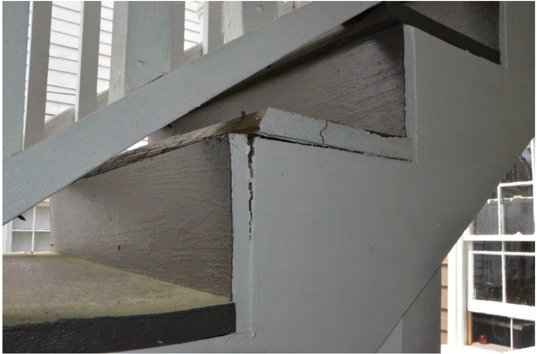
Figure 47. Splitting Wood on the Exterior Piazza Stairs.
