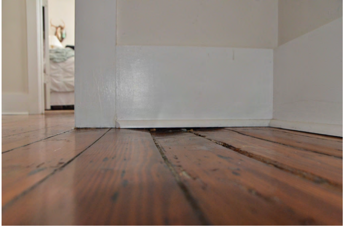
Figure 67. Deformation and Settlement of the Wood Flooring.
