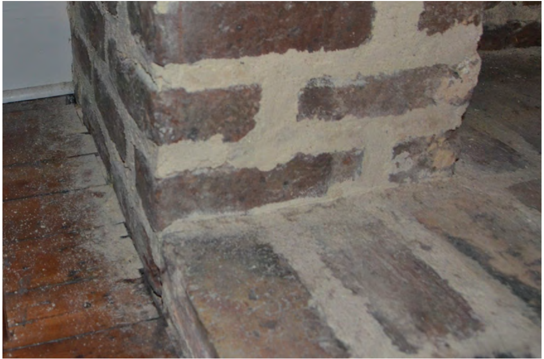
Figure 87. Jagged Flooring at the Fireplace.
