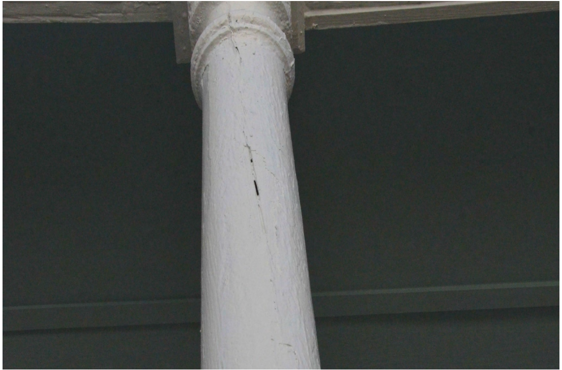
Figure 45. Splitting Columns.
