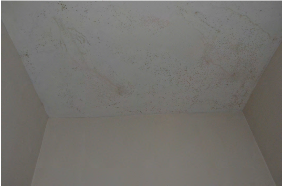
Figure 85. Mold in the Bathroom.
