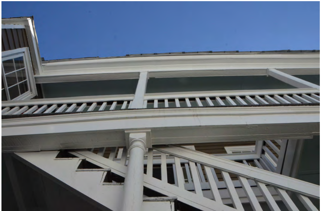
Figure 58. Upward Bowing of the Edge Beam at the North Column.
