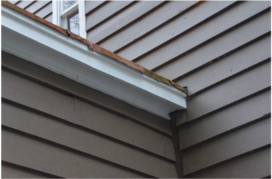
Figure 31. Corroded Roofing Material Over the Hyphen.
