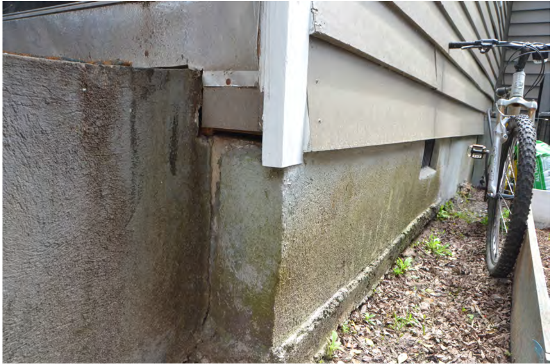
Figure 19. Biogrowth at the Northwest Corner of the Outbuilding.
