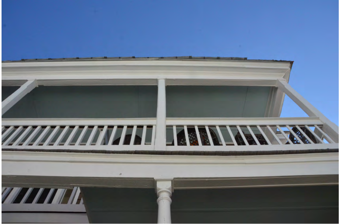
Figure 57. Deflection of the Edge Beam at the South Column.
