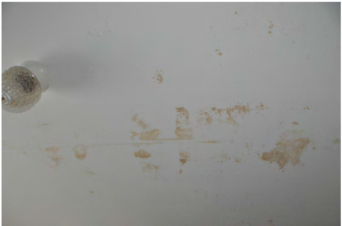
Figure 74. Water Stains on the Ceiling of the Laundry Room.
