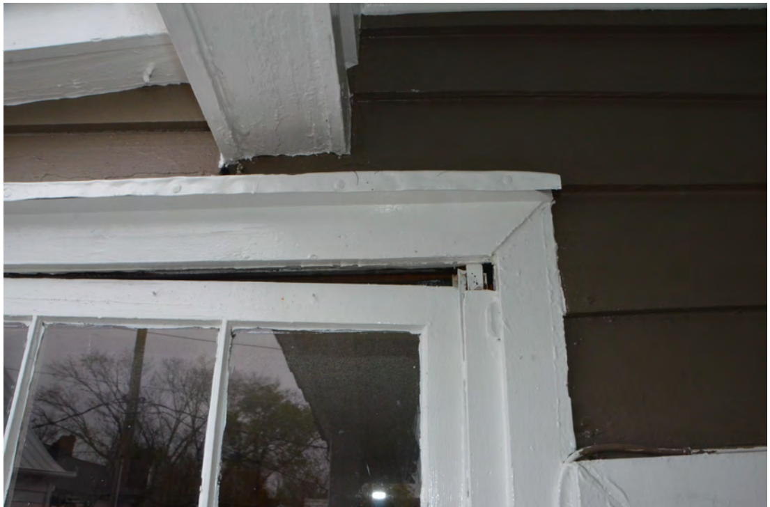
Figure 34. Shifting of Fenestrations on the 2nd Level.
