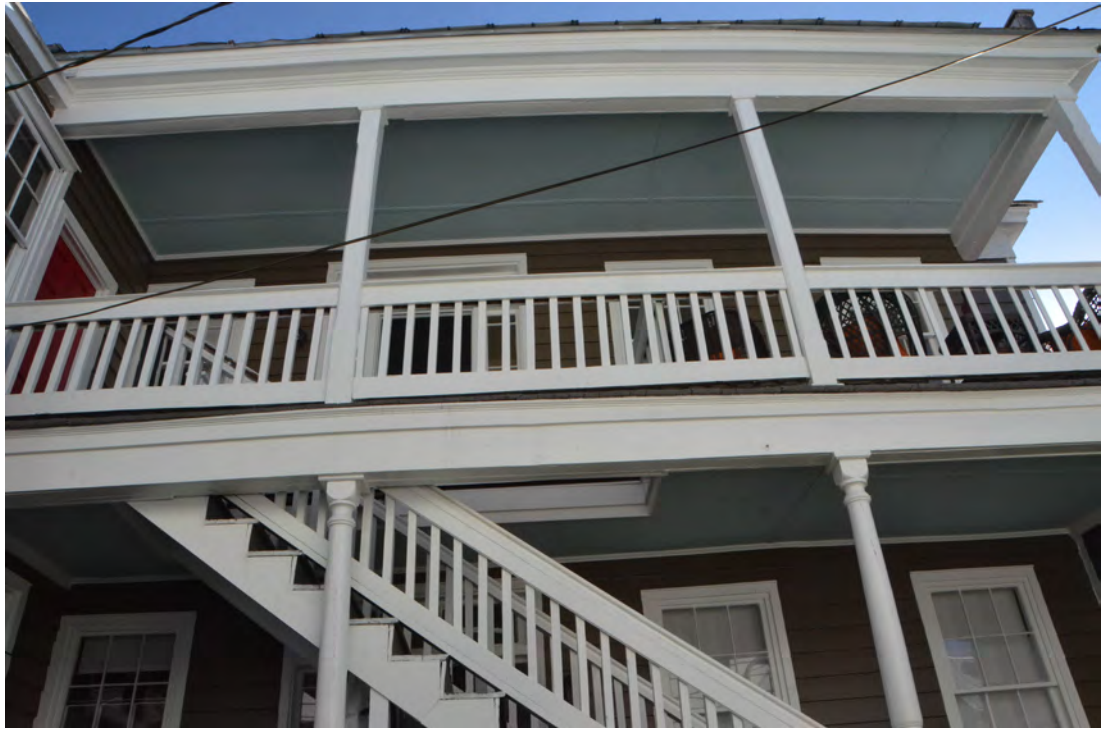
Figure 59. Deformation of the 2nd Floor Framing Edge Beam.
