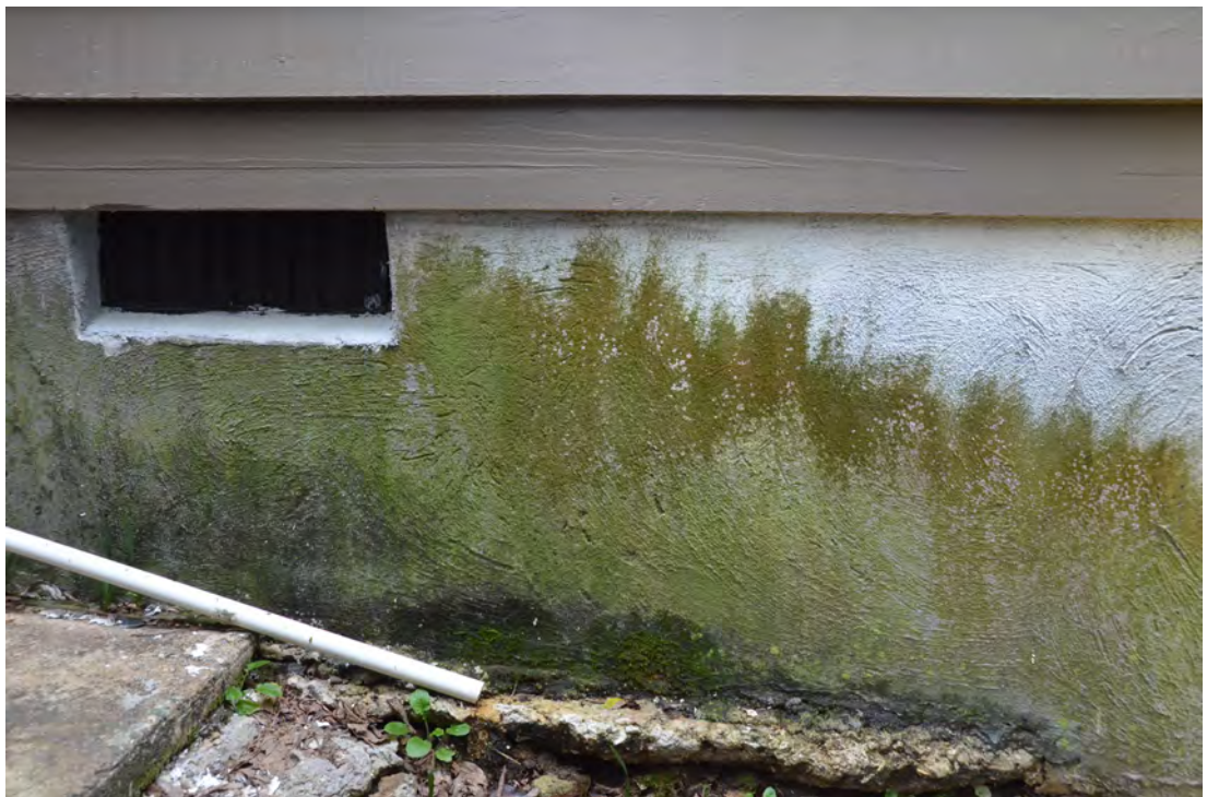
Figure 20. Biogrowth on the West Foundation Wall of the Outbuilding.
