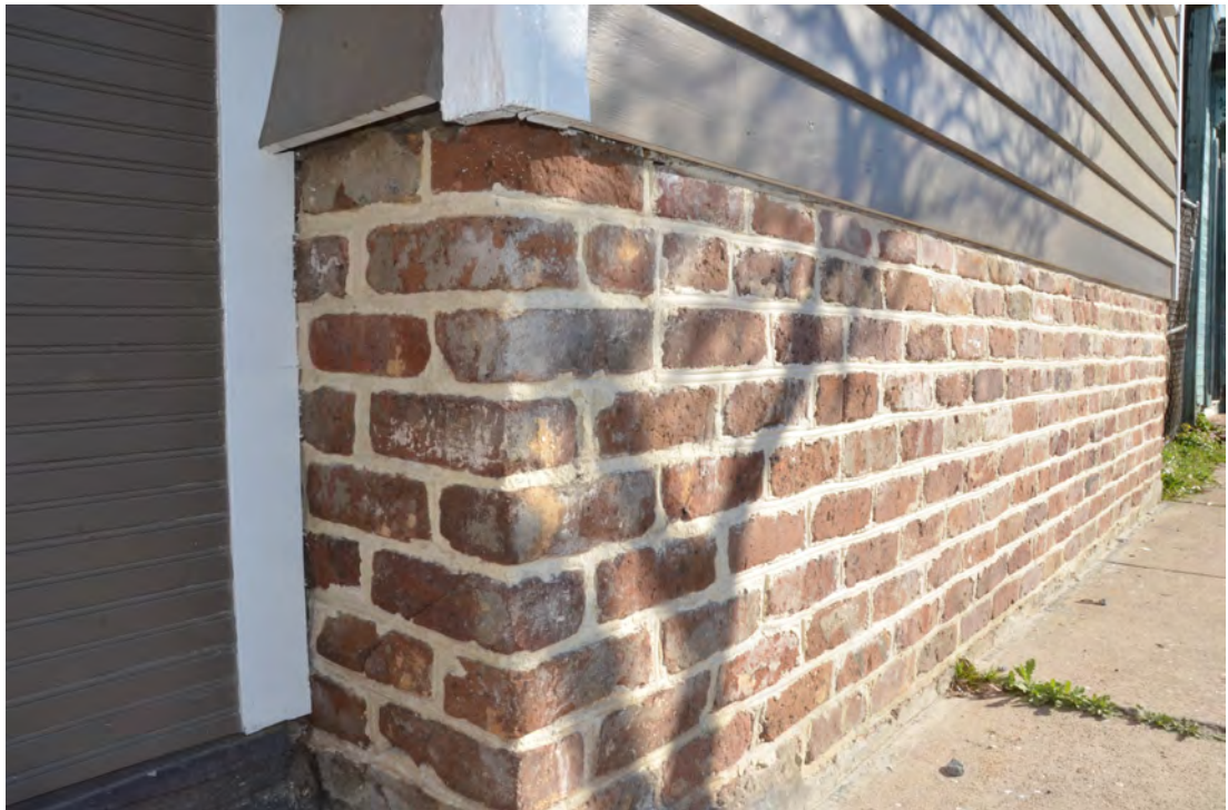
Figure 18. Repointed South Foundation Wall.
