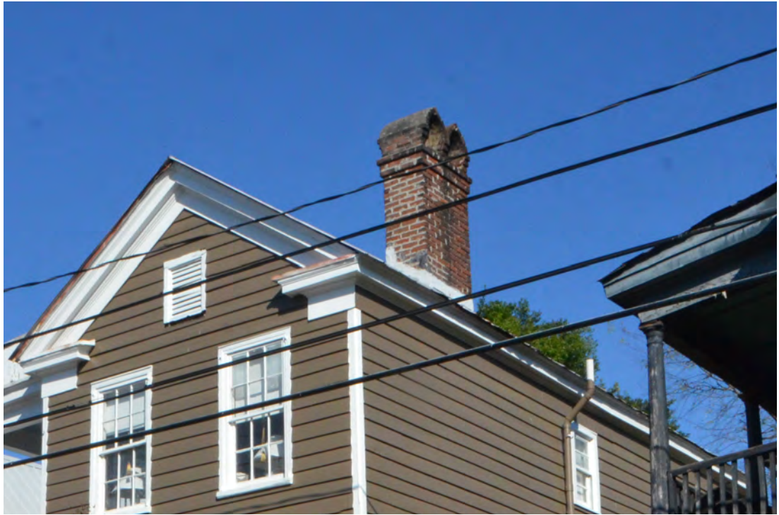
Figure 37. Loss of Mortar on the Chimney.
