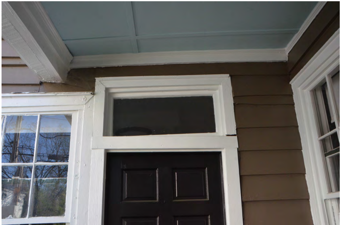
Figure 32. Shifting of Fenestrations on the 1st Level.
