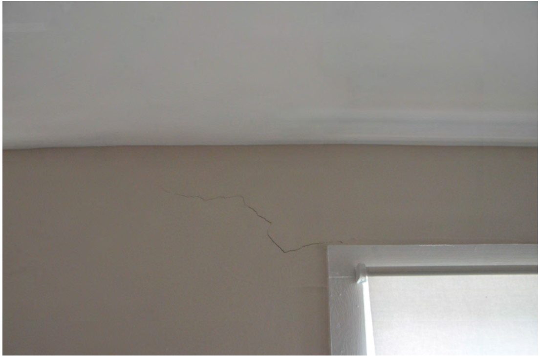
Figure 79. Diagonal Crack in the Plaster at Corner of the Window.
