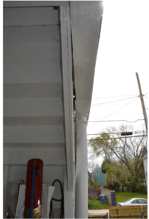
Figure 53. Outward Bowing of the Piazza Columns.
