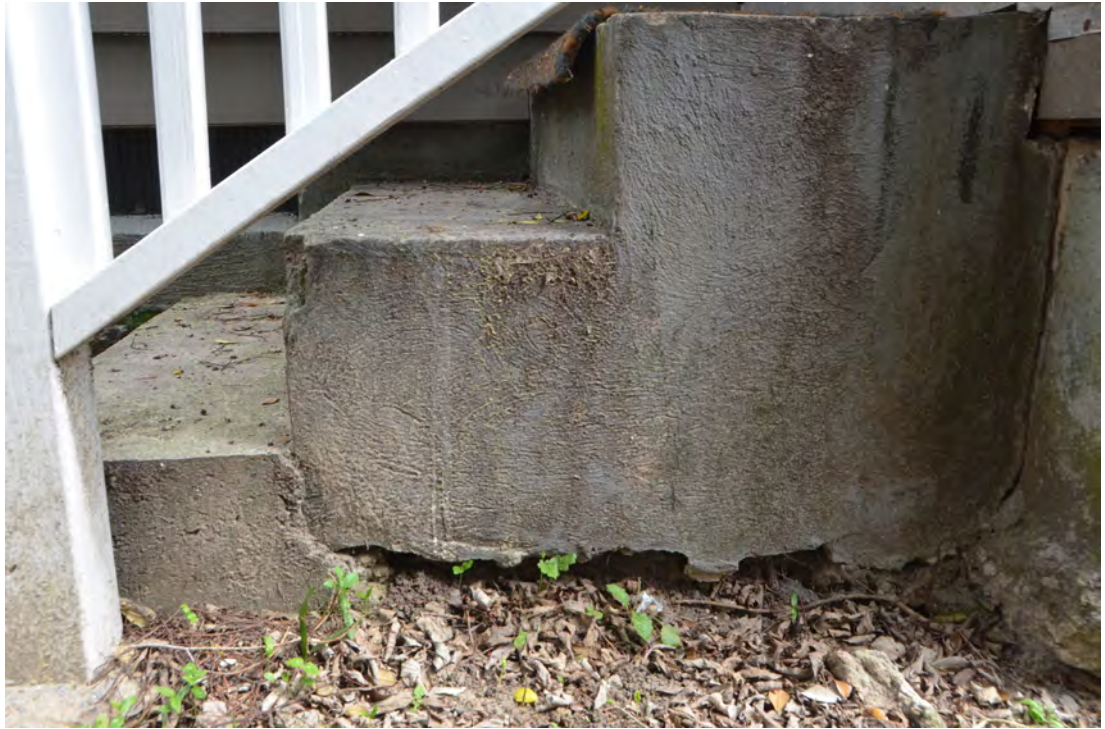
Figure 21. Soil Washout at the Rear Stairs.
