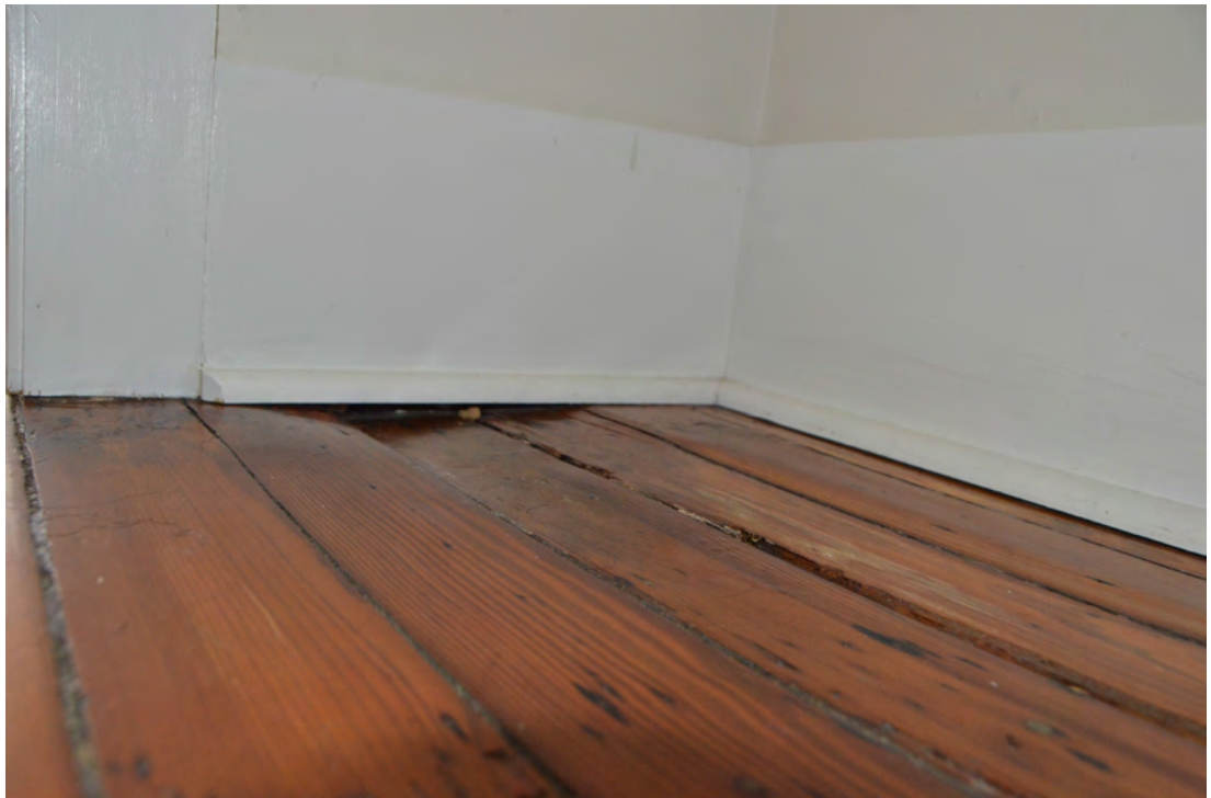
Figure 68. Deformation and Settlement of the Wood Flooring.
