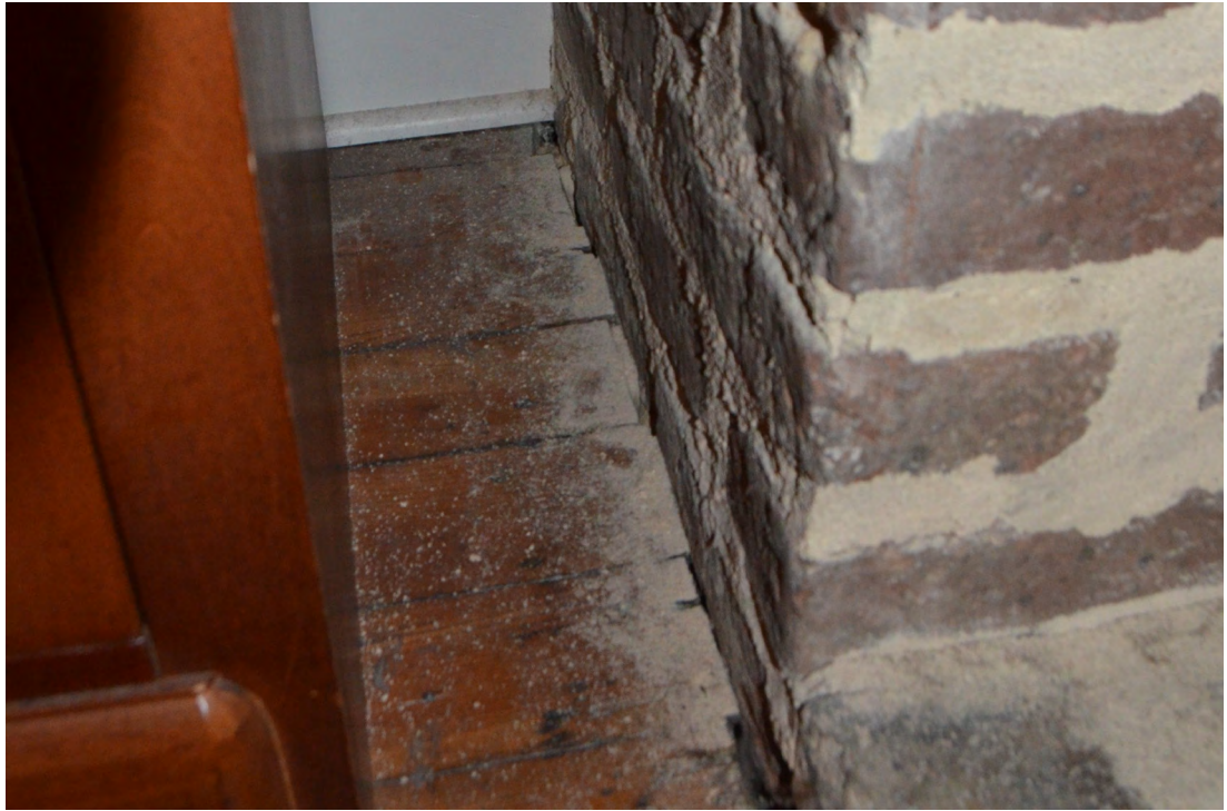
Figure 77. Inappropriate Mortar Repair and “Dusting”.
