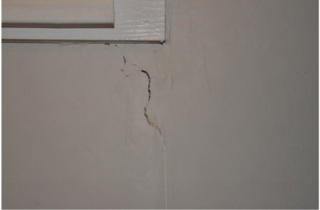
Figure 81. Crack in the Plaster at Corner of the Window.
