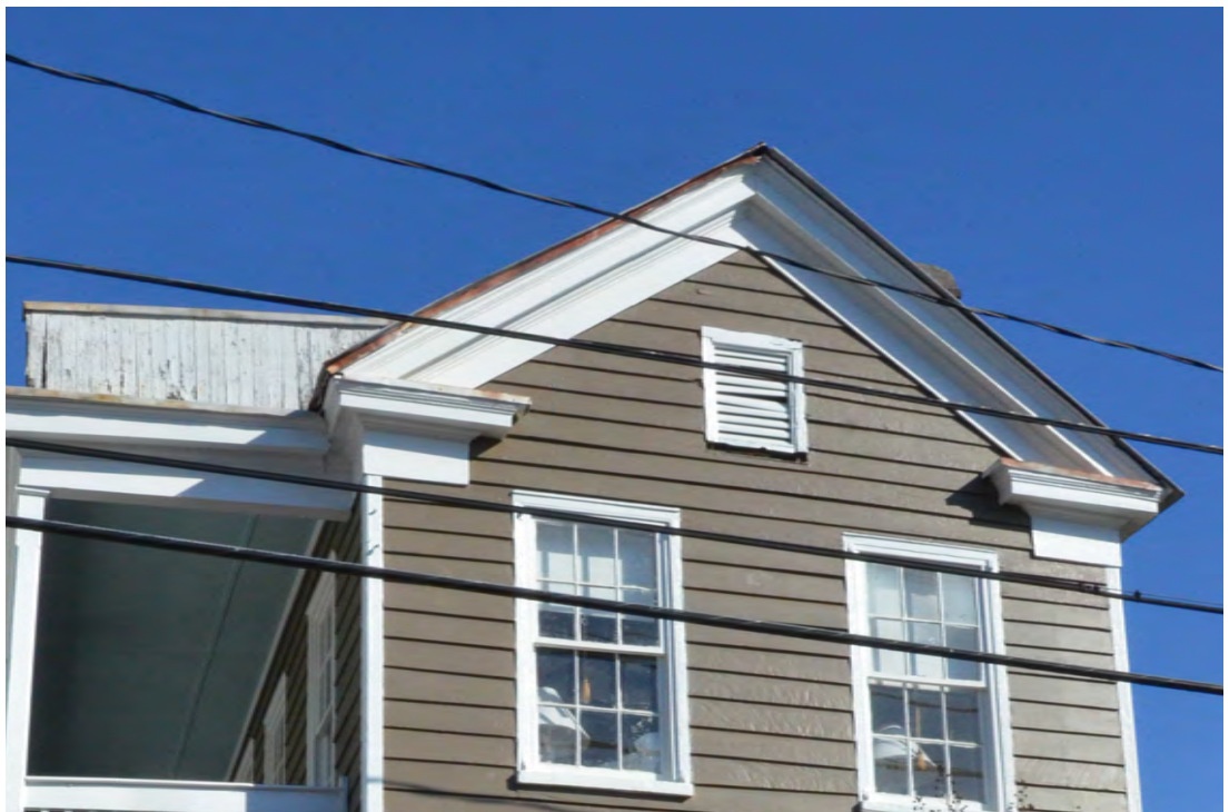
Figure 36. Corroded Flashing at the South Facade Gable.
