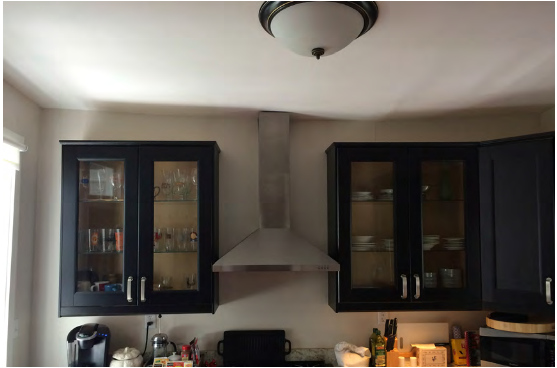
Figure 91. Ceiling Deformation in the Kitchen Addition.
