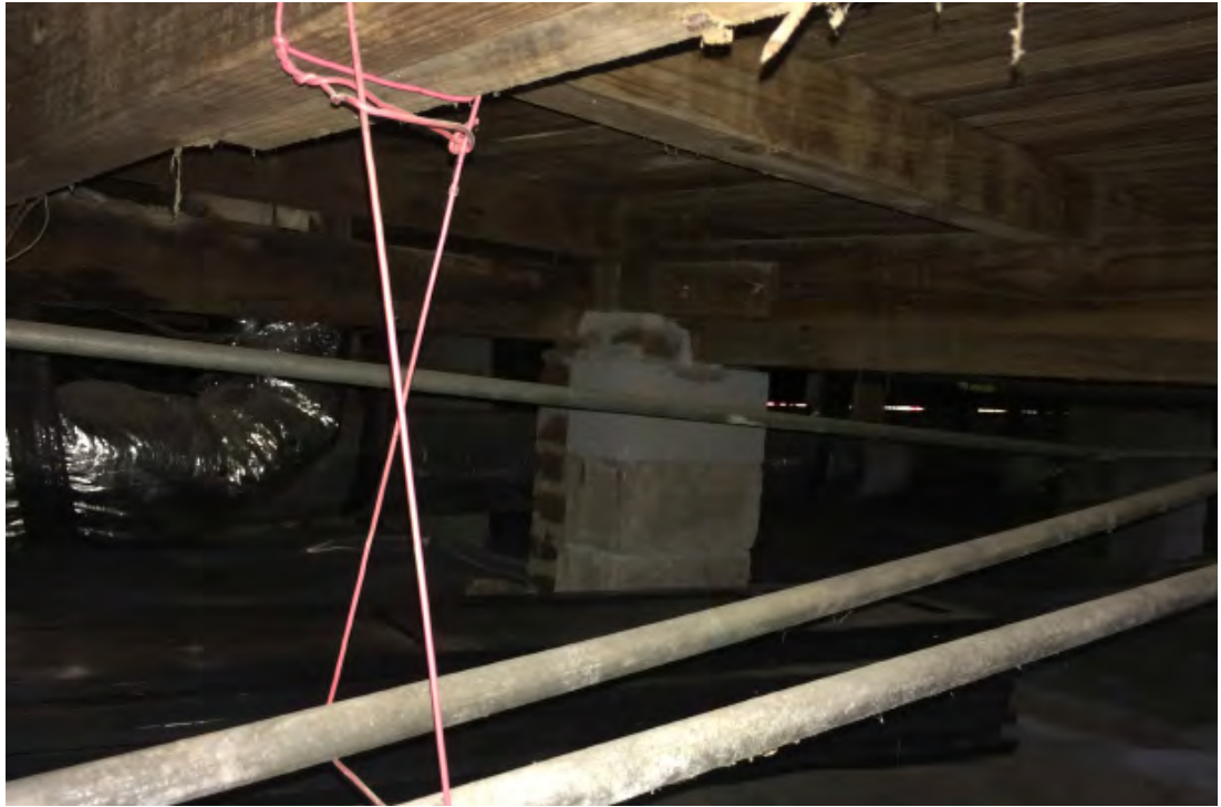
Figure 93. New CMUs beneath the house strengthening the masonry piers.
