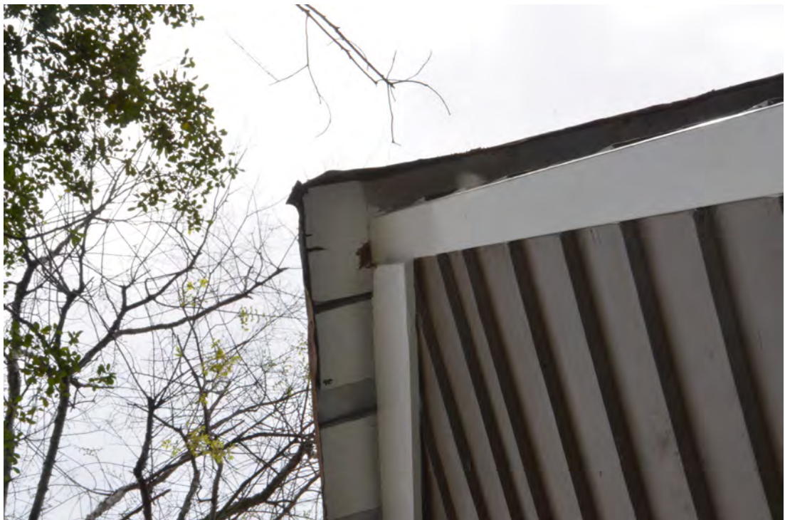
Figure 38. Deteriorated Rafters Beneath the Gable of the Outbuilding.
