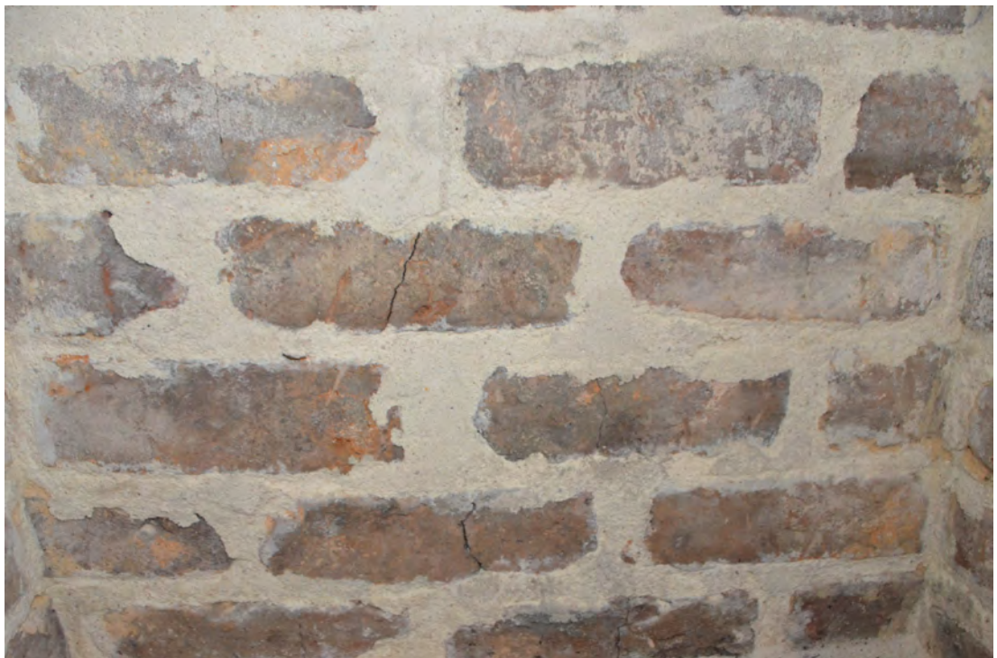
Figure 76. Cracking Bricks in the Fireplace Box.
