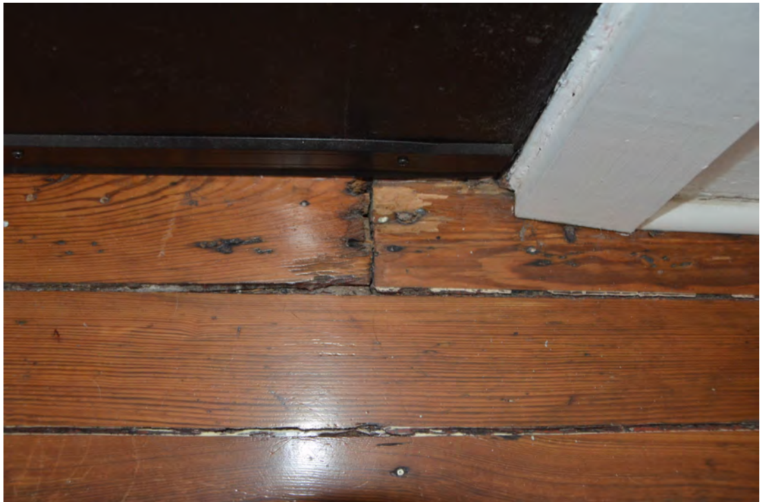
Figure 64. Deterioration of the Wood Flooring.
