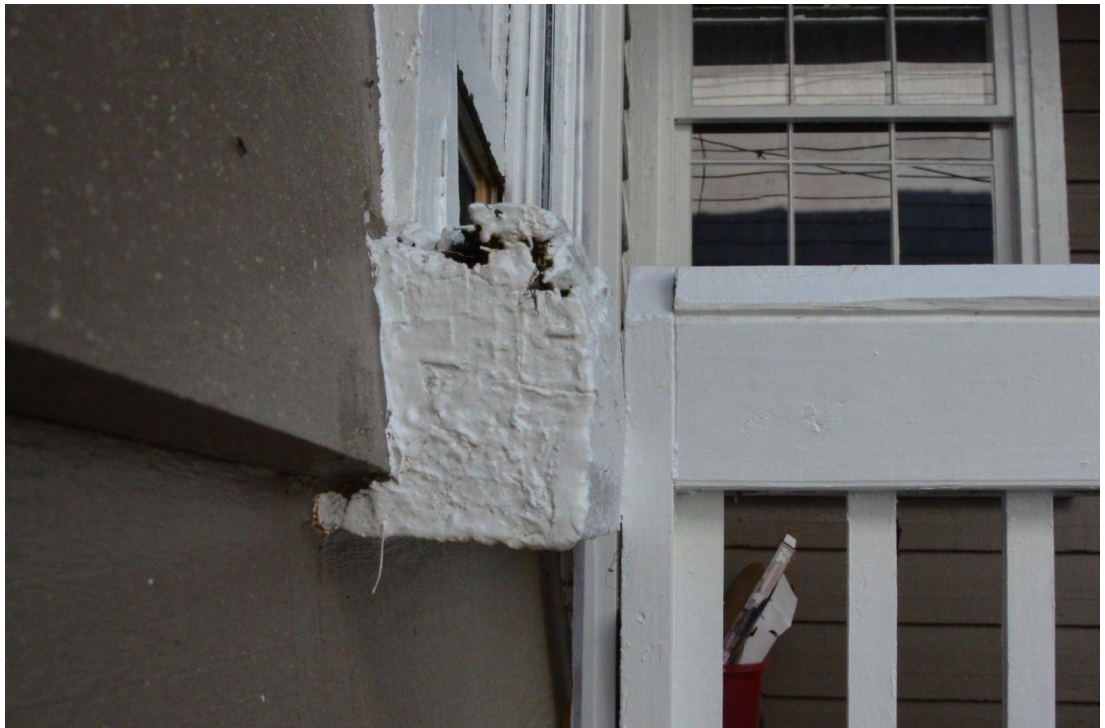
Figure 30. Wood Rot on a Windowsill.
