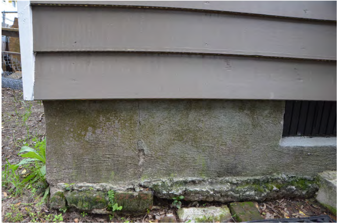
Figure 23. Soil Washout at the West Elevation.
