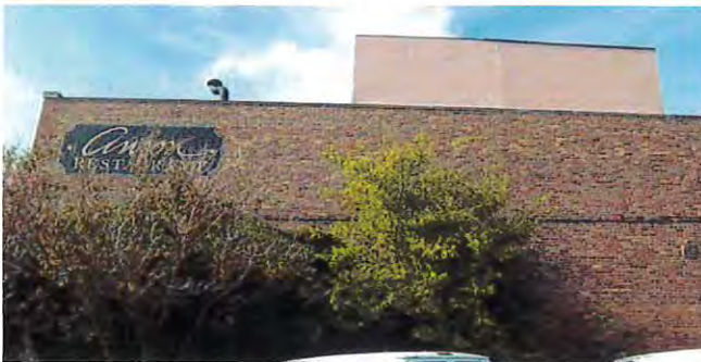
Figure 6. Rooftop addition that possibly required replacement of gable roof. The distinct brick course is possibly part of a vestigial wall of a sister building depicted in the 1928, 1944 and 1951 Sanborn maps. Photo taken September 2011.
