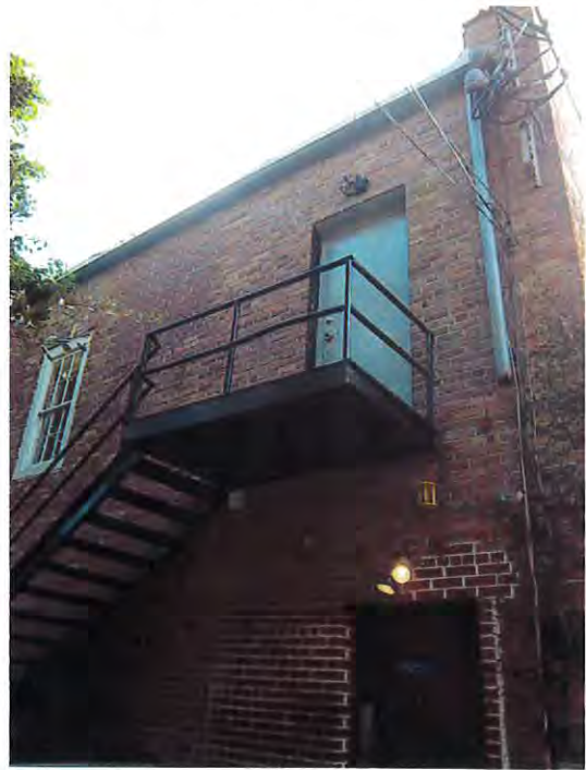
Figure 5. West (rear) elevation of 12 Anson with evidence of ground floor door alteration and rear window installed in 1995. Note also the change in color and pattern to the upper right of window indicating a previous, larger opening.
