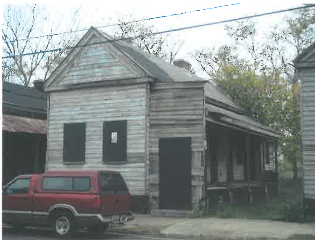
Figure 13: 195 Jackson Street, horizontal clapboard on surrounding doorway leading to piazza matches what is on the house. Photo by the author, November 2009.
