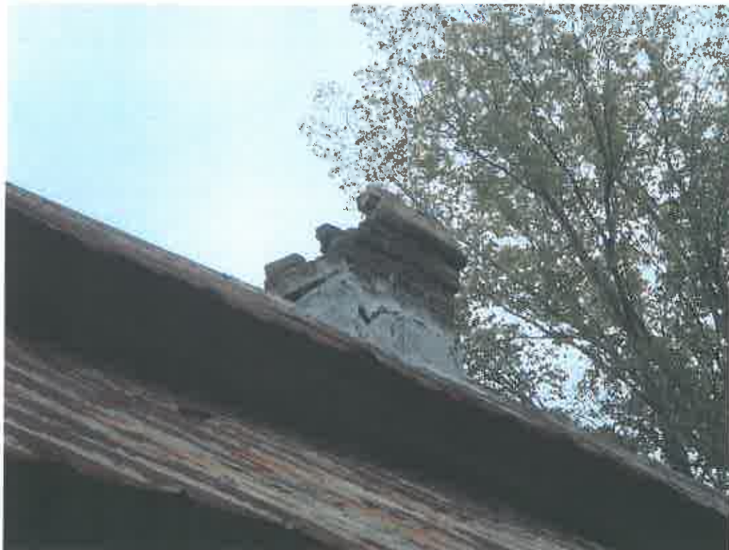
Figure 9: 199 Jackson Street, Chimney. Photo by the author, November 2009.
