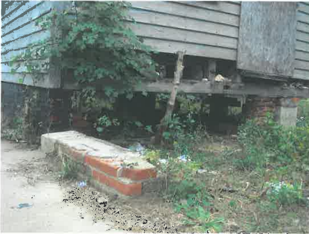
Figure 10: 197 Jackson Street, open foundation. Photo by the author, November 2009.
