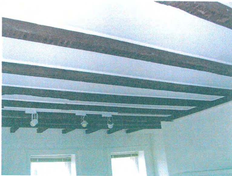
Timber ceiling joists on 3rd floor
