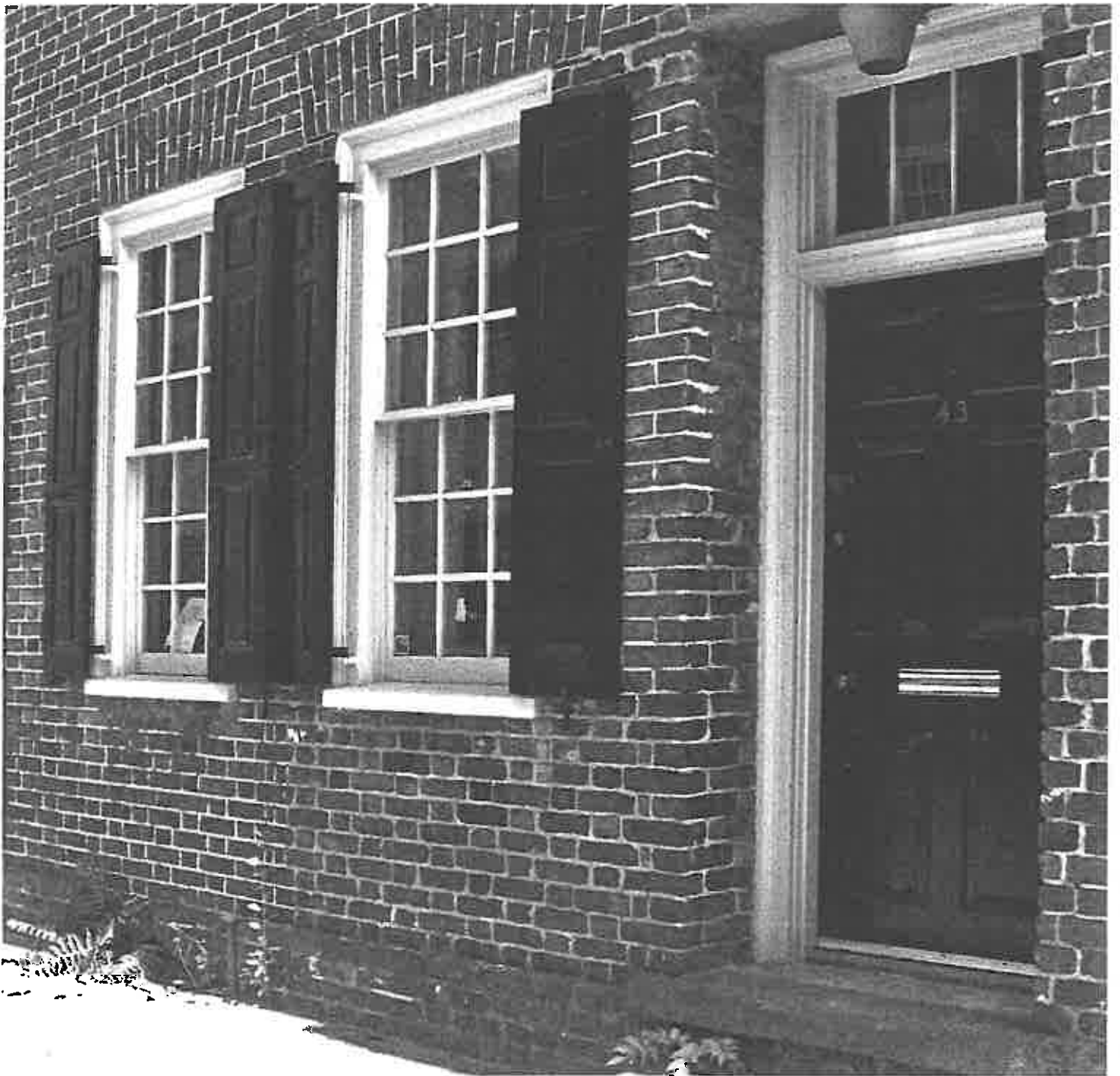
43 Tradd Street Existing Conditions
