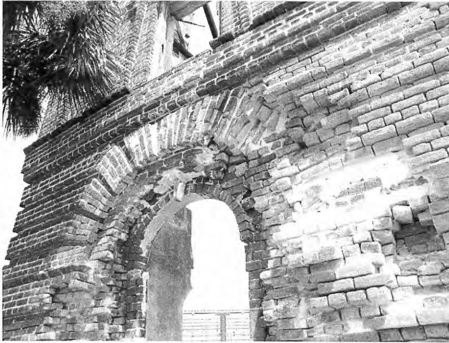
Eroded tabby has led to sloughing of original bricks.
