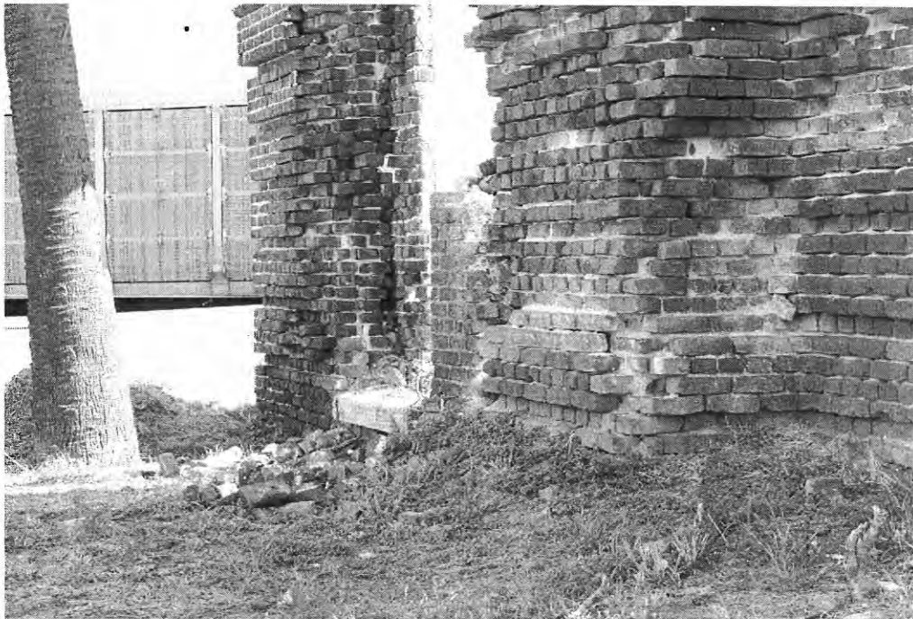
Eroded tabby has led to sloughing of original bricks.
