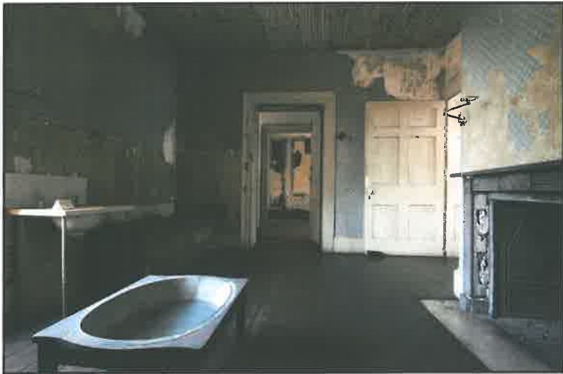
The northeast dressing room at the Aiken-Rhett House. Note the exposed lathe ceiling and peeling wall paper.
