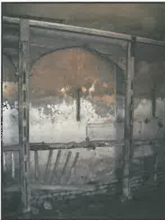
Stables in the West Dependency. Note the wood to ground contact, failing stable balustrade, failing ceiling plaster, and woodwork no longer connected to the ceiling.
