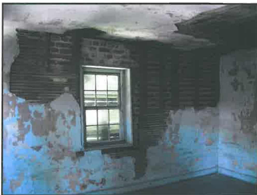
Failing wall and ceiling plaster in the north room of the slave quarters.
