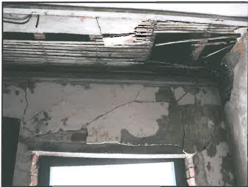
Failing wall and ceiling plaster atop the East Dependency exit.
