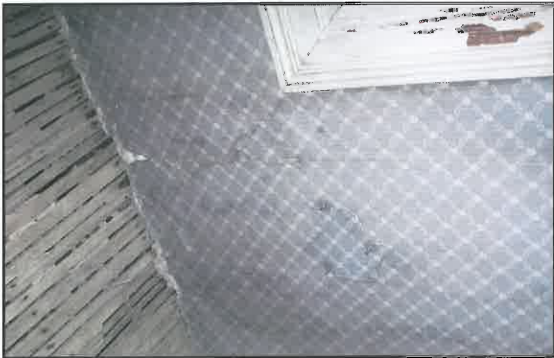
Detail of the northeast dressing room at the Aiken-Rhett House. The exposed lathe ceiling abuts re-pinned wall paper.
