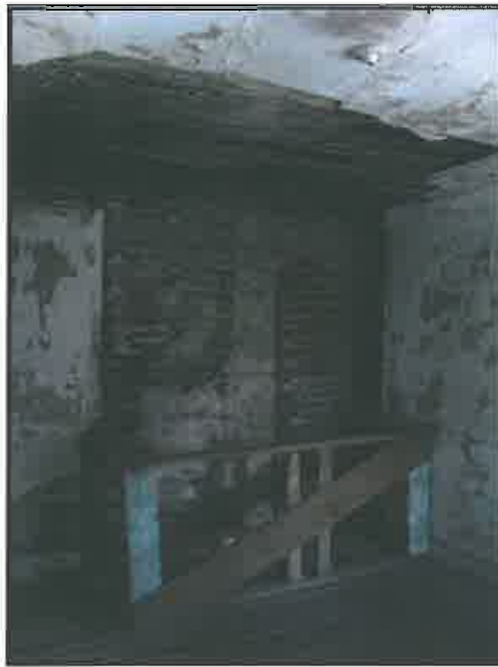
Failing wall and ceiling plaster in the north room of the slave quarters. Also note the temporary barricade surrounding the chimney flues. This chimney was removed after extensive damage following Hurricane Hugo in 1989.
