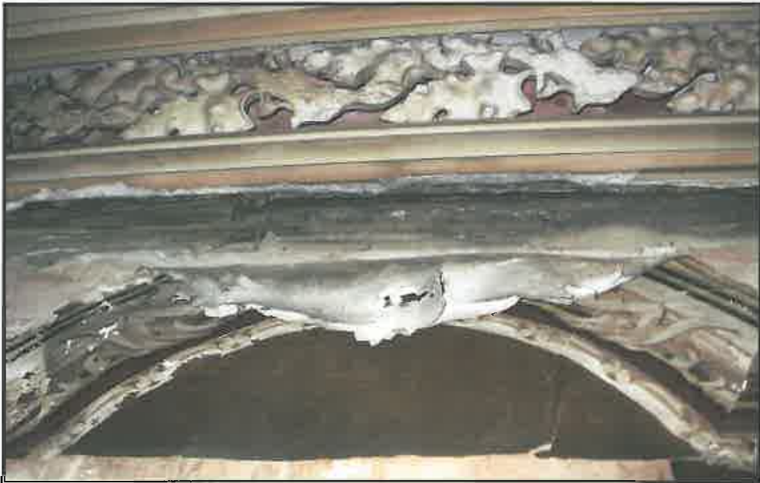
The withdrawing room at the Aiken-Rhett House. Details of the deteriorated wallpaper and plaster.
