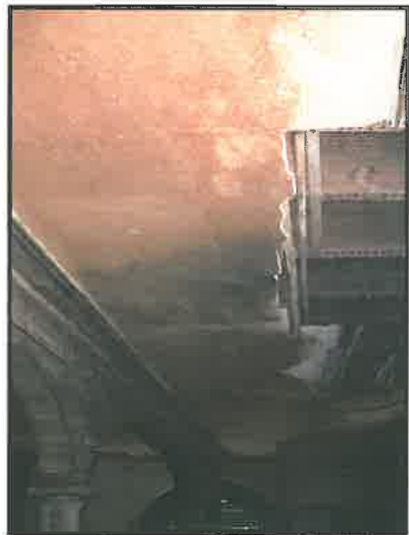
Stables in the West Dependency. Note the wood to ground contact, failing stable balustrade, failing ceiling plaster, and woodwork no longer connected to the ceiling.
