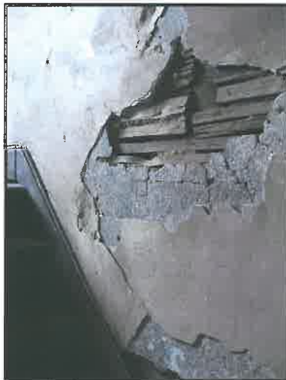
Failing plaster surrounding the stairway in the East Dependency.
