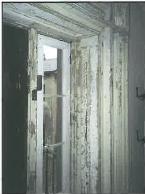
Detail of typical peeling paint at the Aiken-Rhett House.
