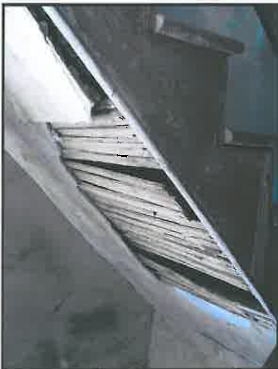
Failing plaster surrounding the stairway in the East Dependency.
