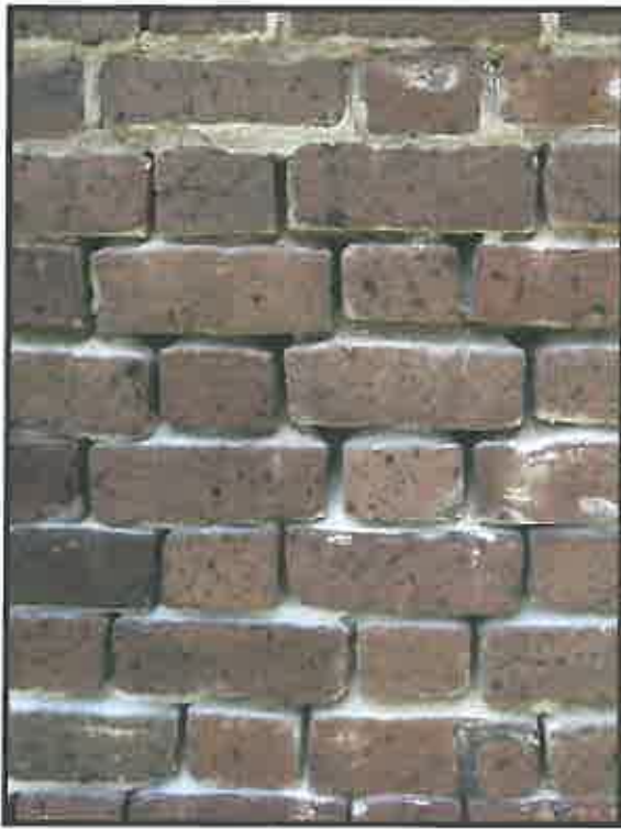
Absent mortar between bricks on the north wall of the property.
