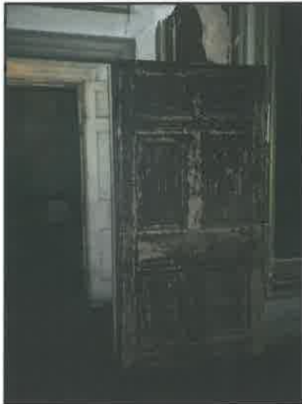
Detail of peeling paint and wall paper in the withdrawing room at the Aiken-Rhett House.
