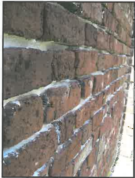
Absent mortar between bricks on the north wall of the property.
