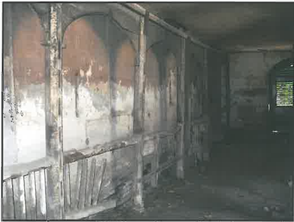
Stables in the West Dependency. Note the wood to ground contact, failing stable balustrade, and woodwork no longer connected to the ceiling.
