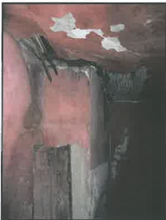
Failing wall plaster in two of the slave quarters. Note the dripped paint as a result of a previous ceiling repair in the yellow room.
