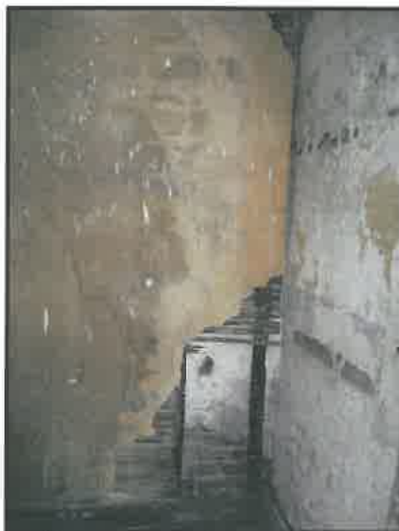
Failing wall plaster in two of the slave quarters. Note the dripped paint as a result of a previous ceiling repair in the yellow room.
