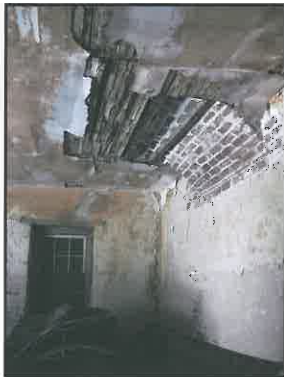
Failing ceiling plaster in the carriage house.
