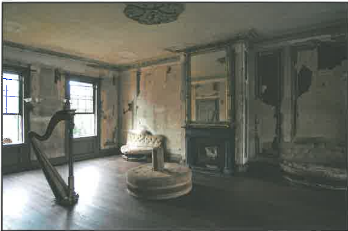
The withdrawing room at the Aiken-Rhett House. Note the deteriorated wallpaper and plaster against the patching above the windows and on the ceiling.
