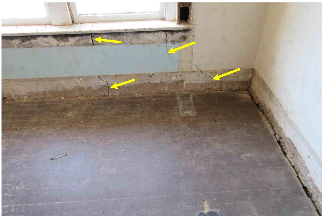
Photo 16: Typical crack in a second floor HCT wall due to a window header failure below.
