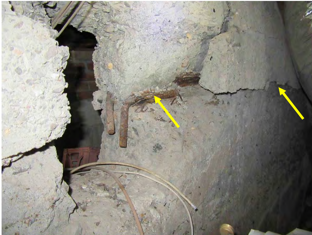
Photo 3: Opening through an interior foundation wall. The horizontal rebar is visible at the spalled concrete and horizontal crack.
