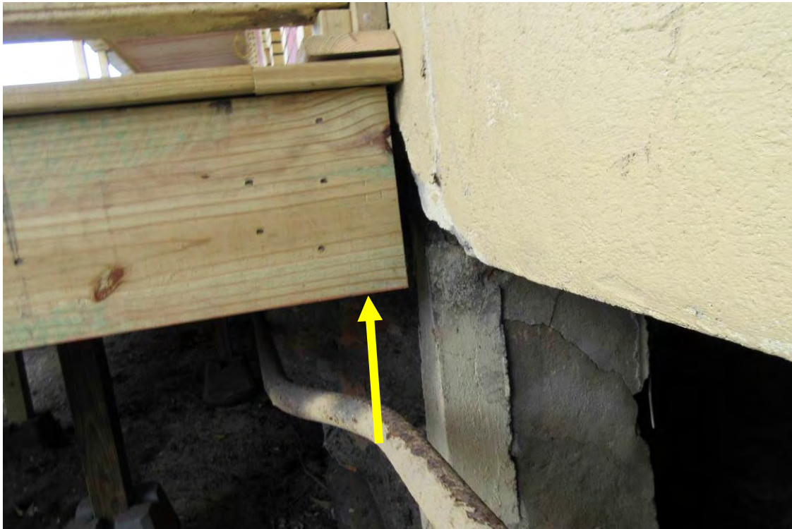
Photo 23: No support was provided for the deck band beam in this location.
