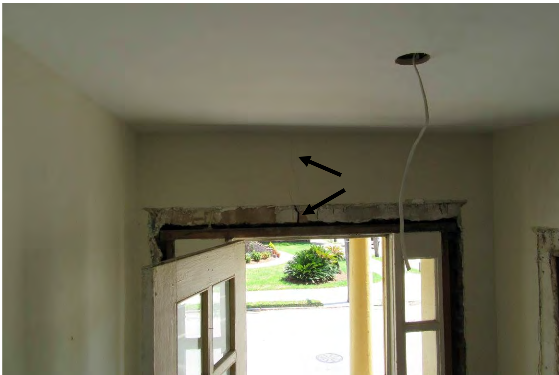
Photo 14: Crack in the HCT load-bearing wall header above a front door (arrow).
