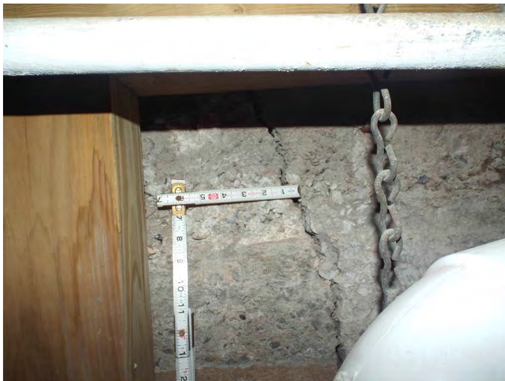
Photo 7: Through-wall crack in the north exterior foundation wall below Unit 11.
