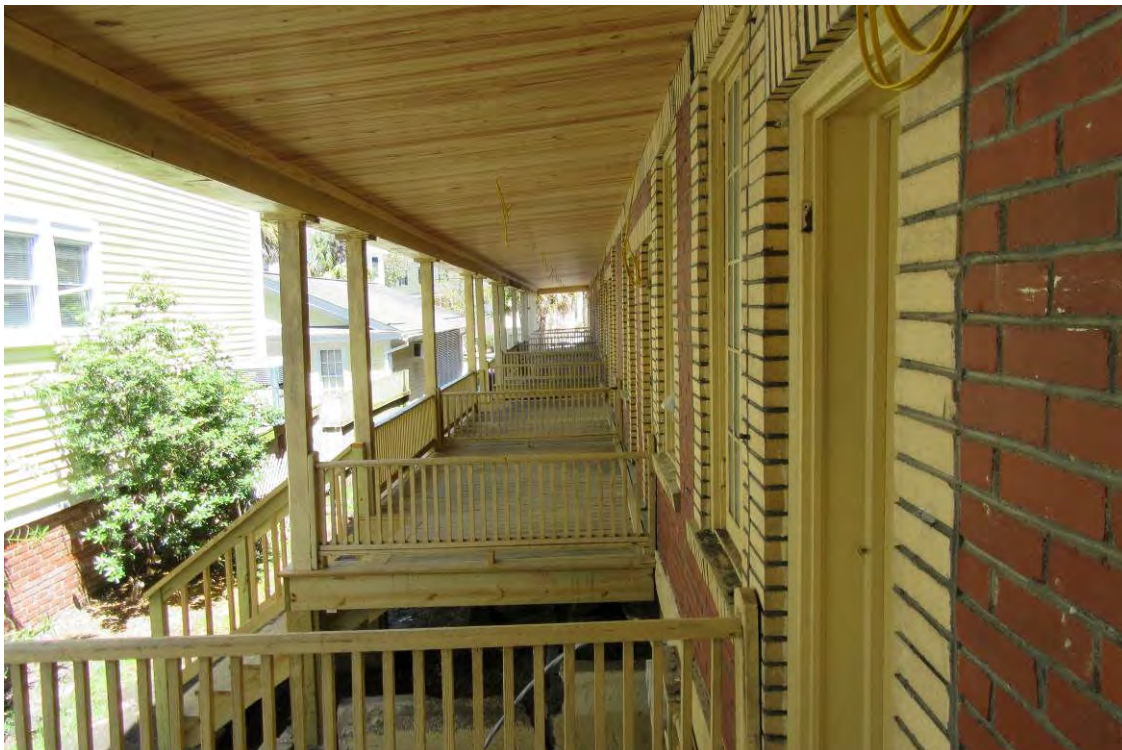
Photo 22: New deck framing, flooring, and ceiling on the rear of the building.
