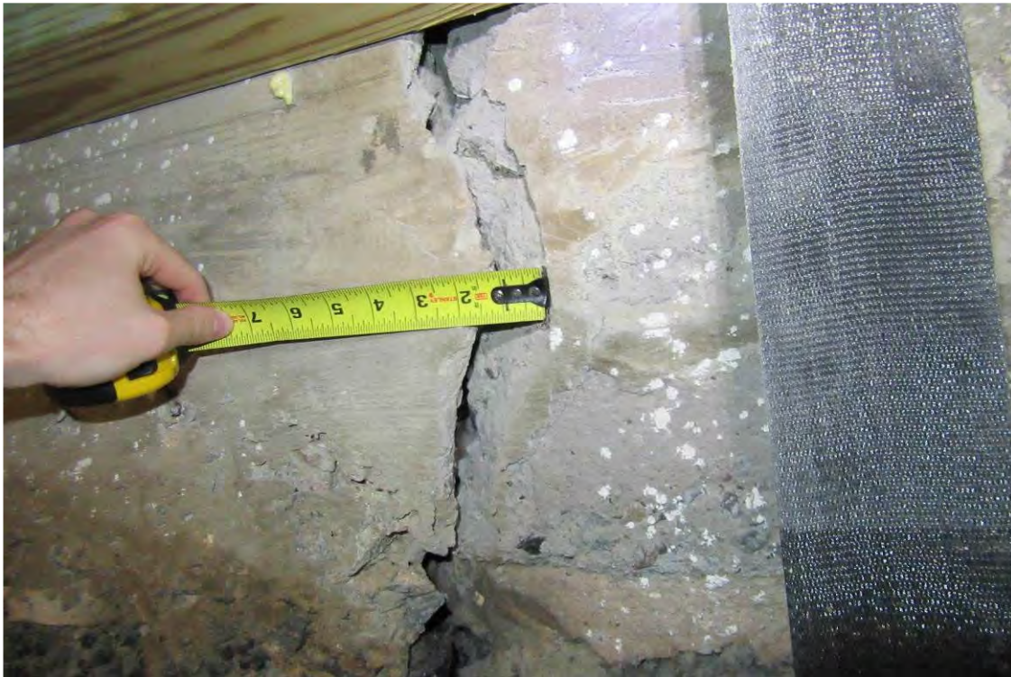
Photo 5: Through-wall crack in the south exterior foundation wall below Unit 1.
