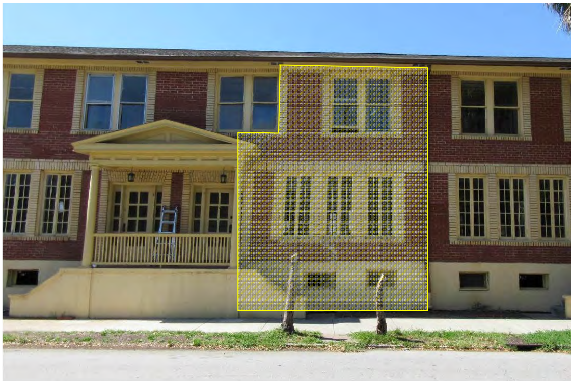
Photo 10: Front elevation of unit 7. The hatched wall section will need to be removed and rebuilt.
