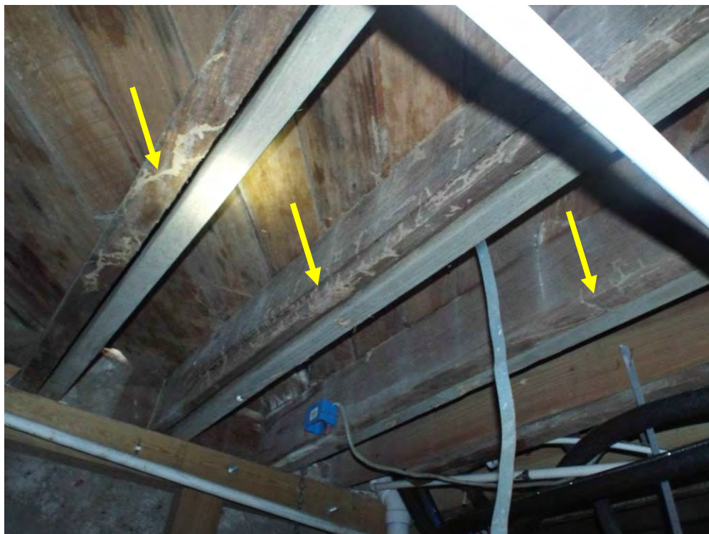
Photo 19: Evidence of termite infestation and damage was observed in some locations. Termite tubes are visible on three floor joists in this photo (arrows). Note the recent addition of a bolted ledger and post in the background, presumably repairs to damaged joists in this location.
