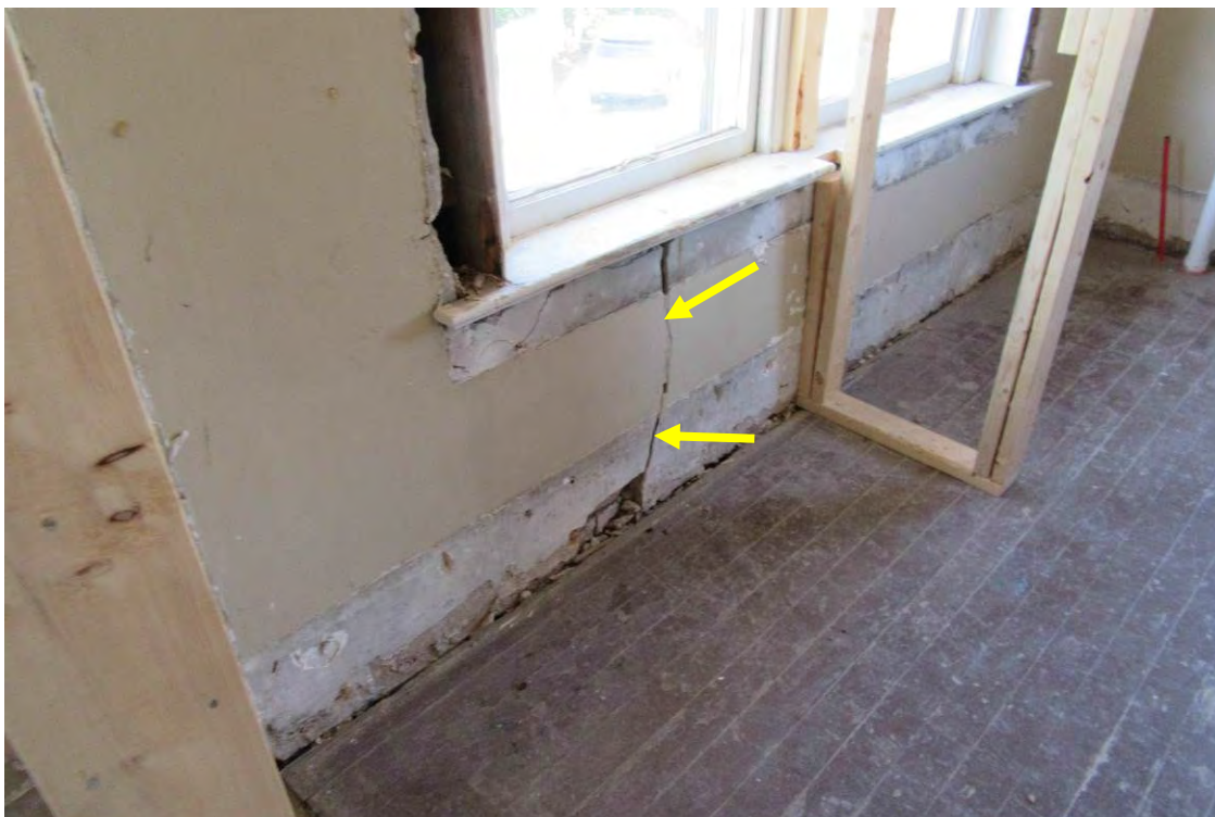
Photo 15: Typical crack in a second floor HCT wall due to a window header failure below.
