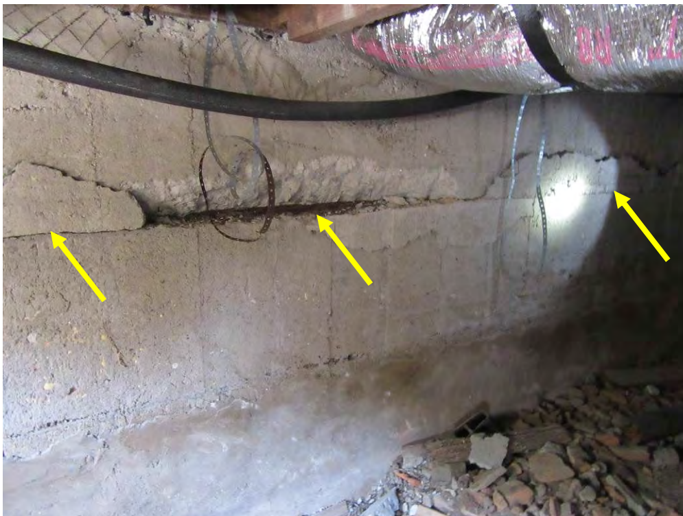
Photo 2: Typical horizontal crack caused by rebar corrosion at an interior foundation wall. The corroded rebar is visible at the center of the photo.
