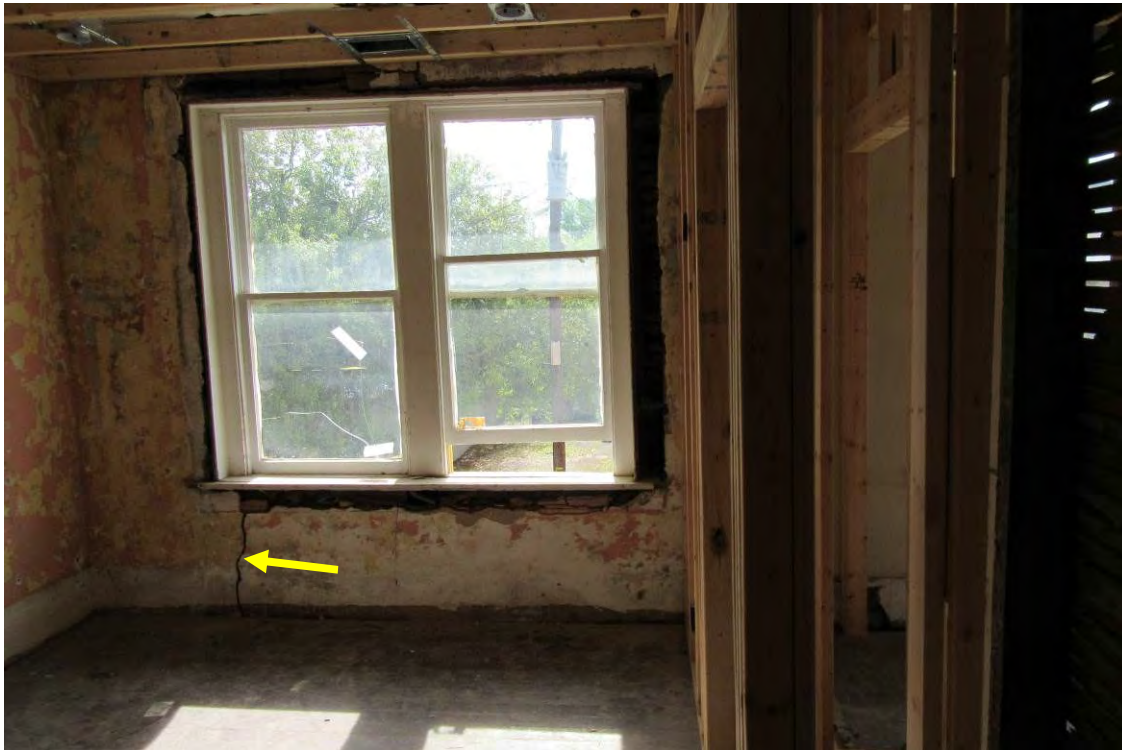
Photo 17: Typical crack in a second floor HCT wall due to a window header failure below.
