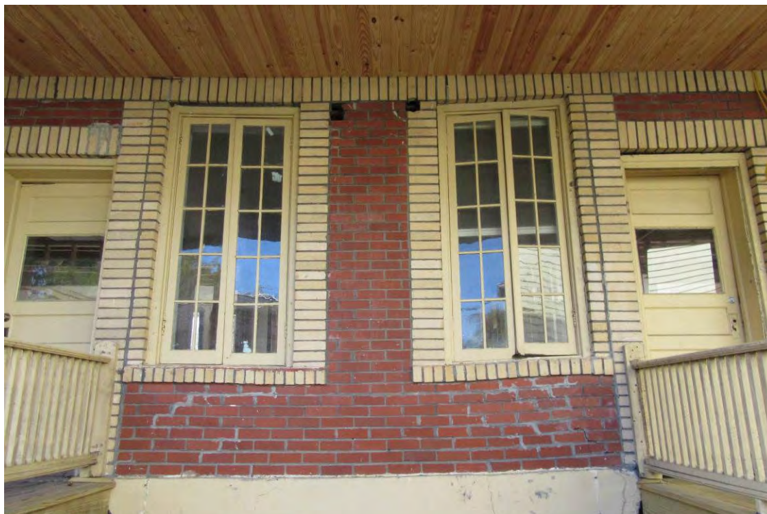
Photo 12: Rear wall section between units 5 and 7. Foundation damage below this wall (see photo 8) will require the wall to be removed and rebuilt up to the roof.
