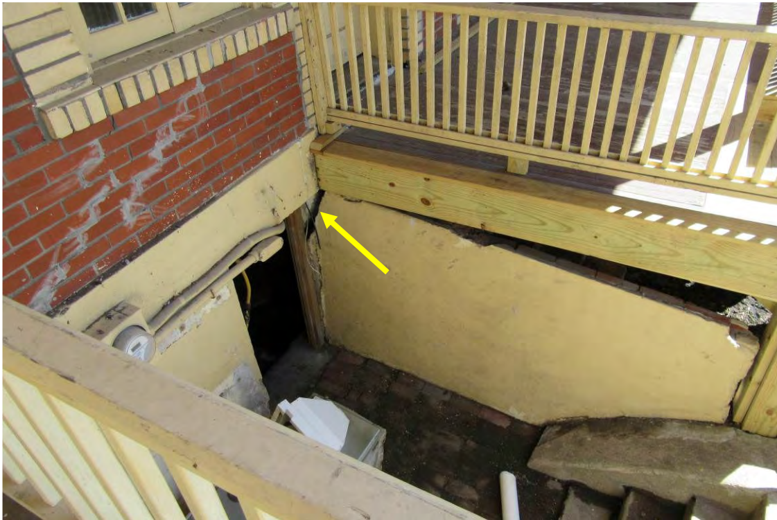
Photo 9: Concrete wall segment between units 9 and 11. Note the typical foundation wall fracture at the adjacent knee wall (arrow).
