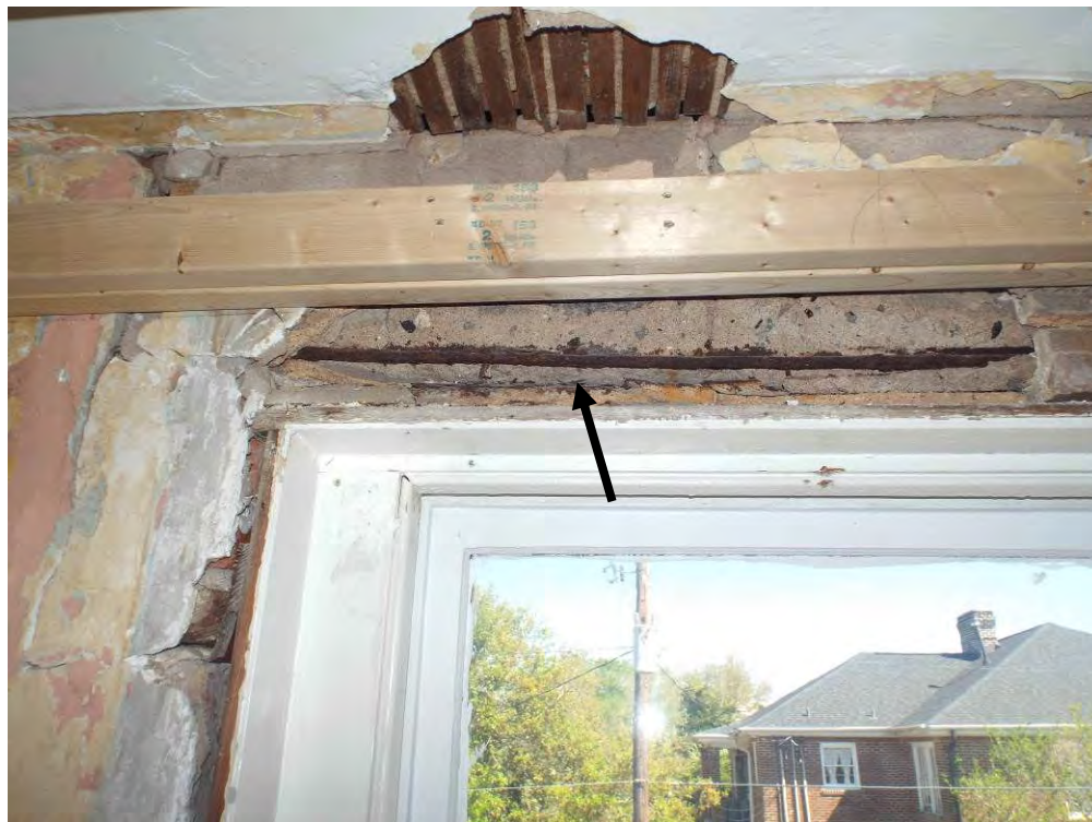
Photo 18: A reinforced masonry header was observed in one location. The rebar was exposed, corroded, and section loss was observed (arrow).
