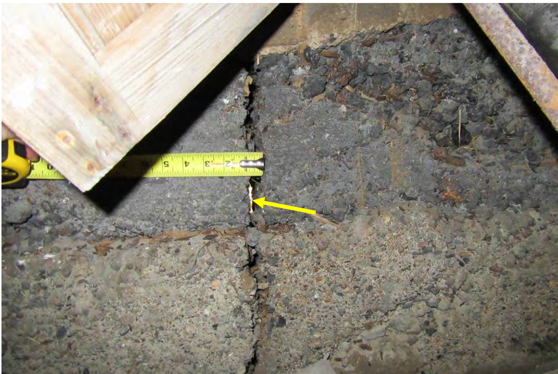
Photo 6: Through-wall crack in the east exterior foundation all below unit 1. Daylight can be seen through the crack (arrow).
