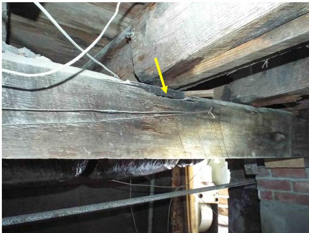
Photo 20: Typical example of moisture and possible insect related damage to a first floor drop girder (arrow).
