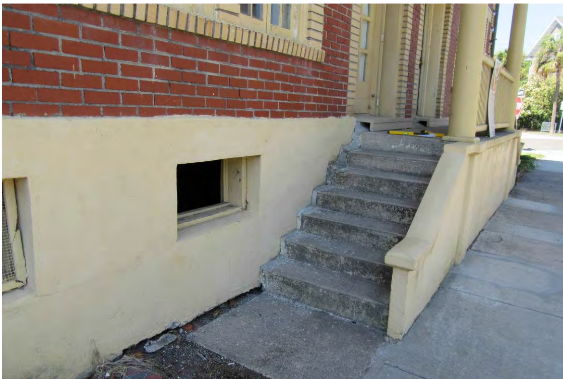
Photo 25: Grout or repair mortar was noted between the front stoops and the building foundation wall. It was reported that this cavity was filled as the stoops settled.
