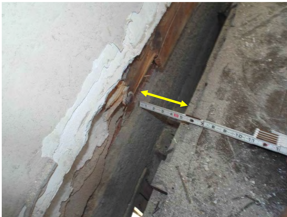
Photo 11: Unit 7 – The exterior wall has pulled approximately 5 inches away from the first floor framing in this location (arrow). The floor support girder below is at risk of losing support if the wall shifts closer to the street.
