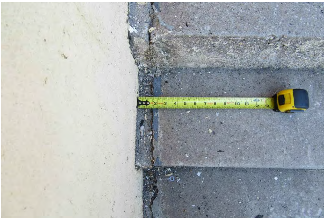
Photo 26: Grout or repair mortar was noted between the front stoops and the building foundation wall. It was reported that this cavity was filled as the stoops settled.
