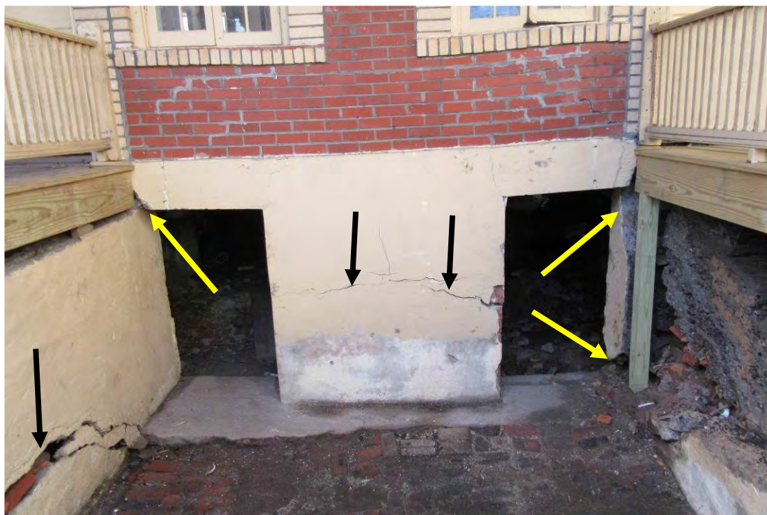
Photo 8: Foundation wall segment between Units 5 and 7. Note the horizontal crack in the foundation wall; the large fracture in the foundation wall to the right of the rightmost access door adjacent to the concrete stoop; the spalled concrete above the leftmost access door, and the large crack in the concrete knee wall on the left of the photo.
