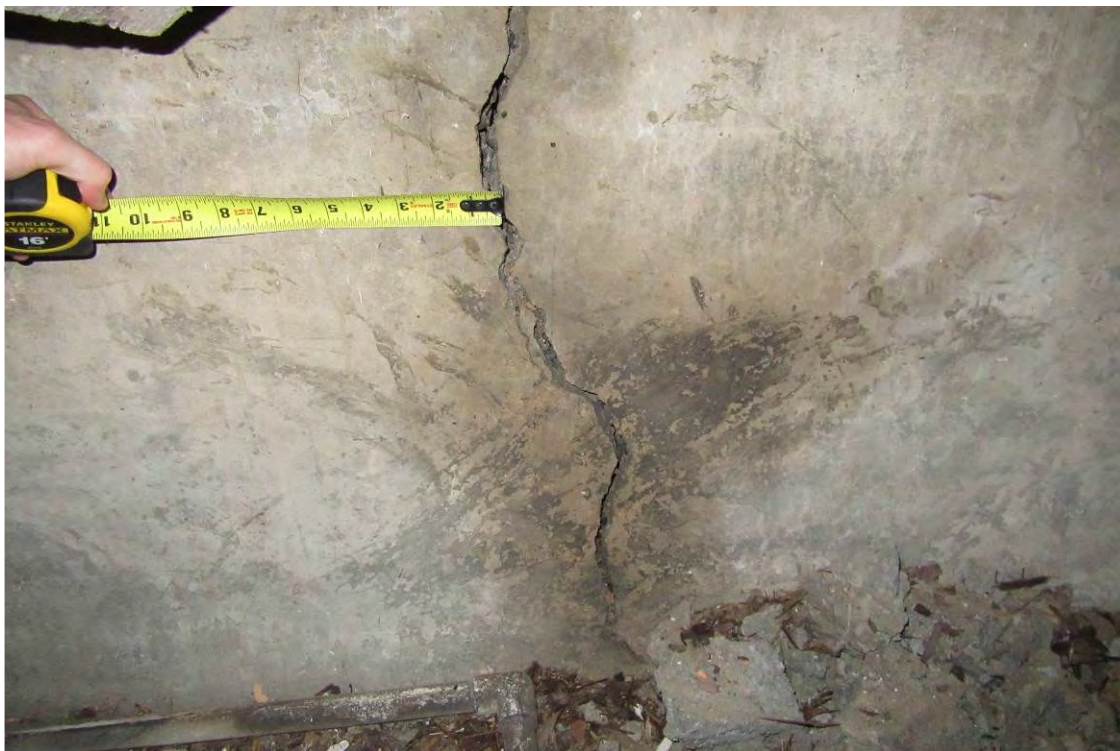
Photo 4: Vertical through-wall crack in the west exterior foundation wall below Unit 1.
