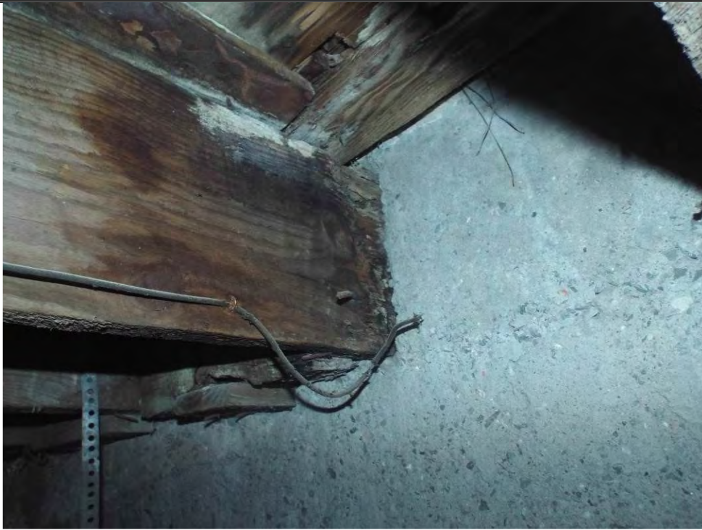
Photo 21: Typical example of moisture damage where a floor joist is embedded into the concrete foundation wall.
