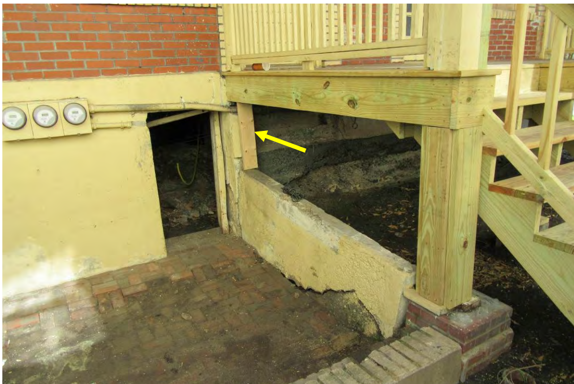
Photo 24: New rear deck framing supported by a single 2x member on unstable knee wall (arrow).
