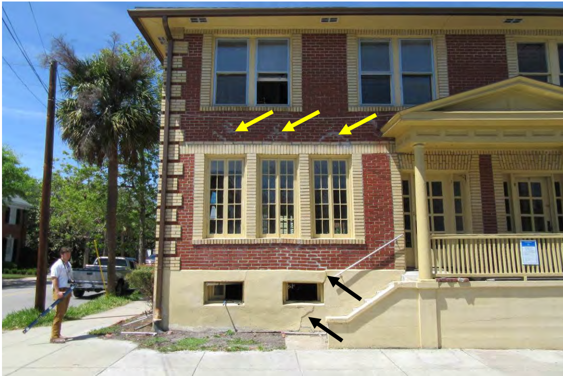
Photo 13: Front elevation of Unit 1. Note the typical cracks above the failing window headers. Note the through wall foundation crack and header failure above the crawl space vent.
