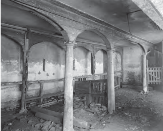
Figure 5.78: Interior photo of the portion of the carriage house containing the stables. There are pointed gothic arches between the columns, 1979. (Library of Congress, Prints and Photographs Division, Historic American Buildings Survey, HABS SC,10-CHAR,177B-6, http://hdl.loc.gov/loc.pnp/hhh.sc0025 )
