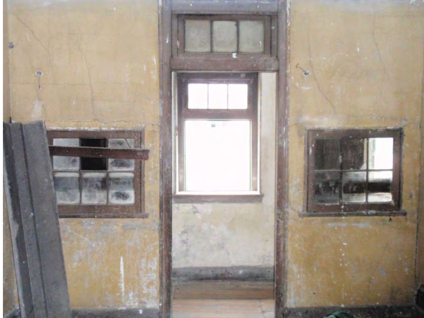
Figure 5. 80: View from one of the interior servant's rooms into the hallway that has the exterior windows. Note the windows on the interior hall wall that help provide light to the rooms. (Photo by Author, 2010)
