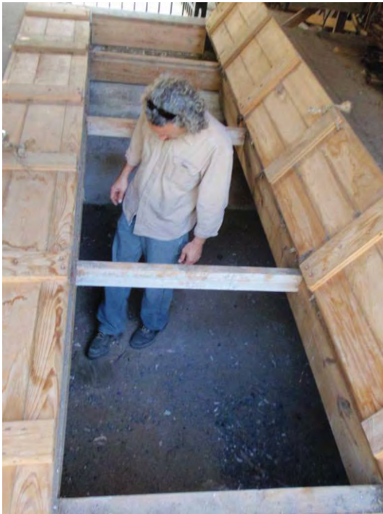
Figure 5.53: The doors leading to the tabby pit below the raised portion of the floor. (Photo by Author, 2009)
