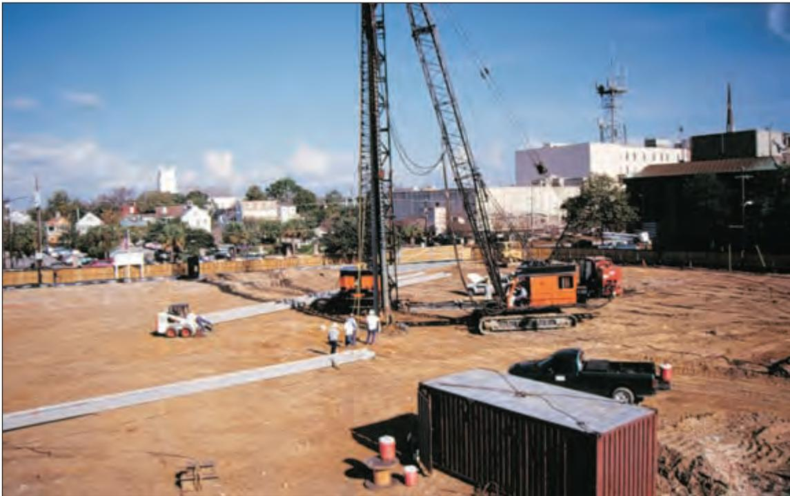
Drilling for a test piling. The cement test pilings in the background are lying across several archaeological features. The process of installing and testing the pilings prevented access to most of the archaeological site. Looking northeast.
