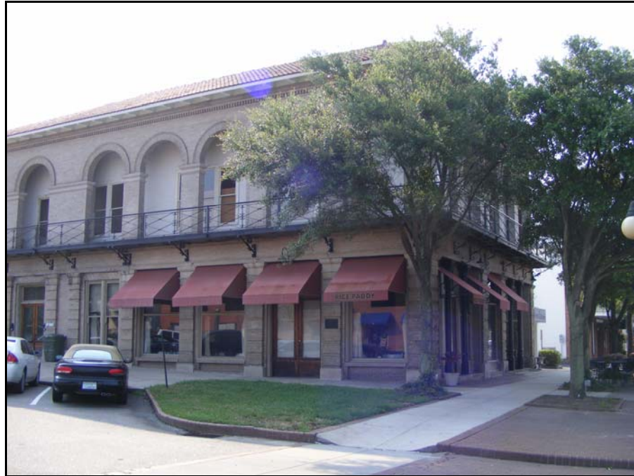
Figure 22. Spanish Colonial Revival style commercial building at 732 Front Street (Site No. 191-0246)
