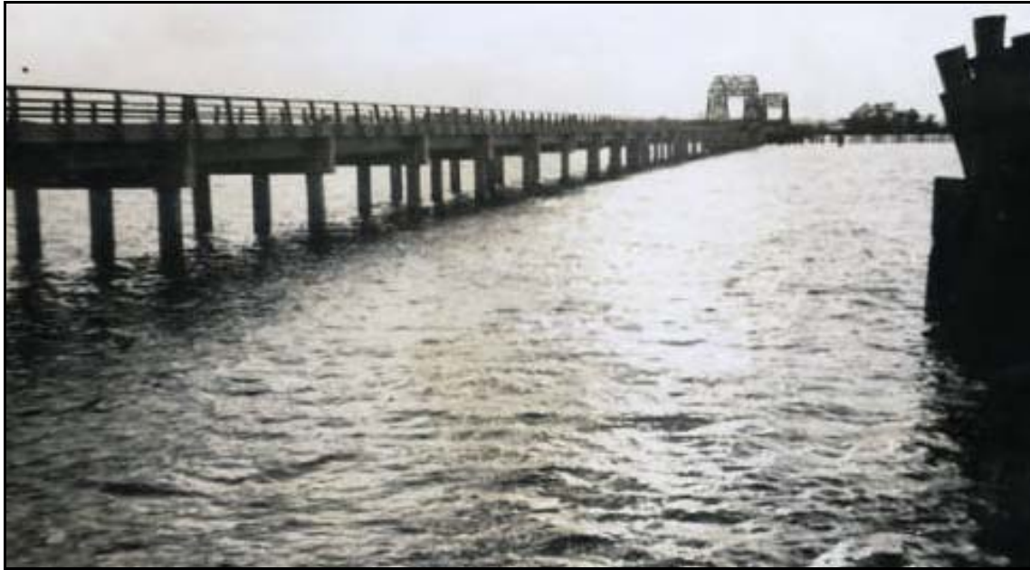
Figure 4. The Lafayette Bridge over the Black and Waccamaw Rivers at Georgetown photographed shortly before its opening in 1935. The bridge was the last link in the route of US 17 between Maine and Florida. It also replaced the ferries that had carried passenger and vehicular traffic since colonial days. Source: Georgetown Digital Library
