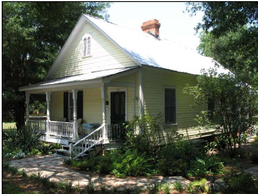
Figure 31. Frame Vernacular house at 215 St. James Street (Site No. 191-0217)
