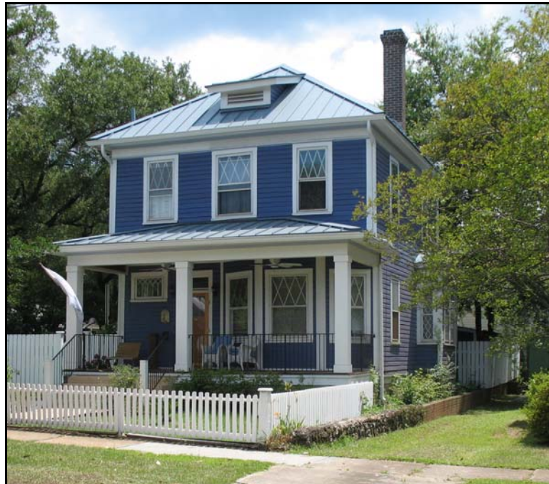
Figure 23. American Foursquare at 1201 Prince Street (Site No. 191-0519)
