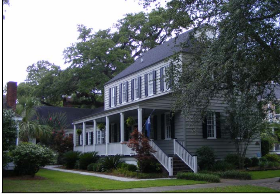
Figure 11. Georgetown Single House at 513 Prince Street (Site No. 191-0127)
