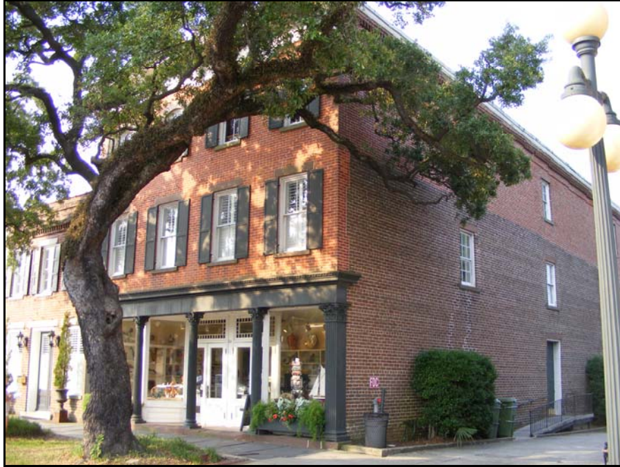
Figure 20. Two-Part Commercial block at 633 Front Street (Site No. 191-0199)
