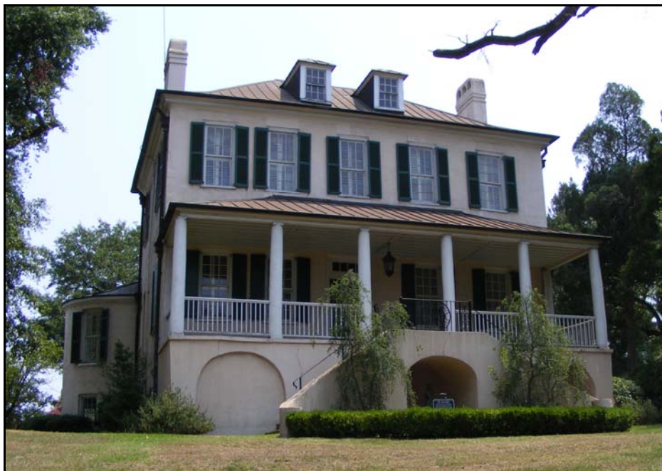
Figure 12. Robert Stewart House with Federal-style alterations (Site No. 191-0075)
