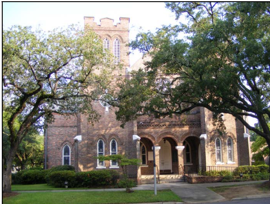
Figure 15. Gothic Revival style Bethel A.M.E. Church at 417 Broad Street (Site No. 191-0158)
