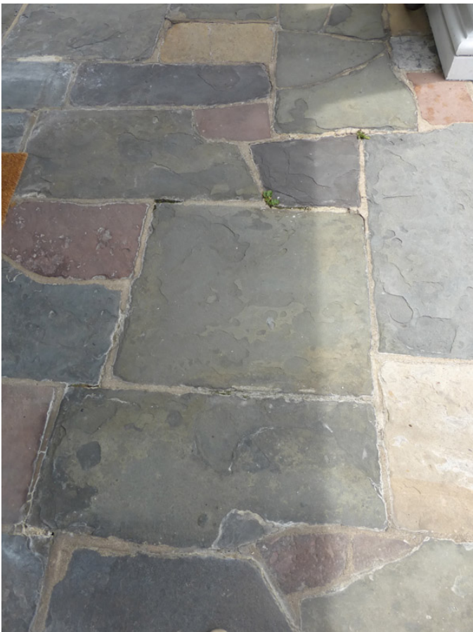
4 EXISTING FLAGSTONE PORCH P-3
