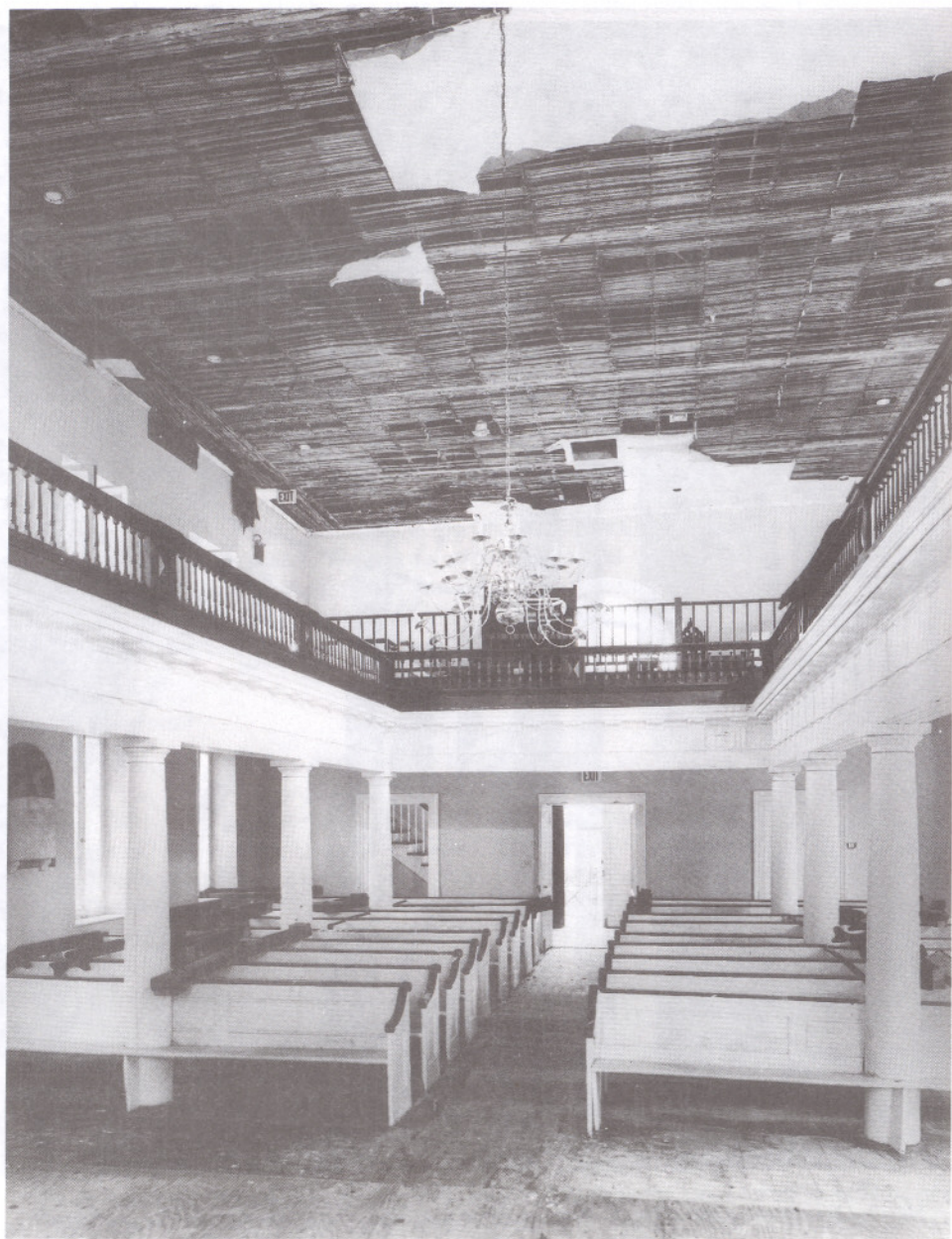
FIG. 3—St. Stephen's Episcopal Church, damage to interior following Hugo and subsequent rains (Jack Boucher, HABS photograph).
