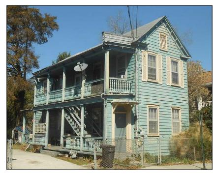
pendants. Although the current shutters are modern replacements, pintles for shutters are still in place. The windows and attic vent on the street façade have slightly peaked architraves. At some point during the 20th century, a second floor was added to what had originally been a single story segment at the rear of the house. The piazza screen and hood over the door seem to be replacements.
