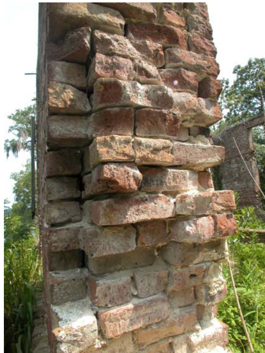
Figure 6.8 Stoke Rice Mill, 2006 Broken bricks that need repair Photo by author
