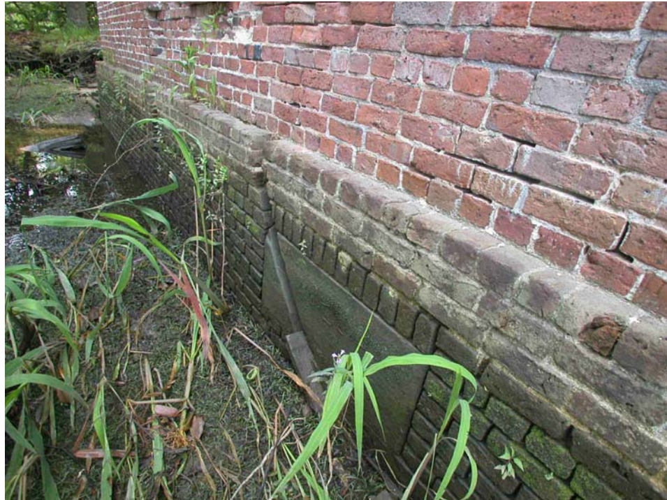
Figure 6.5 Stoke Rice Mill, 2006 Rising damp and fungal growth on the exterior Photo by author
