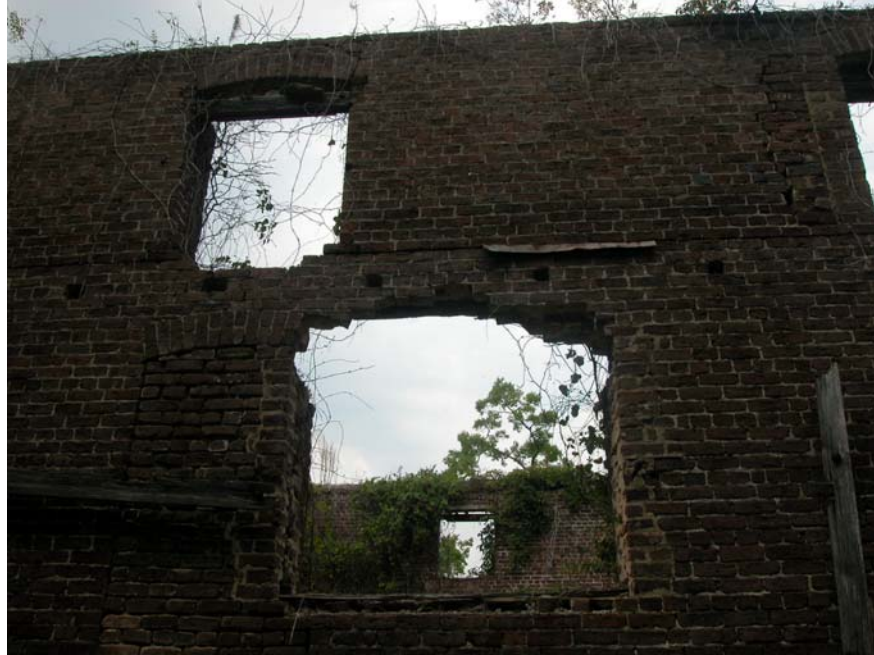
Figure 6.9 Stoke Rice Mill, 2006 Unstable window alignment Photo by author
