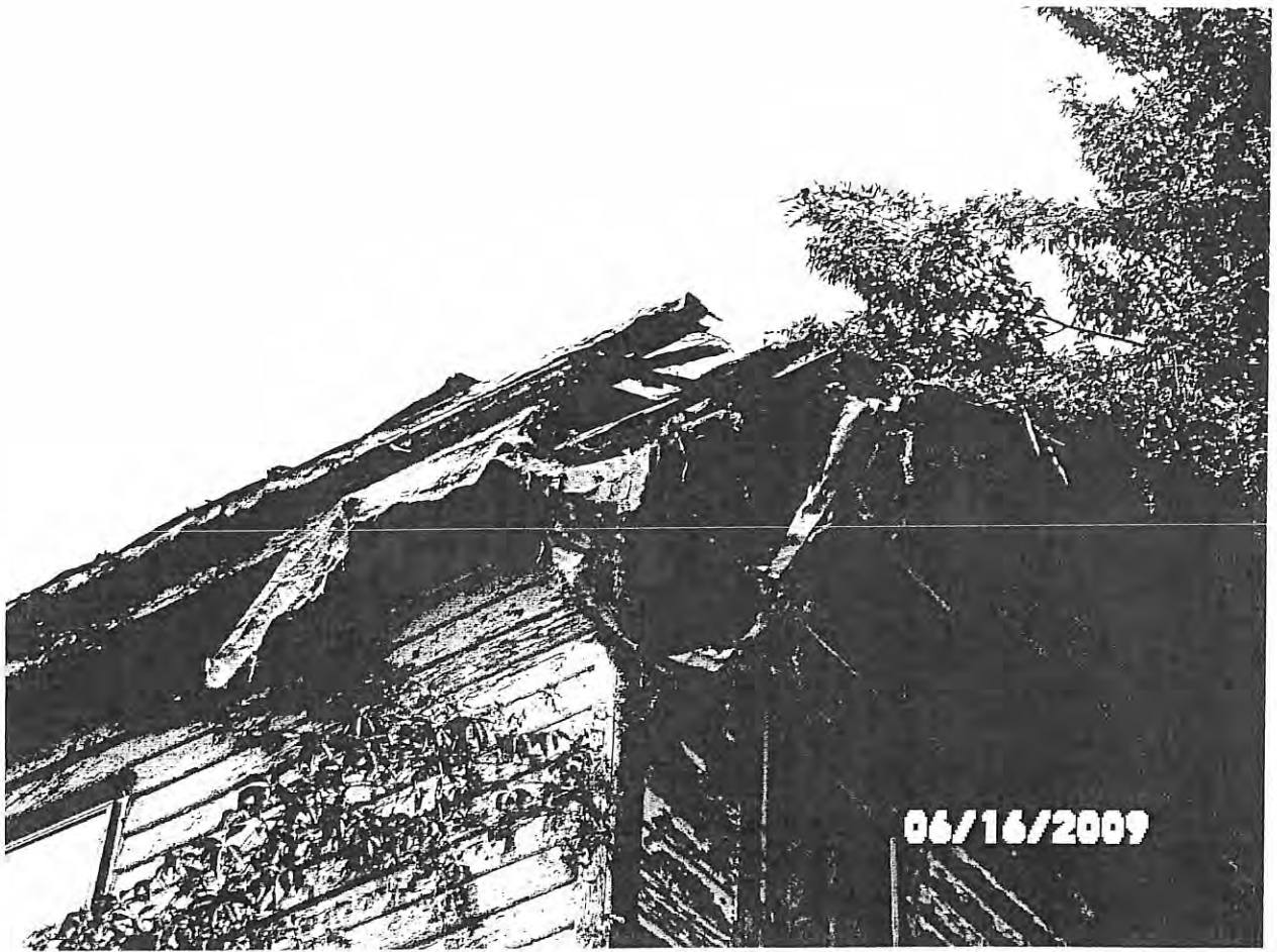
Left Front Corner at Roof
