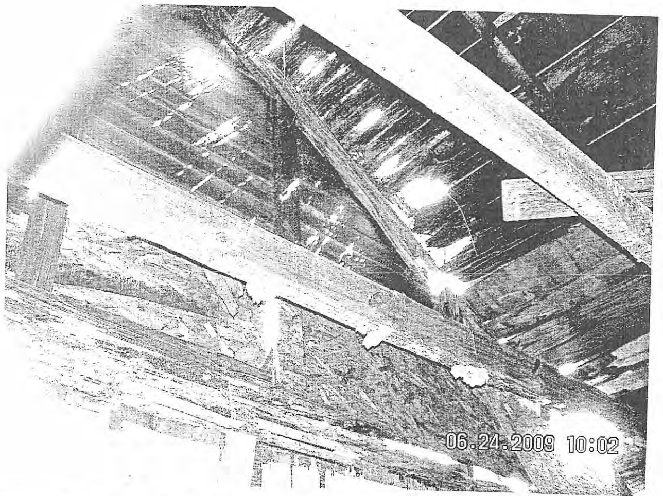
Front left corner of roof - note OSB where second floor porch roof was removed.
