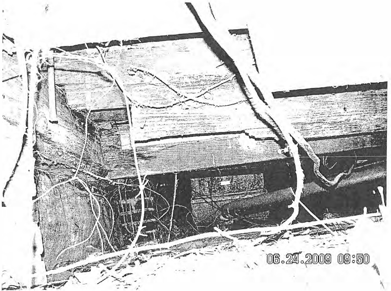
Floor under Kitchen
