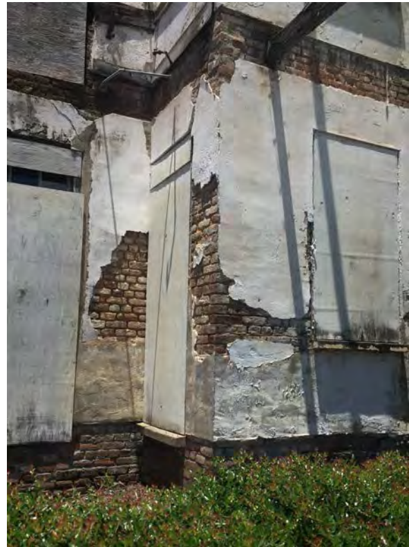
The house has a rear projection measuring approximately 12' deep by 15' long. This was likely an addition, although the brick bonding and composition is similar to the original building. The right hand image shows the addition's intersection with the block of the main house.
