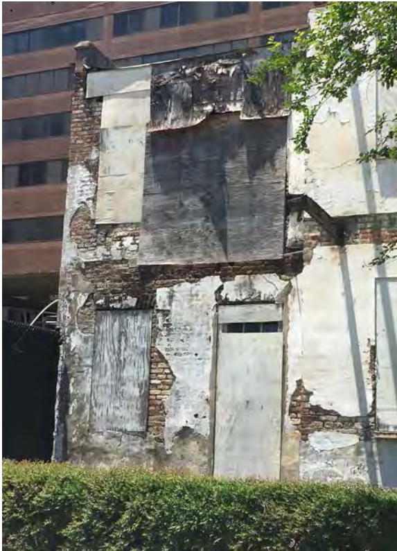
The house has a rear projection measuring approximately 12' deep by 15' long. This was likely an addition, although the brick bonding and composition is similar to the original building. The right hand image shows the addition's intersection with the block of the main house.
