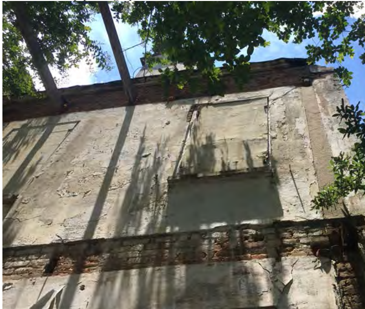
Floor joist pockets from a lost second story piazza and surviving piazza ceiling joists on the south façade.
