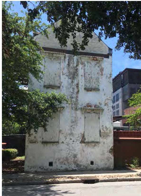
The eastern façade of 141 Ashley has dogtooth brickwork over the symmetrically spaced window openings. The gable end has fallen and the house' envelope is now enclosed with painted plywood.
