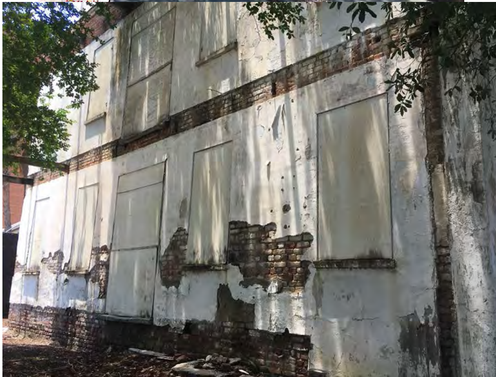
The south face of 141 Ashley, June 2017. The brick is exposed where stucco and the piazza framing have become detached, revealing an irregular bonding pattern of header and stretcher courses alternating, but not in an organized English (row of header and row of stretcher alternating in ABAB pattern) or American bond (several rows of stretchers, punctuated every third to sixth course with a line of headers.) The irregular bonding indicates that the house would have been stuccoed from the time of construction. Wooden window sills and door jambs survive. Remains of a set of masonry stairs leading the front door can also be seen.
