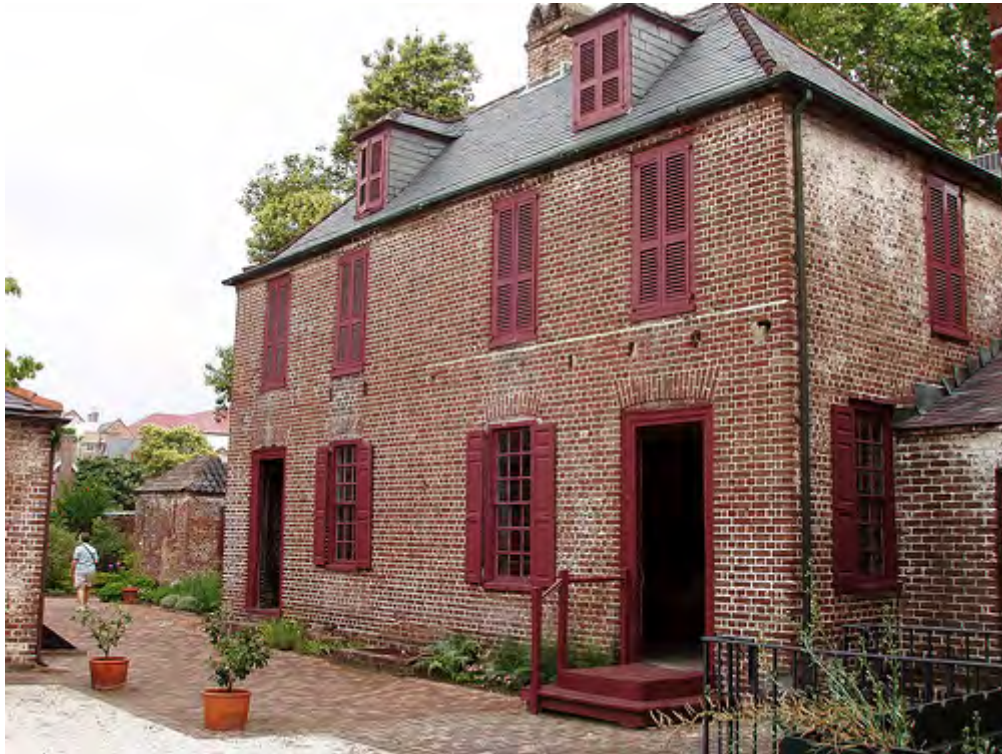
This outbuilding at the Heyward Washington House is divided into two bays or “units” by a large central chimney. The left section featured a laundry downstairs and dwelling space above, and the right bay was a kitchen downstairs and slave dwelling above. This attractive masonry building with operable shutters, dormers, and a slate roof is an excellent model for condo units.
