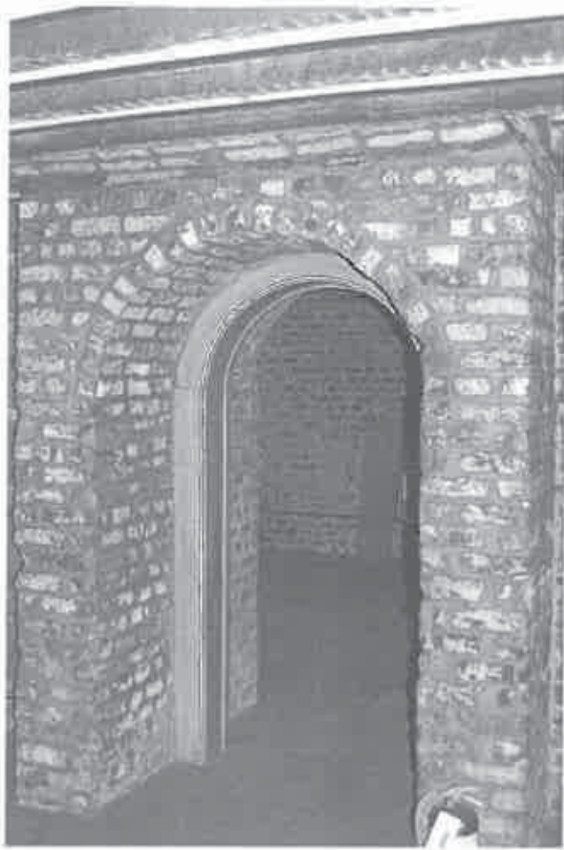
Vaulted chimney base, east stack. A doorway was cut through the chimney base as part of twentieth-century alterations.
