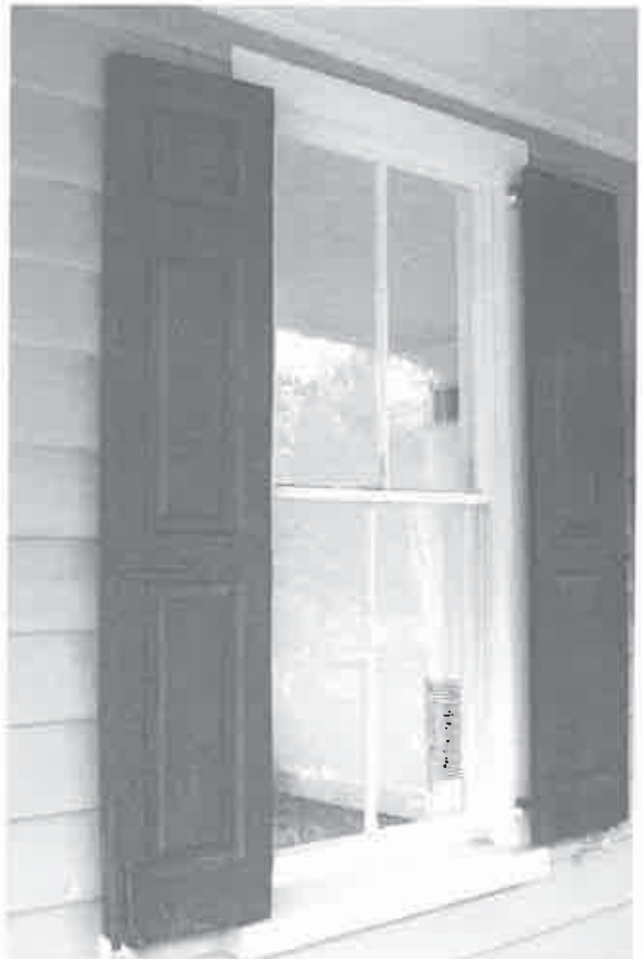
First-floor window, south facade. The jamb, shutter and hardware are original; the sash were replaced about 1870.
