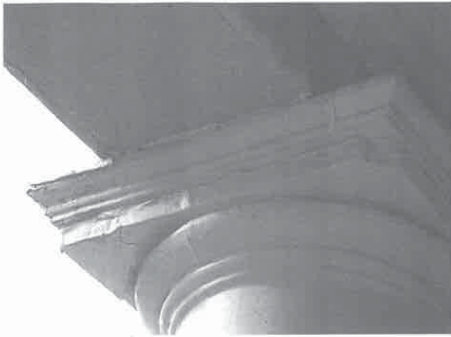
The original chamfered columns were replaced as part of the ca. 1827 work. The new turned columns were done in the Greek revival style, as can be seen here in the moldings of the capital.
