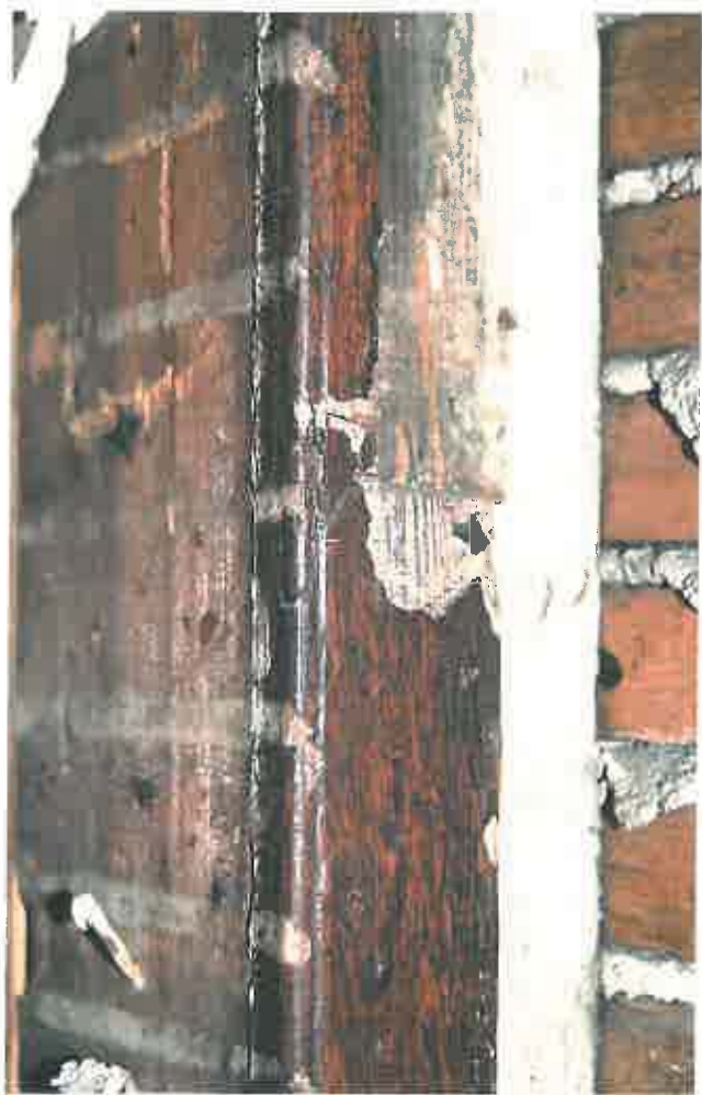
Detail of window trim that was encapsulated in the expanded stair hall, but was not blocked until changes in the 1870s. Circular-sawn lath seen to the right is evidence of the abandonment of this opening. Note the oak graining on the bead that represents a finish predating the 1870s alterations.
