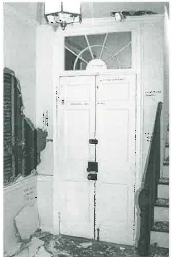
The stair hall was expanded to the south when the stair was moved to its present location in 1827.
