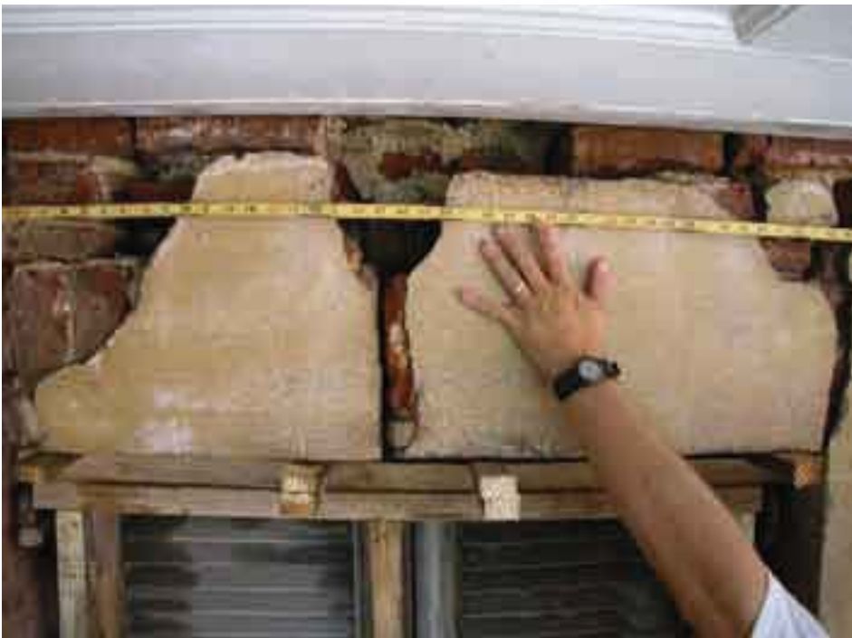
Hoyt Roberts of Richard Marks Restorations repairs a severely deteriorated "jack arch" at the Aiken-Rhett House. The process included removal of the large, intact sections, which were then replaced using a historically appropriate mortar mix. The area was then restuccoed and a yellow limewash applied to complete the restoration.
