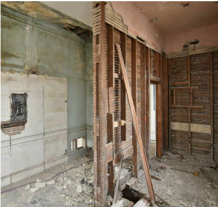
(Figure 16) Second Floor Lath. 2015.
