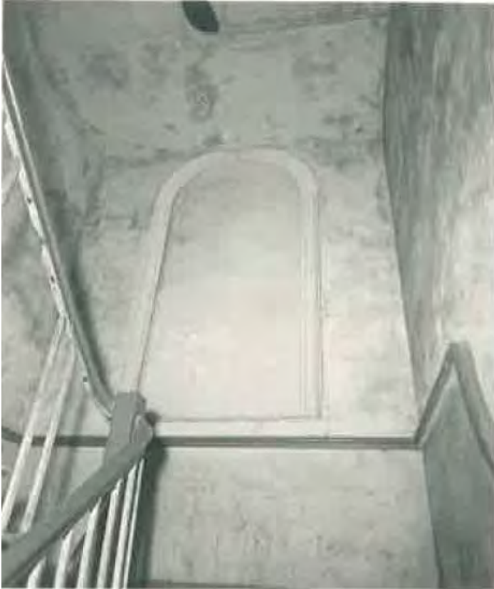
(Figure 13) Closed up/Sealed window from interior staircase. Circa 1950.
