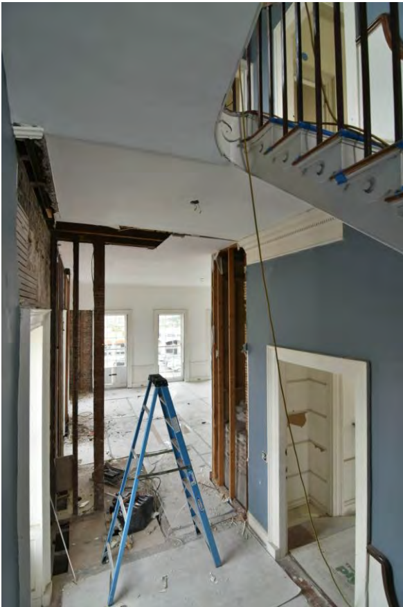
(Figure 32) Second Floor Wall , Opening up the Second Floor Plan. 2015.
