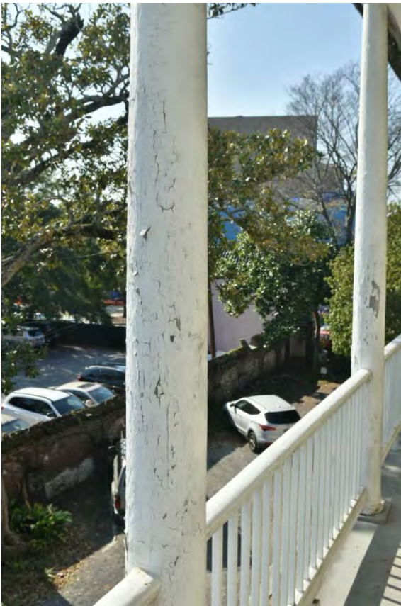
(Figure 34) Close up of wood Column with paint chipping. 2014
