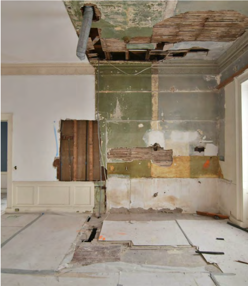
(Figure 15) First Floor, Front Room, showing lath and plaster during Luxury Simplified Restoration.
