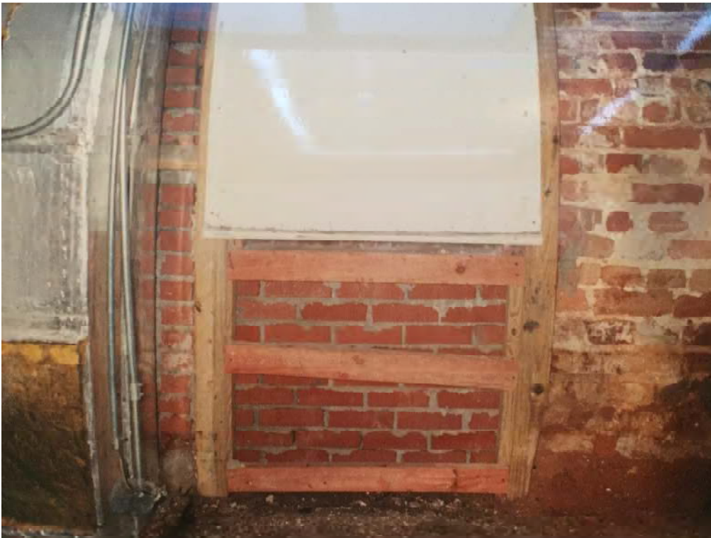
(Figure 17) "West wall, south window, showing that there was originally a doorway"
