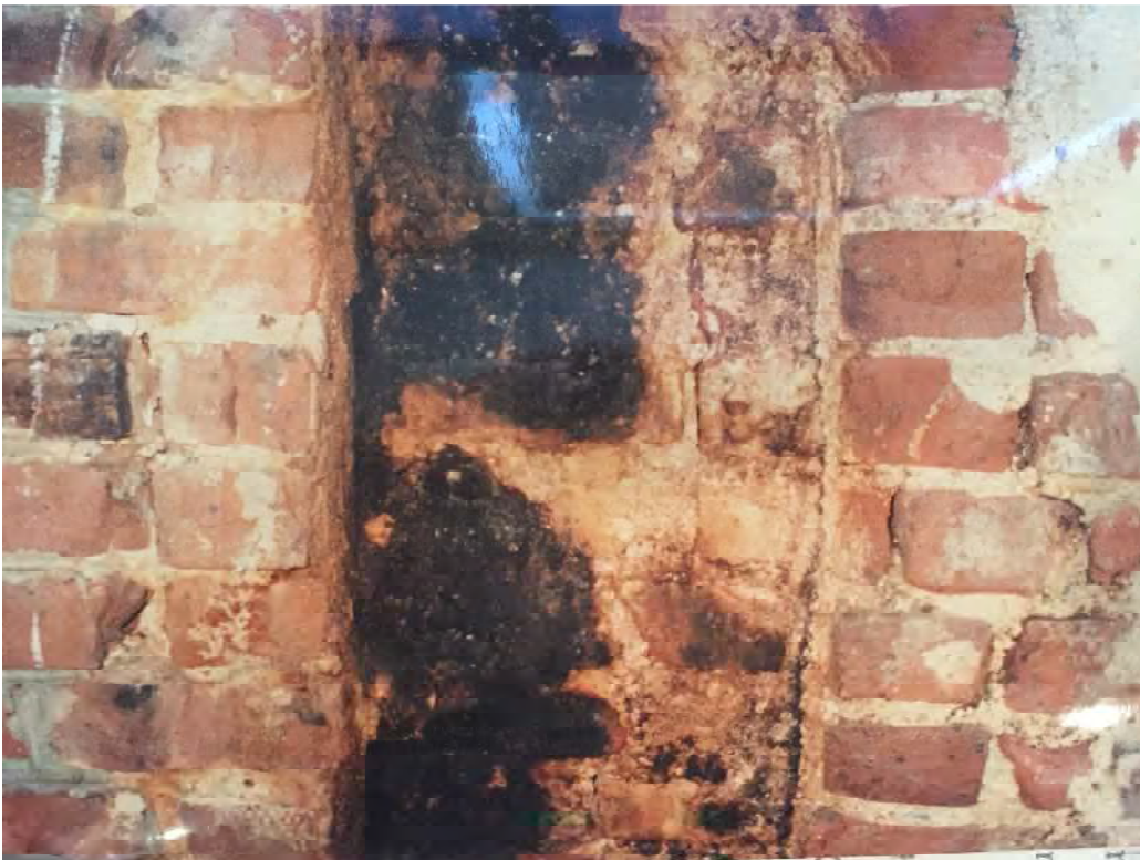
(Figure 14) "Upstairs chimney/east wall, note fire smoke stains"
