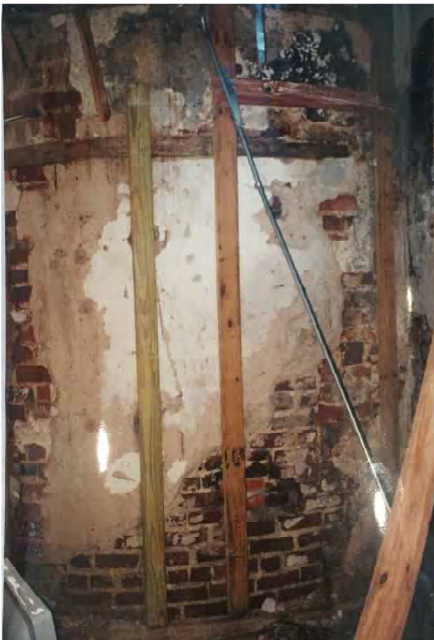
(Figure 16) “downstairs, west wall, north end, showing existence of earlier doorway”
