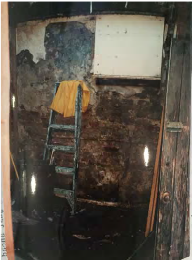
(Figure 20) "Downstairs, north wall, note window was originally much lower"
