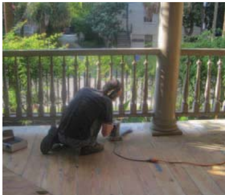
Wood rot was repaired to the first floor piazza decking.
