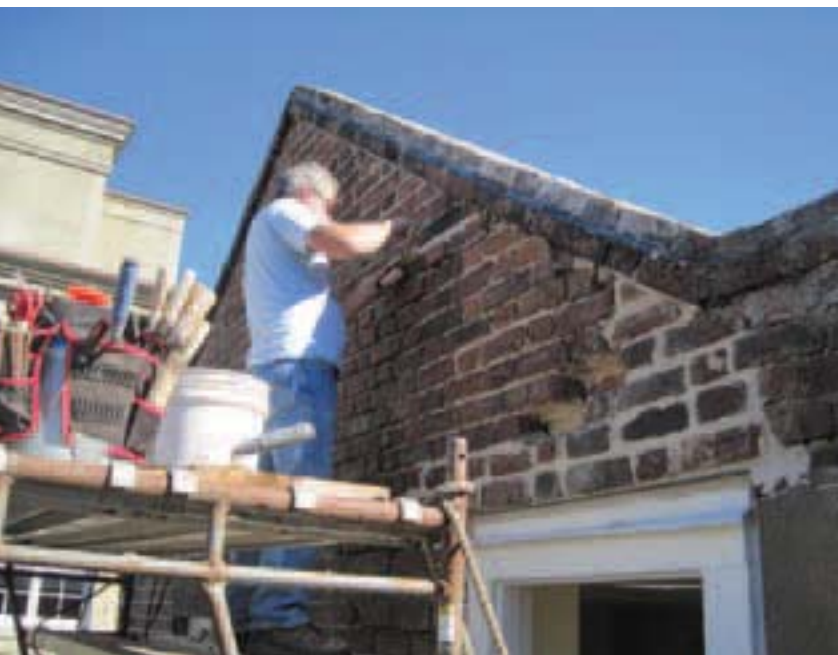
One of the projects at the Russell House was mortar repair to the rear elevation parapet wall.
