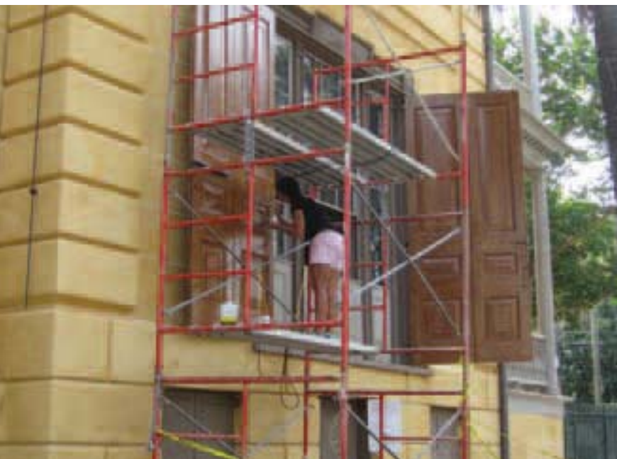
Repairs were made to the faux grained finish on the shutters along Elizabeth Street.
