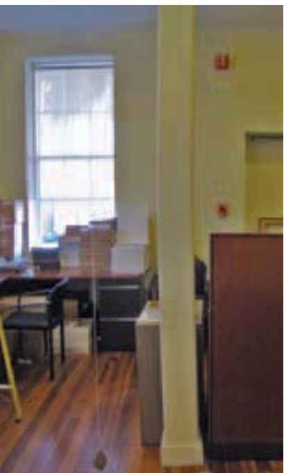
One of the many projects at the Missroon House was to stabilize warping structural columns.
