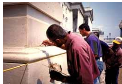
Masons practice using lime putty mortar to
