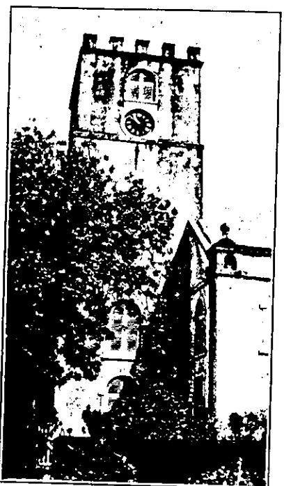
ST. PETER'S CHURCH, SPEIGHTSTOWN, BARBADOS. FRONT VIEW
