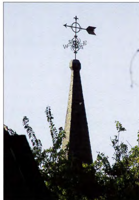
The AME steeple features an inner core of steel.
