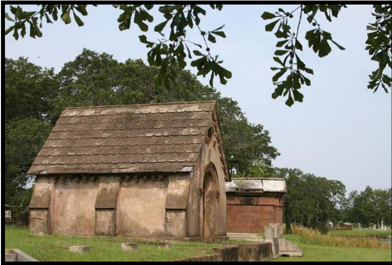
Lowcountry has no native stone, Brownstone became a popular building material in the mid 19<sup>th</sup> century. The inherent weaknesses in the stone which causes it to delaminate when exposed to the elements, contributed to its decline as a building material.
