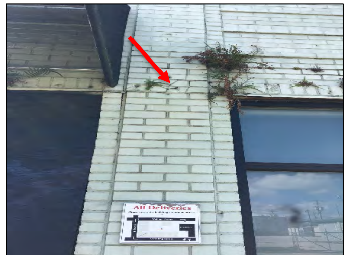
Photo 36: Cracks in brick façade at east elevation
