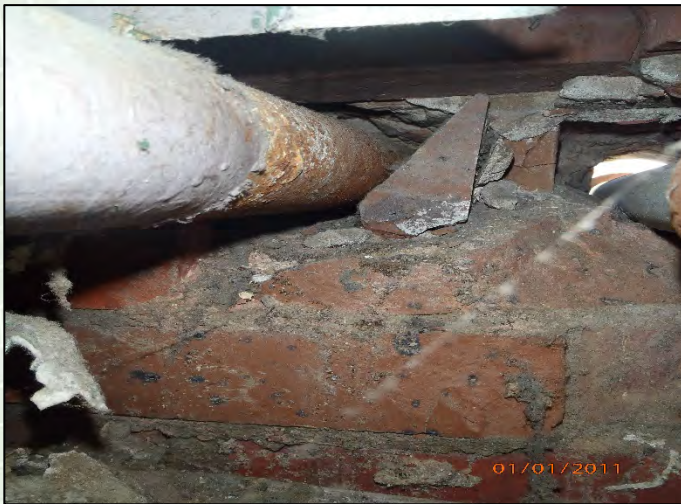
Photo 33: Pipe penetration through CMU at lintel bearing above
