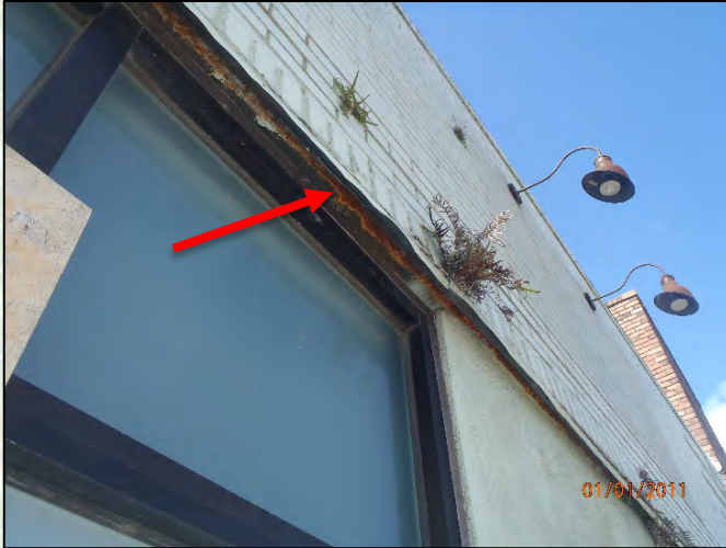
Photo 37: Corrosion of steel lintel at east wall
