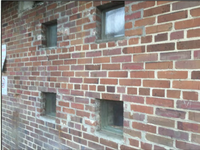
Photo 3: Glass block window infill to south wall
