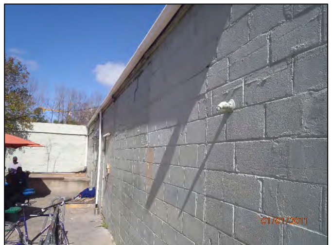
Photo 24: East wall of addition with visible cracking
