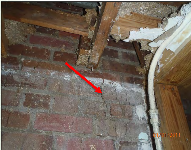
Photo 35: Crack in brick façade at east elevation
