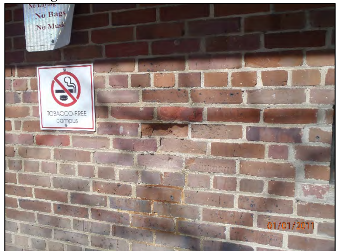
Photo 14: Broken brick in façade
