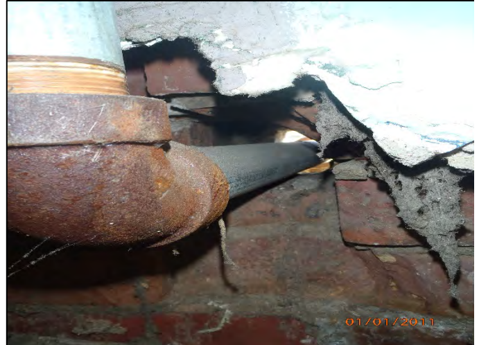
Photo 32: Close up view of penetration at east CMU wall bearing point
