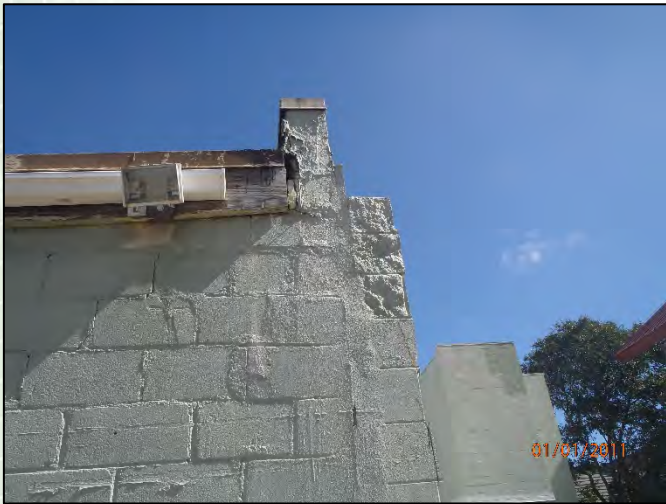
Photo 49: Visible crack in CMU west wall
