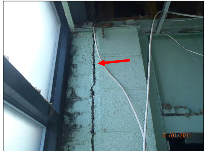
Photo 28: Displaced brick at west façade at roof
