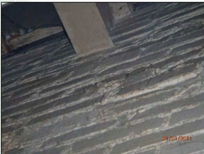
Photo 7: Steel beam bearing in beam pocket at north wall
