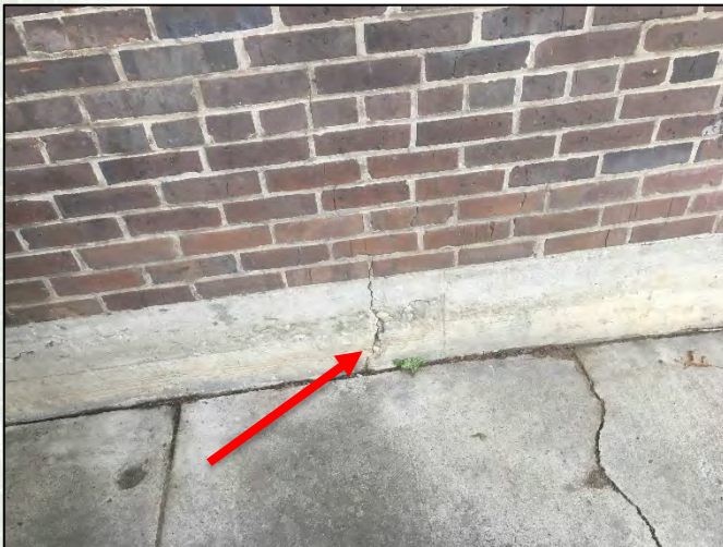
Photo 45: Visible crack in foundation wall
