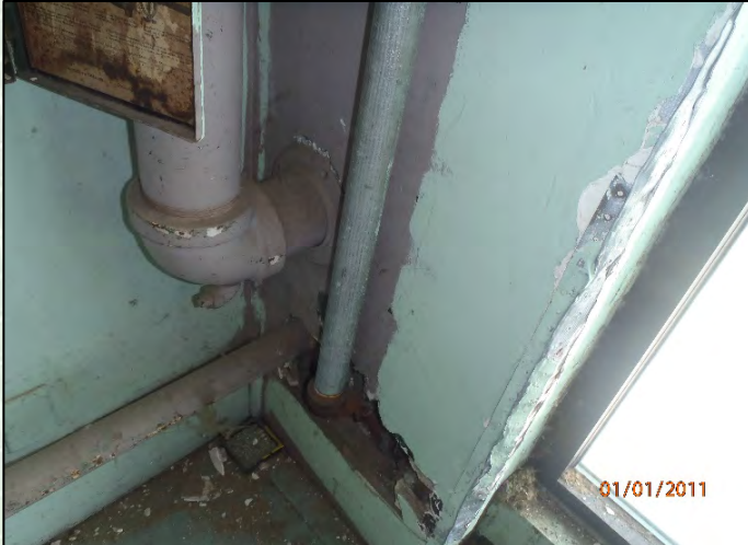
Photo 31: Penetrations at CMU bearing point in East wall
