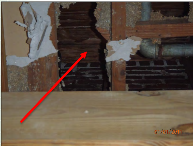
Photo 41: Water intrusion damage near east wall
