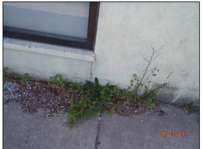
Photo 40: Cracks in stucco veneer near East wall foundation
