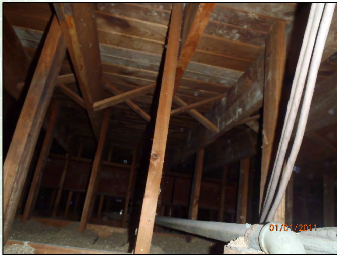
Photo 5: Typical roof framing at original building
