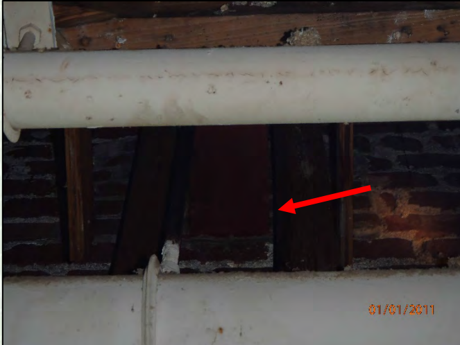
Photo 25: Steel beam bearing on shared north wall
