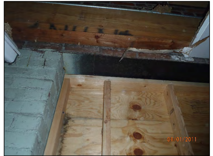
Photo 34: Water intrusion damage at East face wall
