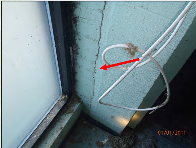
Photo 27: Displaced brick at west façade at foundation
