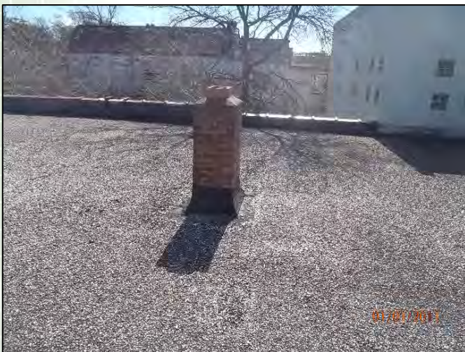
Photo 13: Typical view of modified bituminous roof at original building
