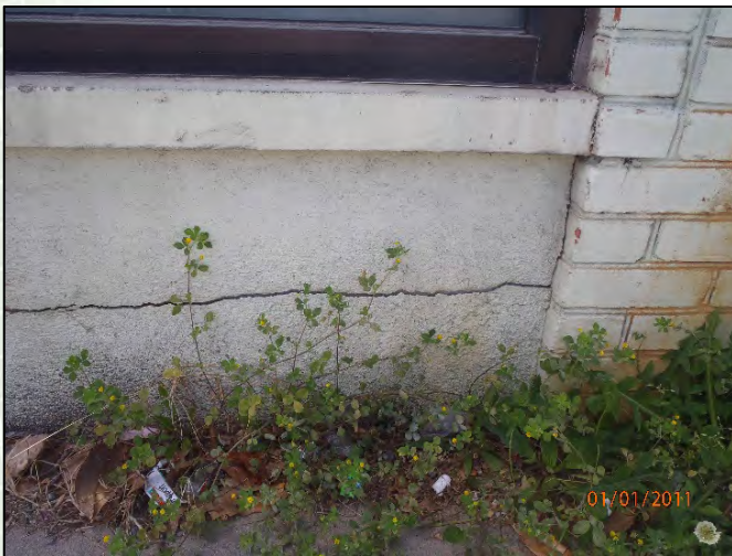
Photo 39: Cracks in stucco veneer at east wall
