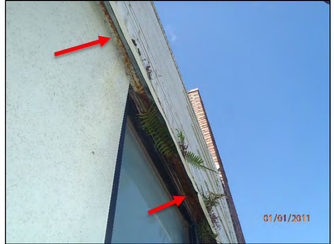
Photo 38: Corrosion of steel lintel at east wall
