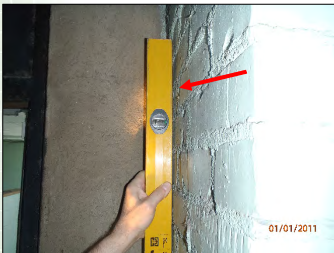
Photo 29: East wall out of plumb
