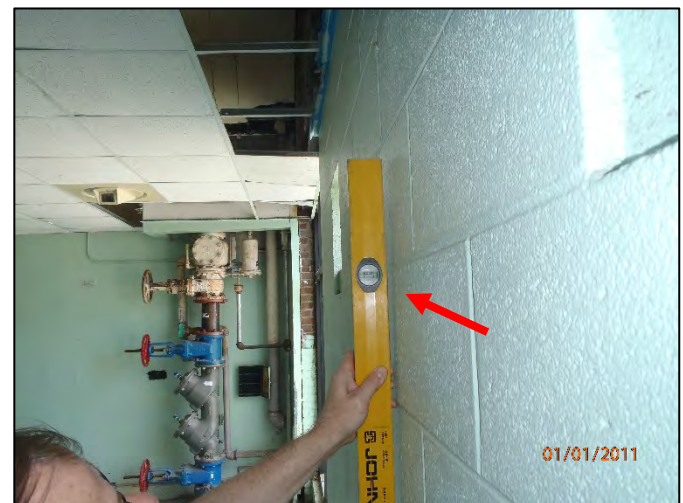
Photo 30: East wall out of plumb
