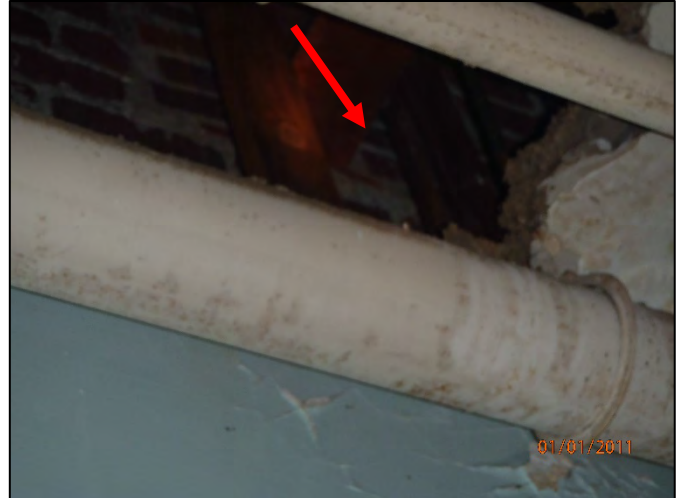
Photo 26: Steel beam bearing on shared north wall
