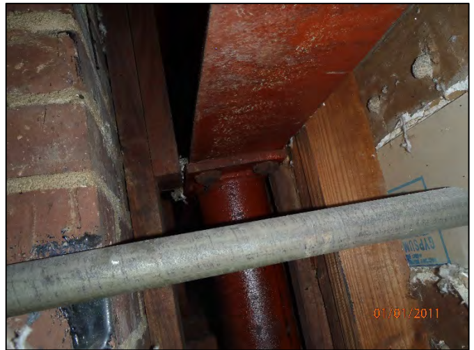
Photo 6: Steel column and beam that support roof
