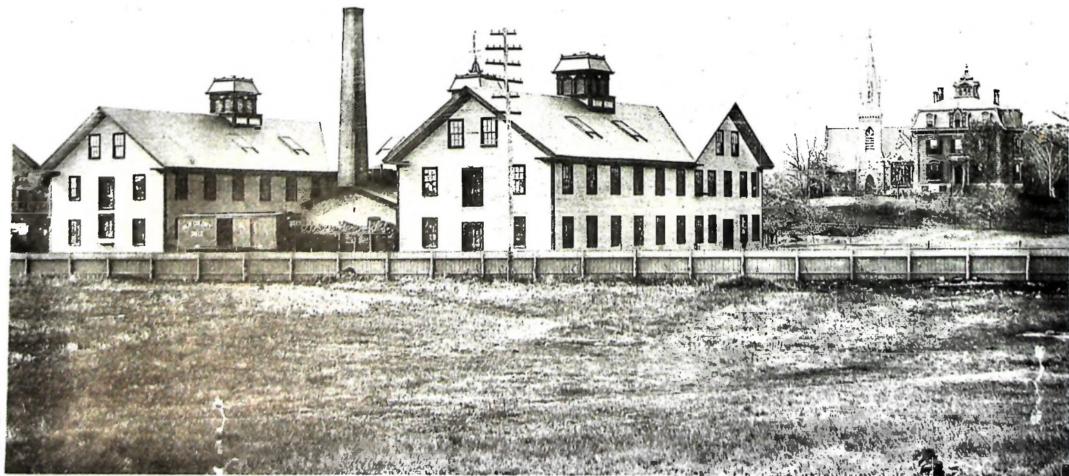
W. GILMORE'S HINGE FACTORY AND HOUSE, NORTH EASTON.
