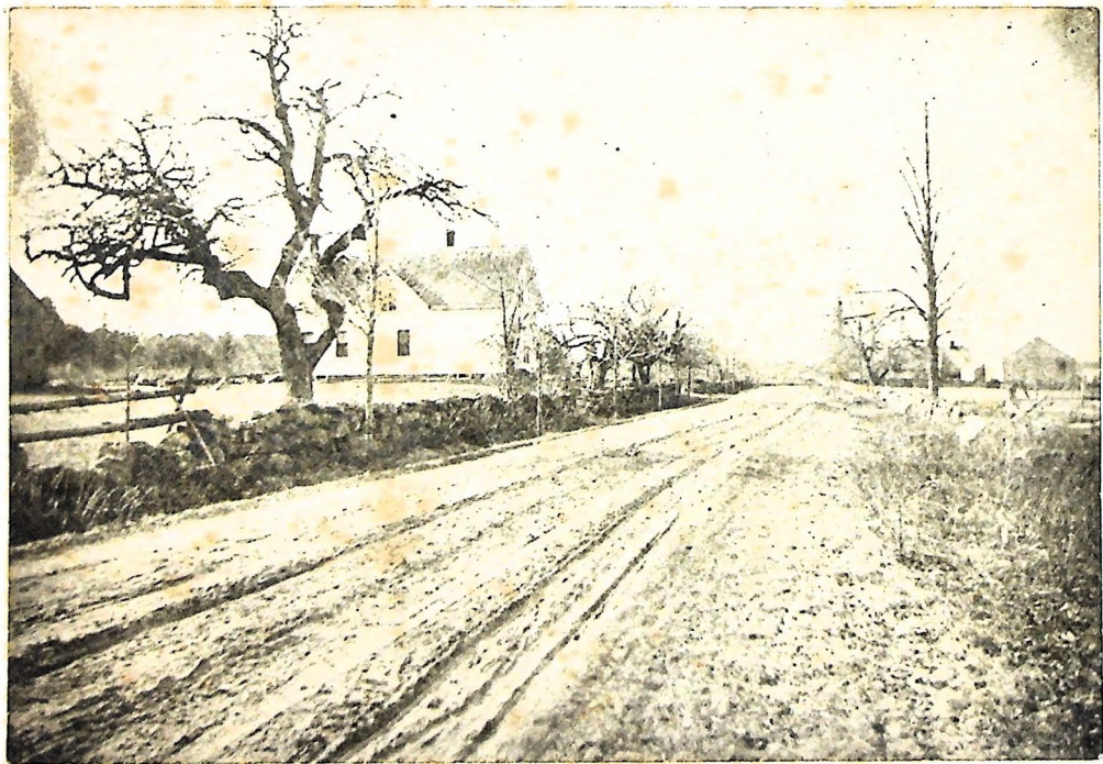
BAY RD - SOUTH TOWARDS NORTON 1895 GEORGE WILLIAMS HOUSE ON LEFT
