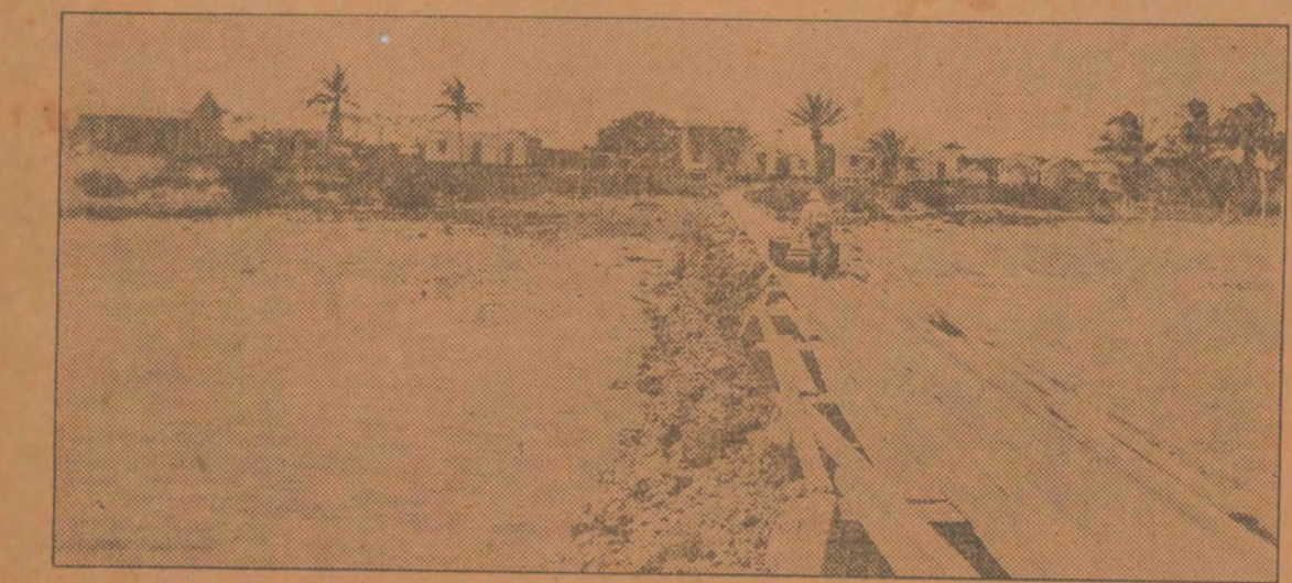
PLANTER AS SEEN FROM THE OCEAN IN 1905—In the days before the railroad, supplies for Key Largo were brought by boat to Planter, then the main settlement on the island. Tenders of the ocean-going ships brought Key Largo-bound passengers and freight to the dock shown in the picture, and the freight was transported to Johnson's store over the wooden trestle, also shown above.
