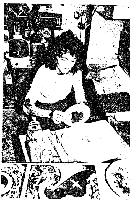
Porcelain fused into copper at 1800° degrees
