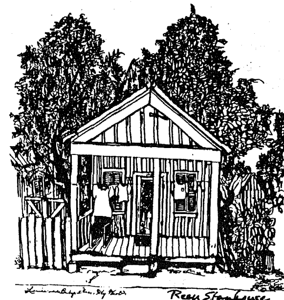
This drawing depicts a typical board and batten structure that housed cigarmakers in days gone by.
