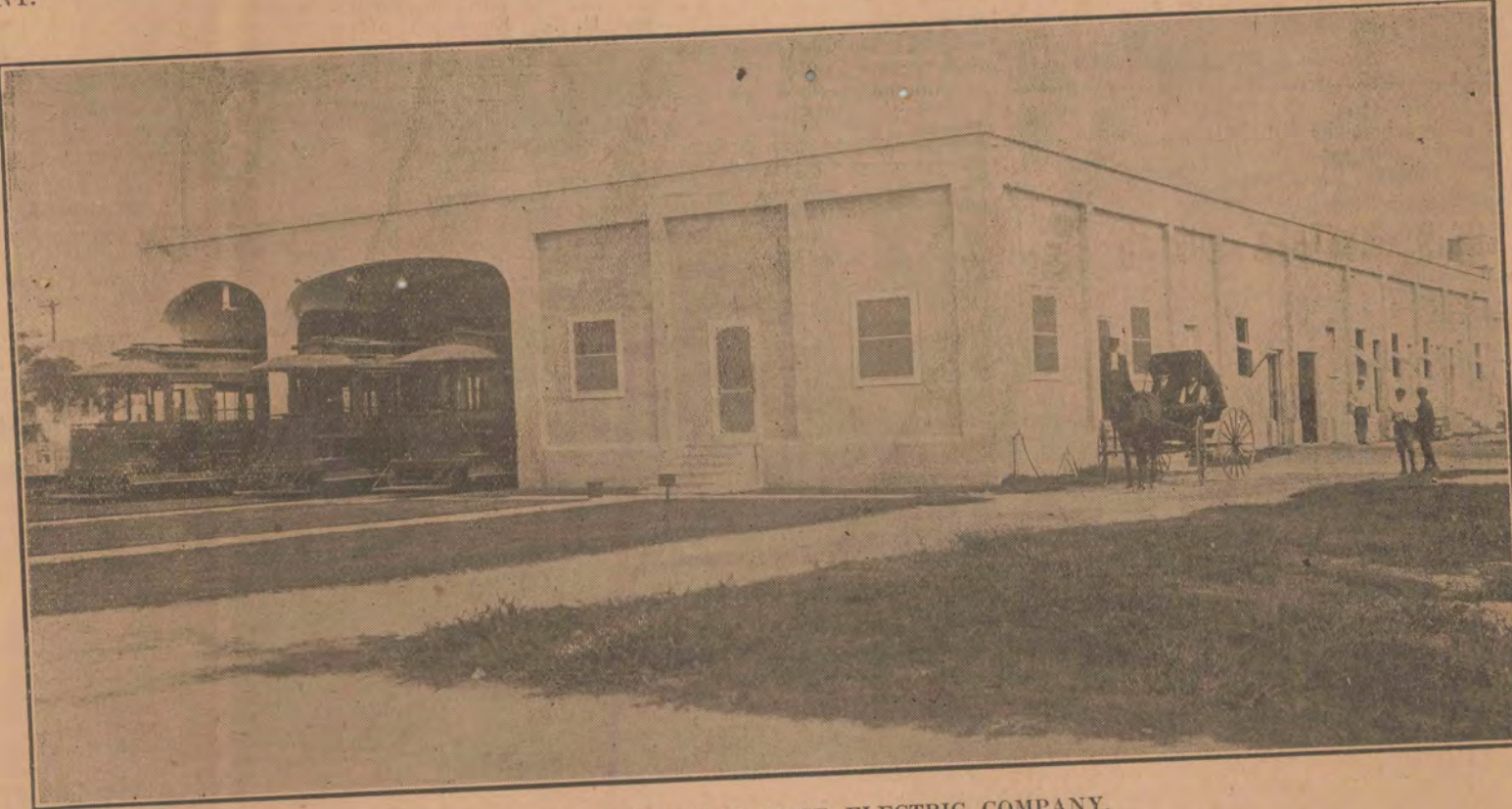
CAR BARN OF THE KEY WEST ELECTRIC COMPANY.
