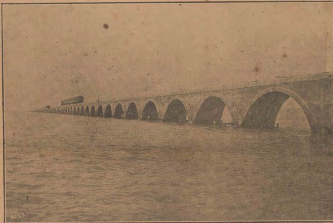
THE FAMOUS LONG KEY VIADUCT--A TRIUMPH OF RAILWAY CONSTRUCTION.
