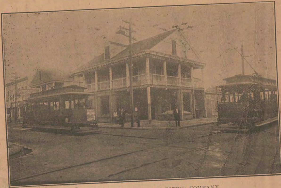
OFFICE OF THE KEY WEST ELECTRIC COMPANY.
